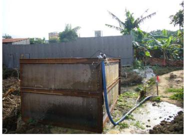
Plastic tube connected to the sedimentation tank was broken; Contractor was reminded to repair immediately.
