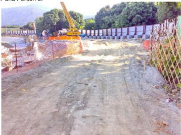
Fugitive dusts emission from the dry haul road was observed at CH080-150. The Contractor was reminded to provide water spray more frequency on the dry and windy season.
