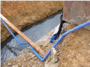
Discharge water from the sedimentation tank directly hit on the exposed surface, the Contractor was reminded to provide the tarpaulin sheet to protect the exposed surface to prevent the any soil runoff from the discharge water into the stream.
