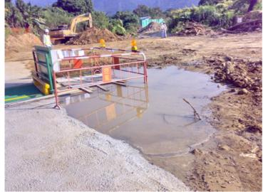
Stagnant water accumulated on-site next to the wheel washing bay was observed. The Contractor was reminded to clean up in regular basis.
