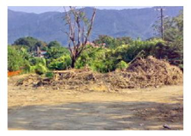
Some C&D wastes accumulated on-site was found at CH 015-020. The Contractor was reminded to clean up and disposal the C&D wastes in regular basis.
