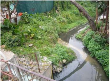
Wheel washing wastewater directly discharge into the stream was observed at CH459, the Contractor was reminded to divert all the wastewater to the desliting facility prior to discharge.
