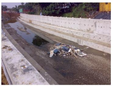
Debris and C&D wastes accumulated on site was observed at CH160. The Contractor was reminded to clean up in regular basis.
