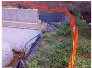
Wastewater directly discharge without diverted to the sedimentation tank was observed at CH500. The Contractor was reminded to provide sedimentation tank accordingly.
