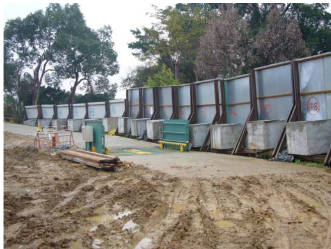
C&D waste at CH 080 was cleaned and tight up
