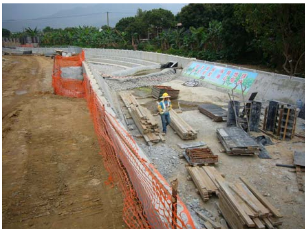
Working area at Bay 23 was tight up.
