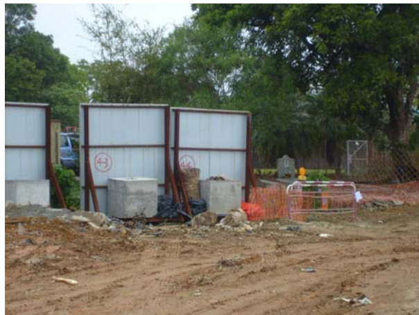
C&D waste at the CH200 was cleared.
