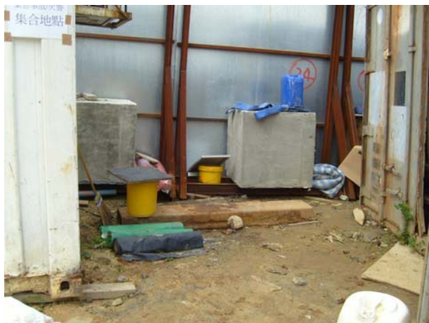
Working area at CH320 was tight up.
