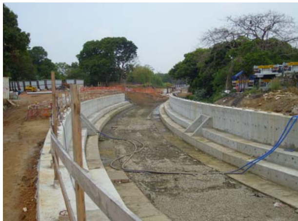
Stagnant water CH 200 was cleared.
