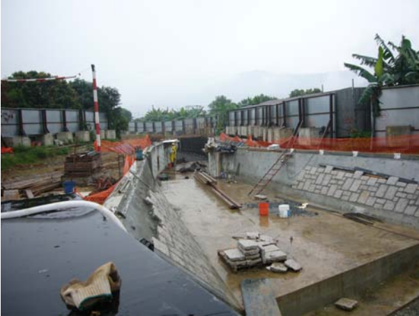
C & D material at CH680 was cleared.
