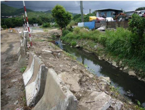
1. General and C&D waste was cleared.
