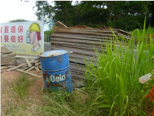
3. Un-used water collection drum was observed at Bay 41, the contractor was reminded to cover the drum to prevent any stagnant water accumulation.
