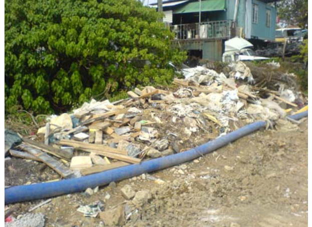
C&D waste accumulated on-site was observed at CH340, the Contractor was reminded to tidy up the C&D wastes and dispose off in regular basis.
