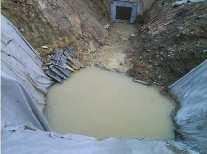
Stagnant water was observed (Ch.20), the contractor shall pump the water out to prevent mosquito breeding especially in wet season.
