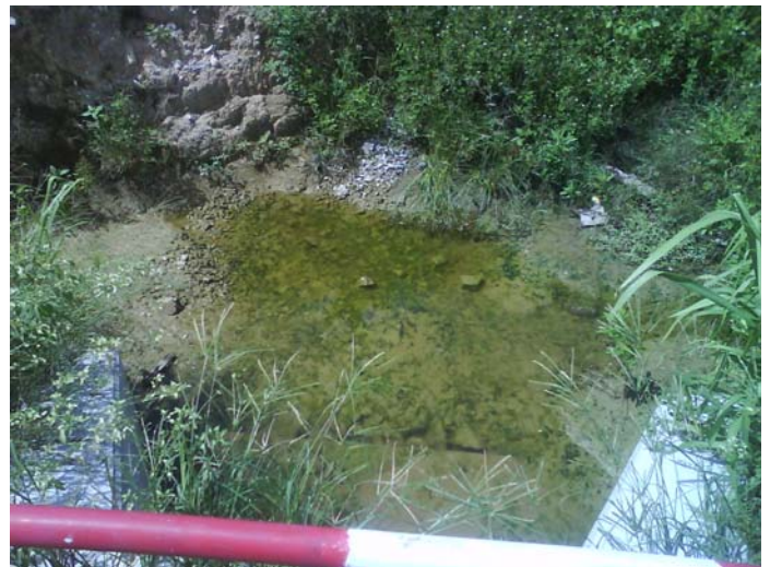
Remark 2: Stagnant water was observed at Ch. 1516, the Contractor shall drain the water away or apply larvicidal oil to prevent mosquitoes breeding.
