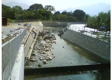
Remark 1: The Contractor is reminded to place the sand bag or bund to isolate the construction area (bay 1) from the existing stream in order to minimize the water quality impact.
