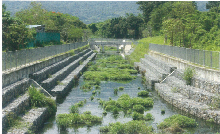
Existing condition of KT15
