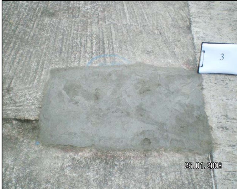
Repaired cracked / damaged concrete ground slab outside Refrigeration Block in Kennedy Town Abattoir
