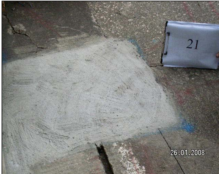
Repaired cracked / damaged concrete ground slab outside Lairage Block and the steel shed in Kennedy Town Abattoir
