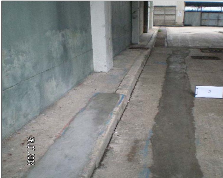
Repaired cracked / damaged concrete road slab between Refrigeration Block and Slaughterhouse Block in Kennedy Town Abattoir
