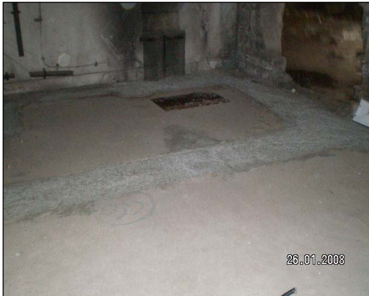
Repaired cracked / broken concrete ground slab inside the Kennedy Town Incineration Plant
