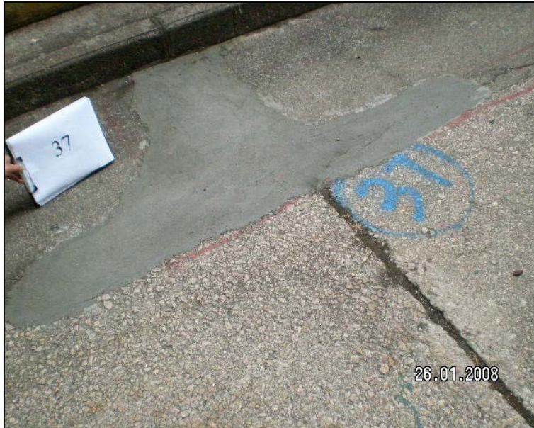
Repaired cracked / damaged road slab between the external wall and Lairage Block in Kennedy Town Abattoir
