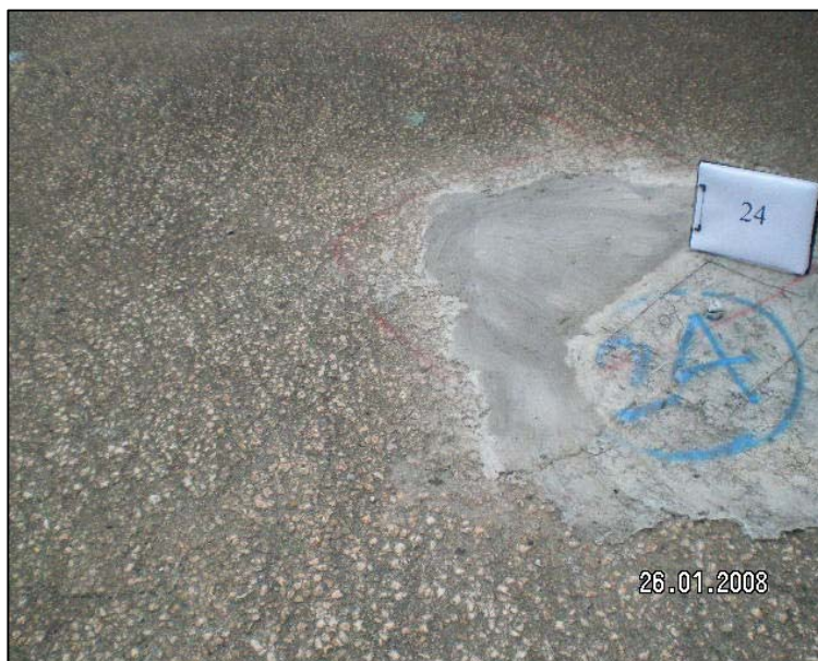
Repaired cracked / damaged road slab between Chimney B and the ramp in Kennedy Town Incineration Plant
