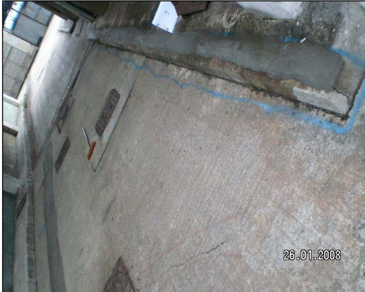
Repaired cracked / damaged concrete road kerb between Refrigeration Block and Slaughterhouse Block in Kennedy Town Abattoir
