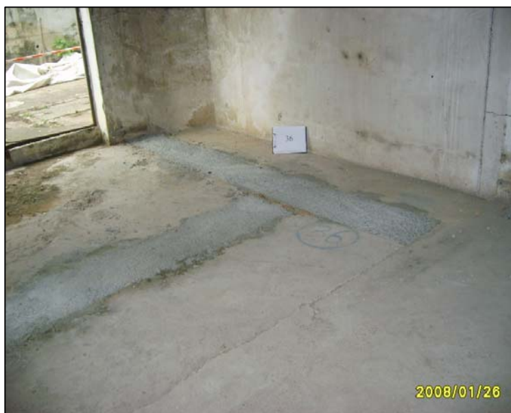
Repaired cracked / broken concrete ground slab inside the Kennedy Town Incineration Plant
