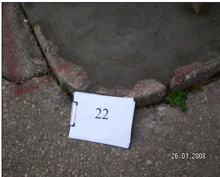
Repaired cracked / damaged concrete ground slab and kerb outside Lairage Block in Kennedy Town Abattoir
