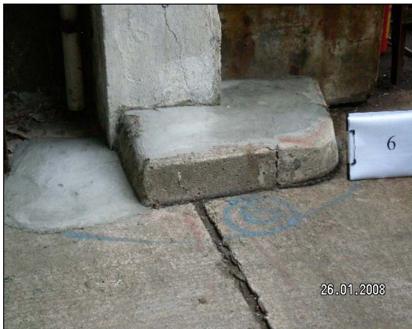
Repaired cracked / damaged concrete road kerb and slab between Refrigeration Block and Slaughterhouse Block in Kennedy Town Abattoir
