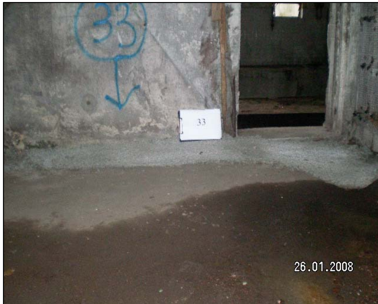
Repaired cracked / damaged concrete ground slab inside the Kennedy Town Incineration Plant
