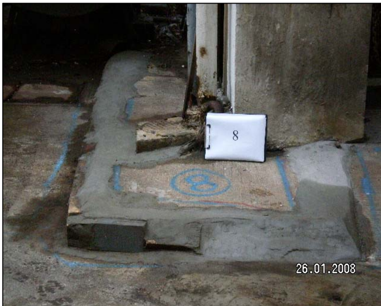
Repaired cracked / damaged concrete ground slab between E&M Services Dept. and Chimney C in Kennedy Town Abattoir
