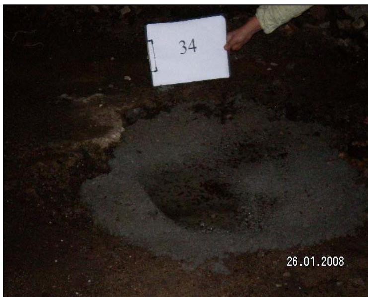
Repaired cracked / damaged concrete ground slab inside the Kennedy Town Incineration Plant
