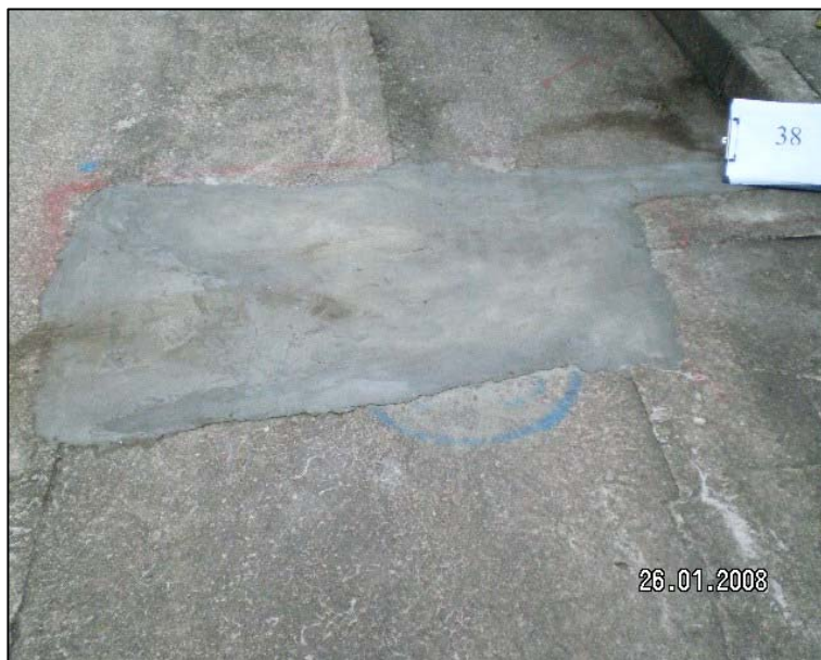
Repaired cracked / damaged road slab between the external wall and Lairage Block in Kennedy Town Abattoir
