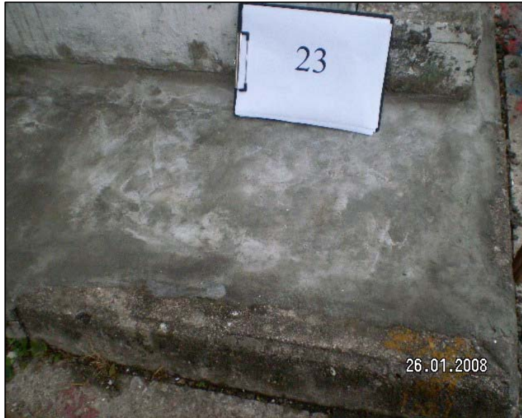
Repaired cracked / damaged concrete ground slab and kerb outside Lairage Block and the ramp in Kennedy Town Abattoir
