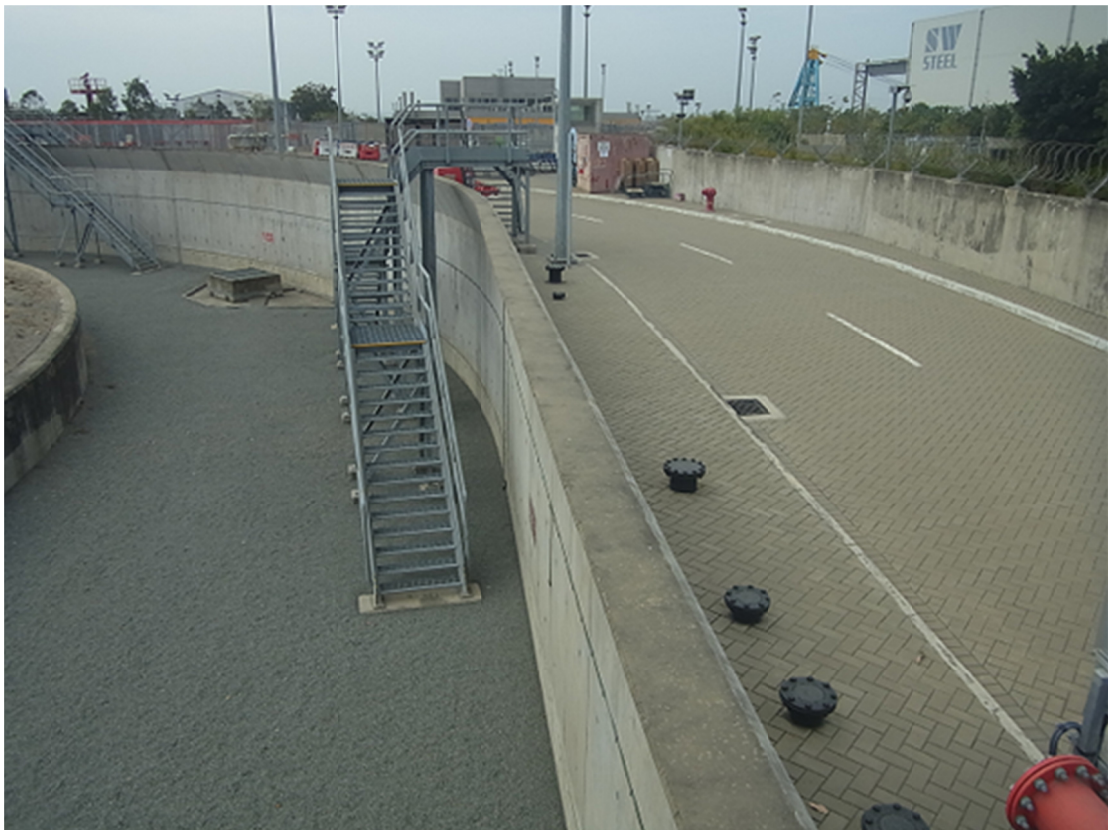
(2) Phase 1a bunded compound is partly sunken below the level of ground outside the bunds
