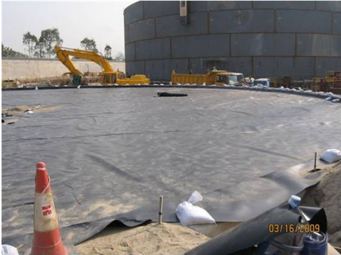
(21) Record photo shows impervious membrane being installed on top of tank foundation
