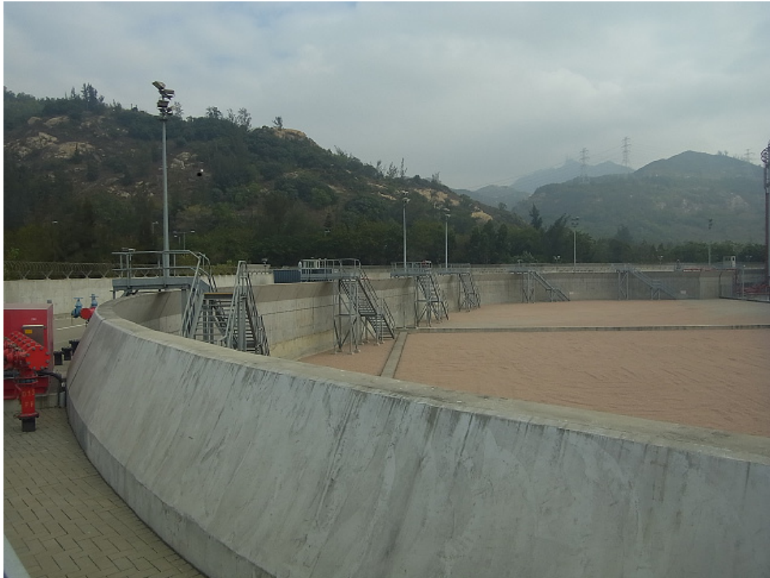
(3) Phase 1b bunded compound is partly sunken below the level of ground outside the bunds
