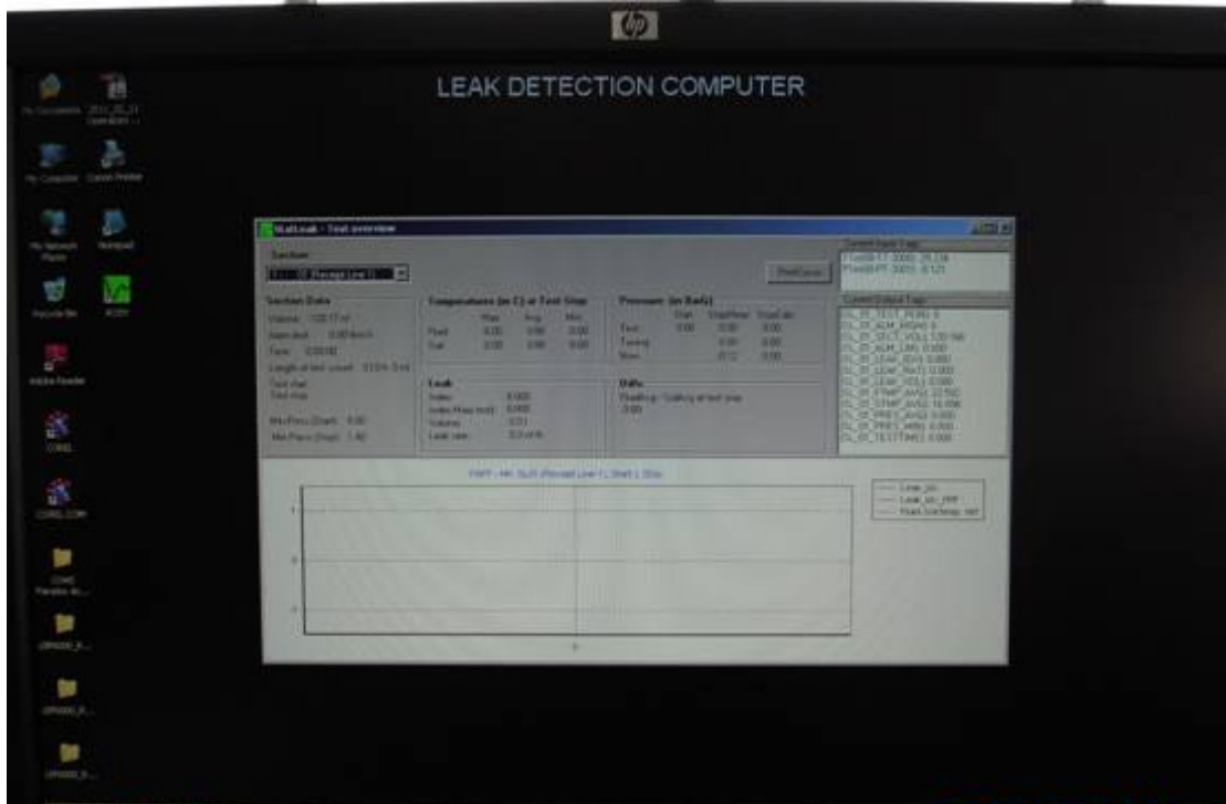
(26) Leak detection “COWI Stat Leak System” installed into computer
