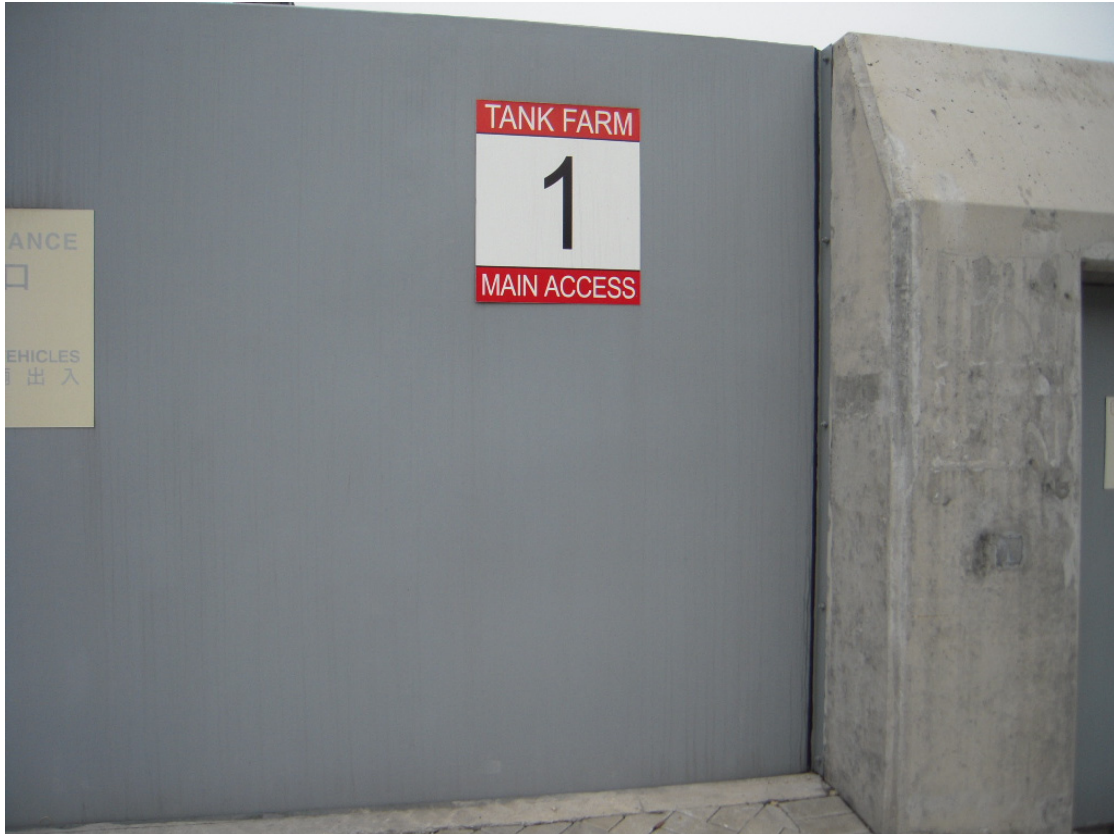
(13) Gates at security walls with sealant are maintained in good condition
