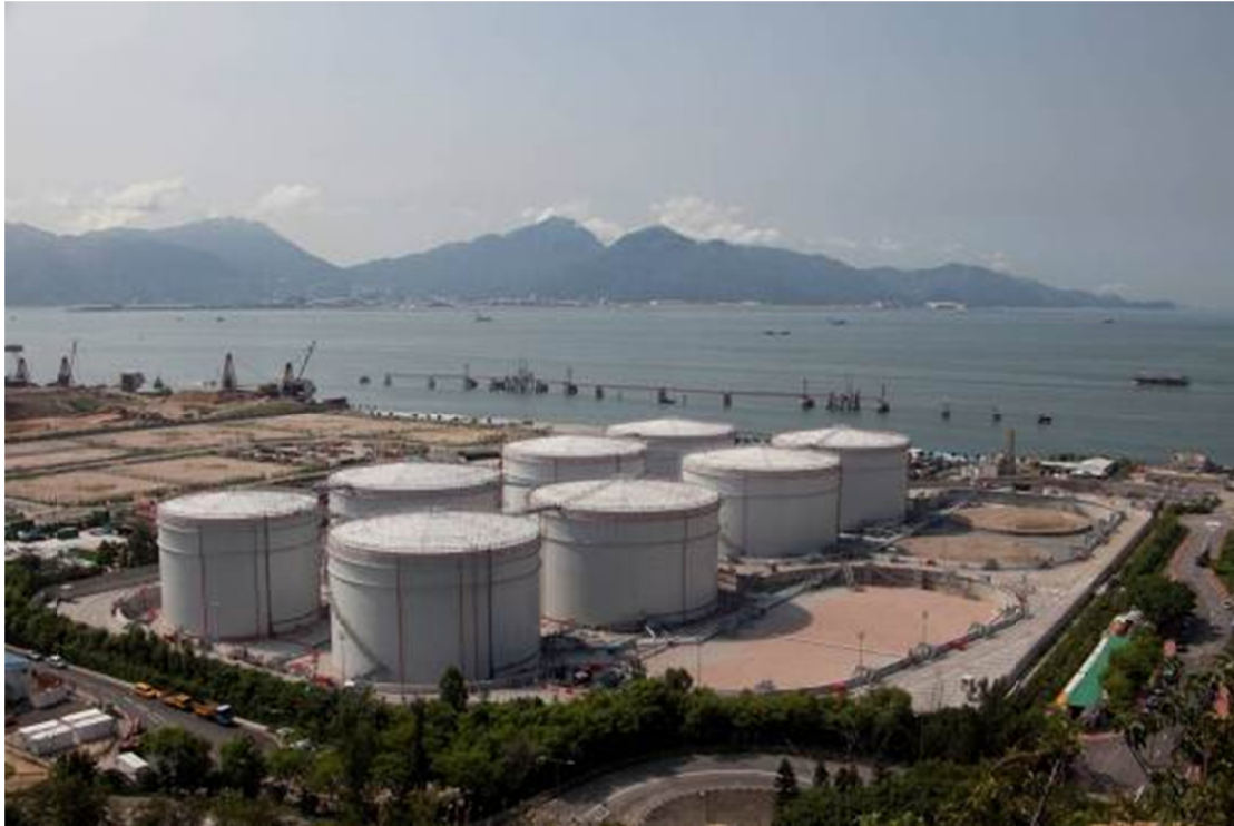
(1) All eight tanks are located within bunded compounds
