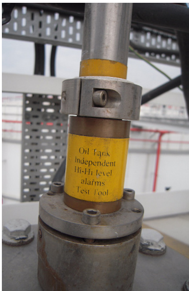
(24) Regular inspection performed on overfilling monitoring device ( HH Level Alarm)
