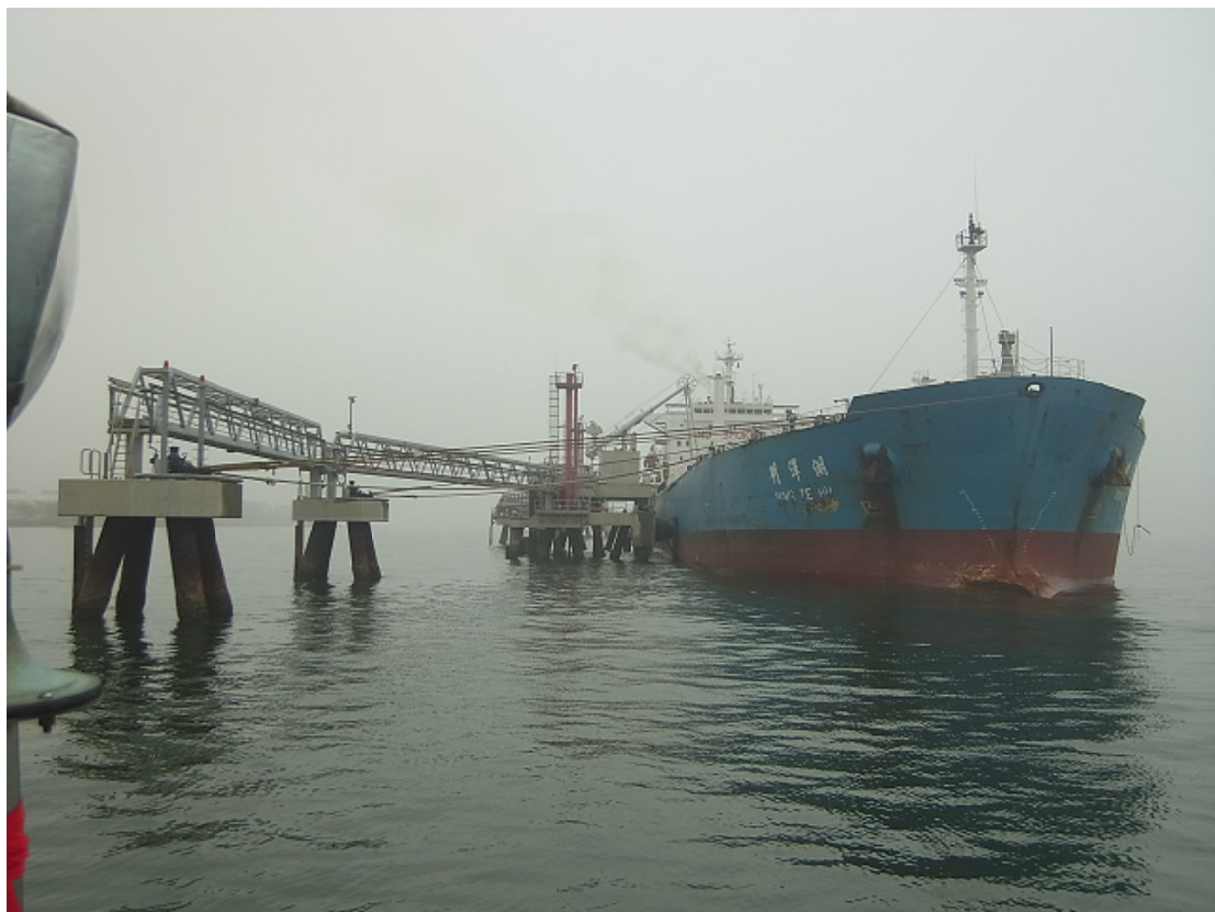
(35) Fenders installed at sea side of the jetty
