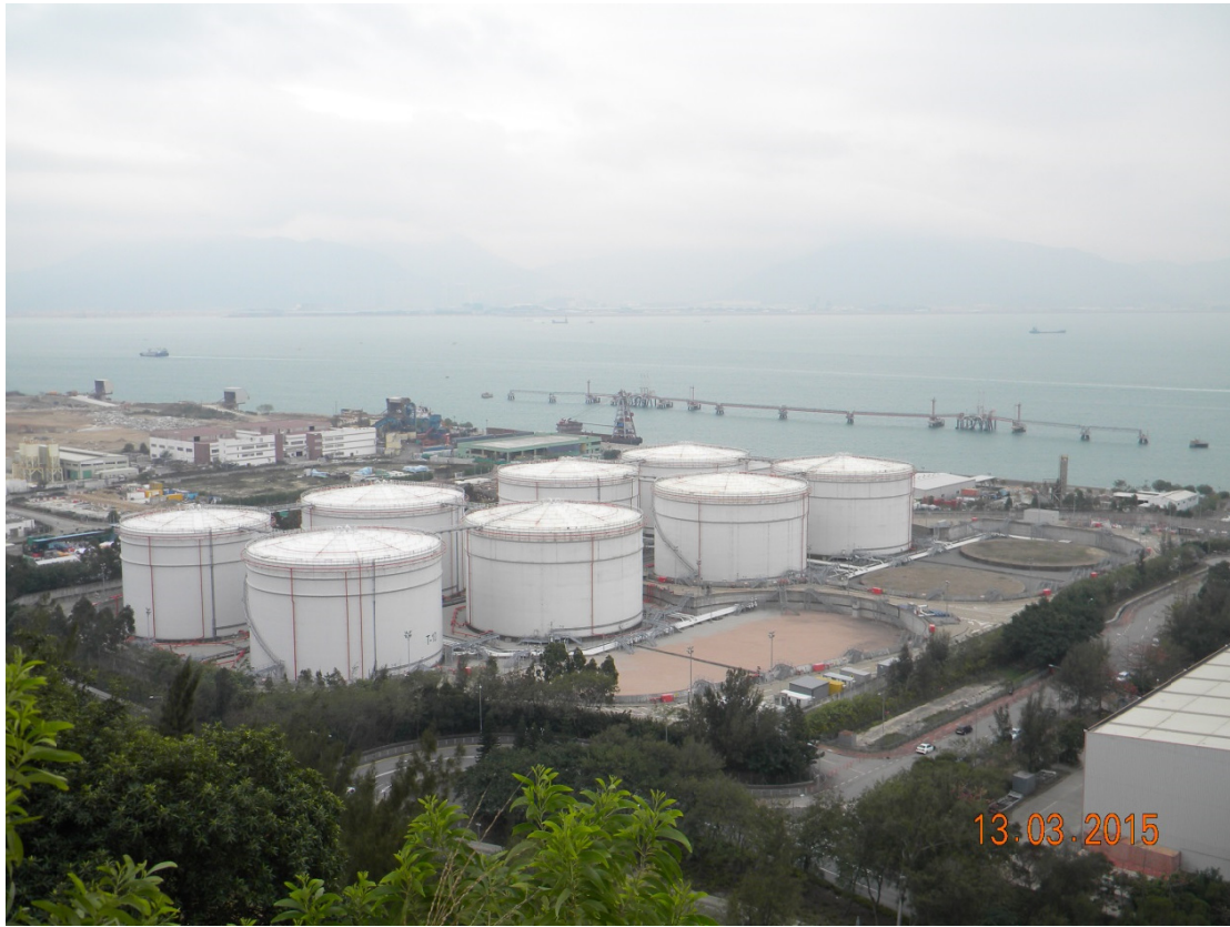
(1) All eight tanks are located within bunded compounds
