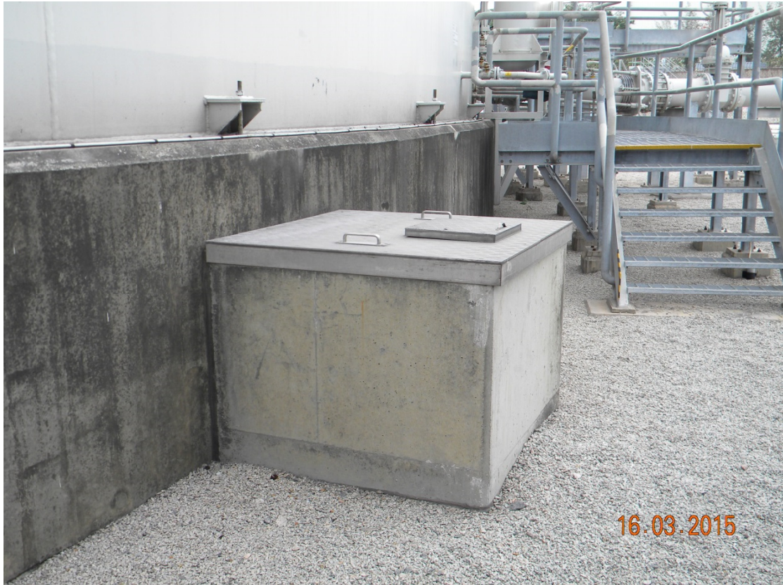
(28) Collection chamber located adjacent to tank foundation is maintained in good condition with periodic inspection
