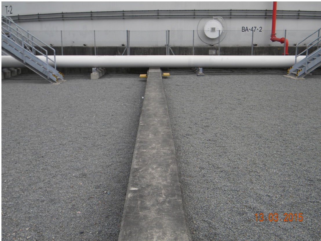
(8) Intermediate bund walls are provided in place near T-01-002
