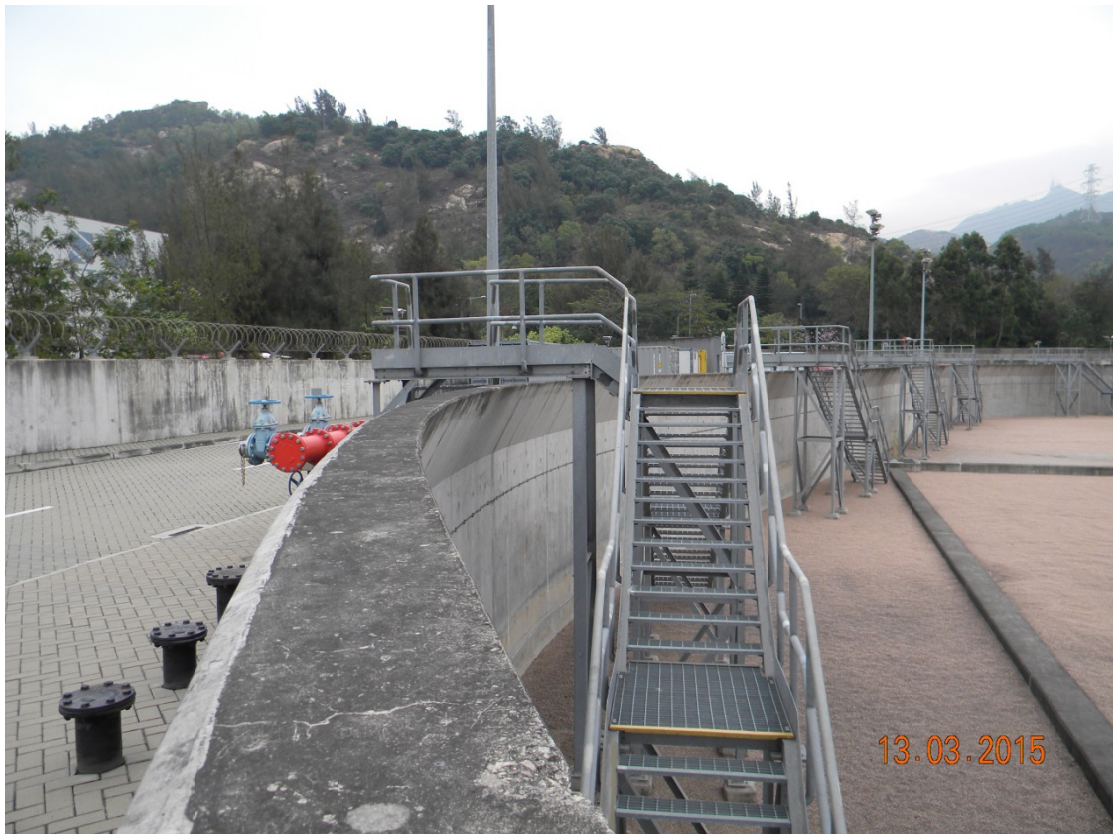
(16) This shows the thickness of the bund wall provided
