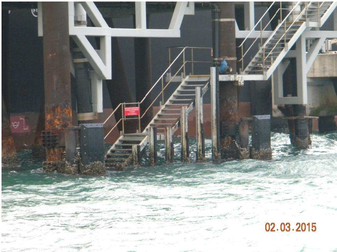
(37) Fenders installed at shore side of the jetty
