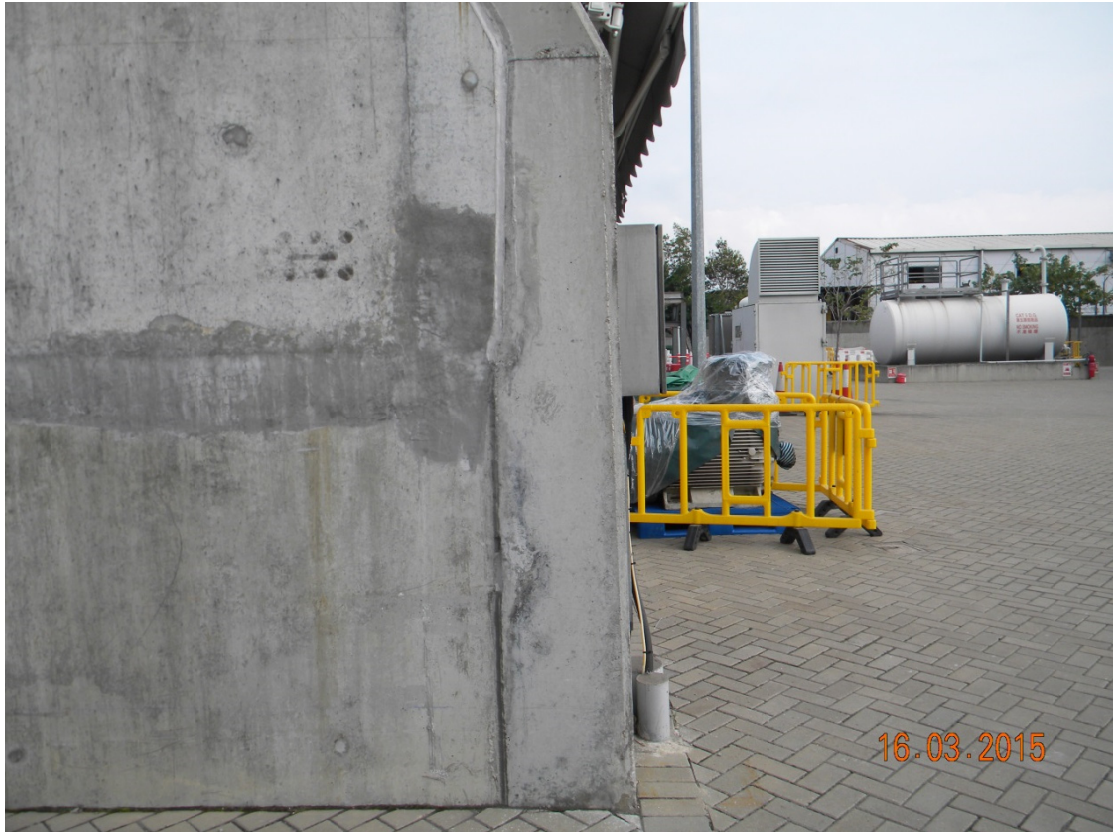
(15) This shows the thickness of the security wall provided
