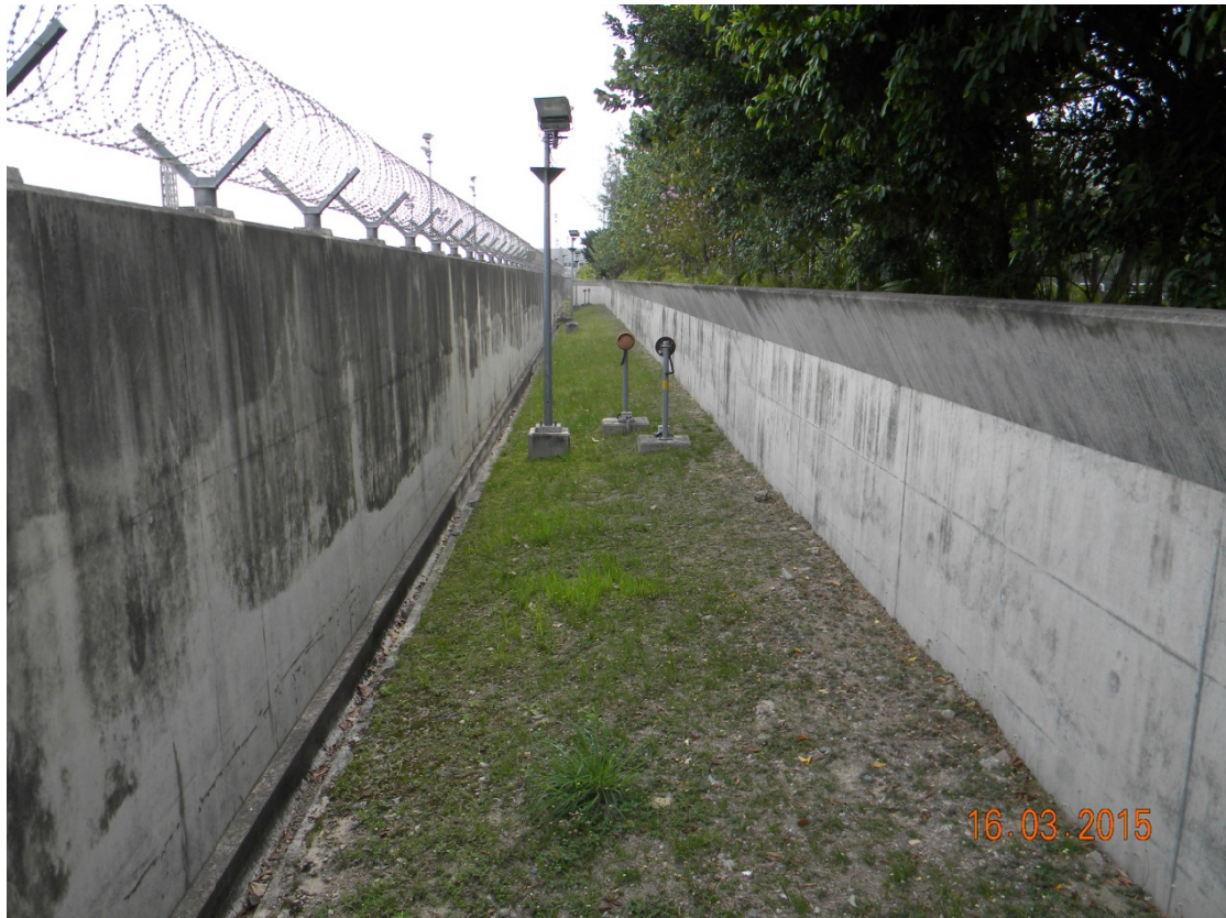
(9) Two impervious security walls are provided outside the bunded compounds
