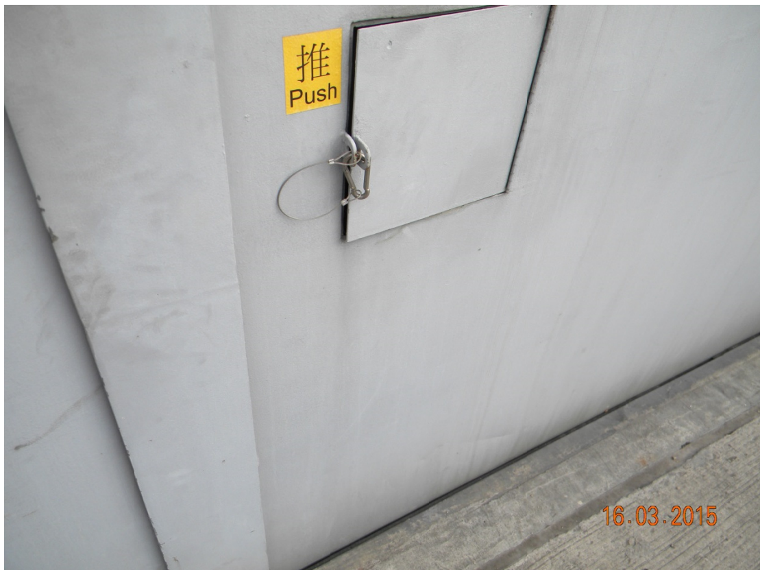
(14) Gates at security walls with sealant are maintained in good condition
