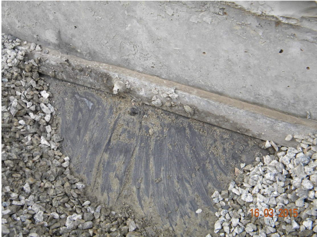
(17) Impervious lining are maintained in good condition
