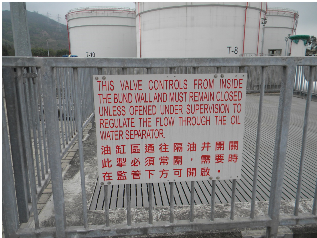
(20) Outlet valve provided for Phase 1b Interceptor with instruction sign to keep “normally closed”
