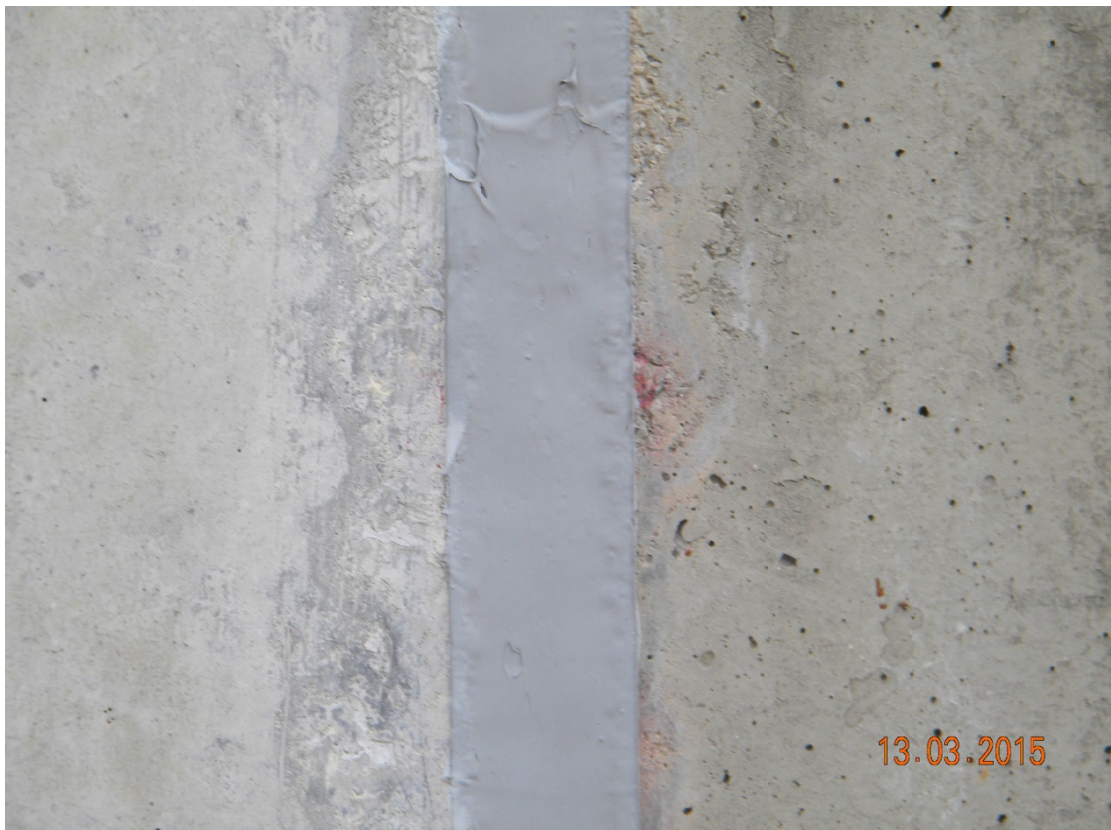
(6) Maintenance works have been performed on sealant at joints
