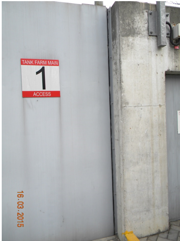
(13) Gates at security walls with sealant are maintained in good condition
