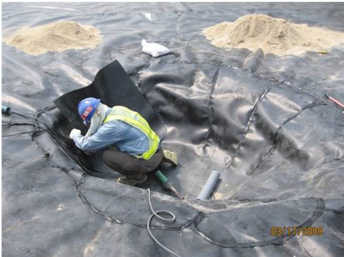
(22) Record photo shows impervious membrane laid at tank center sump with tell-tale pipe embedded for leak detection
