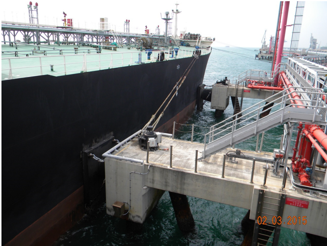
(36) Fenders installed at sea side of the jetty.
