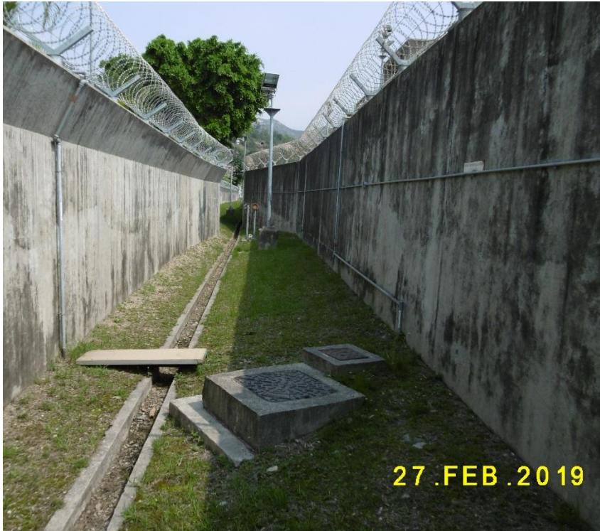
(11) Two impervious security walls are provided outside the bunded compounds
