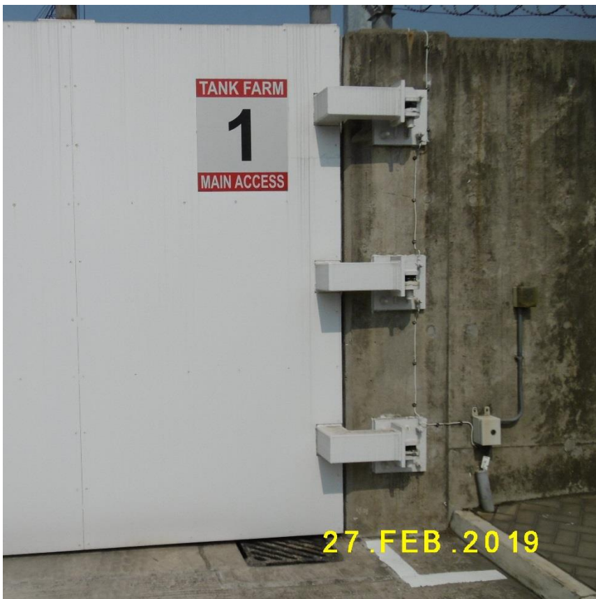
(14) Gates at security walls with sealant are maintained in good condition
