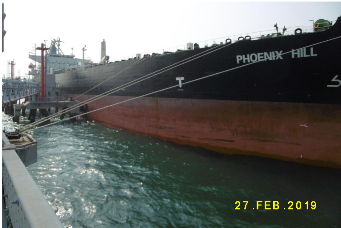
(36) Fenders are installed at sea side of the jetty
