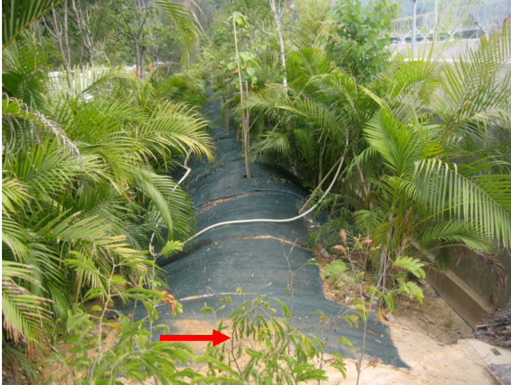
Photos 3 & 4- Example of soil erosion control matt outside boundary wall.
