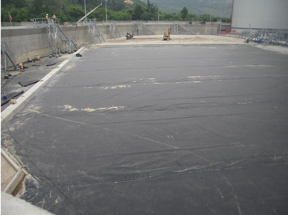
(35) Impermeable Lining of bunded areas
