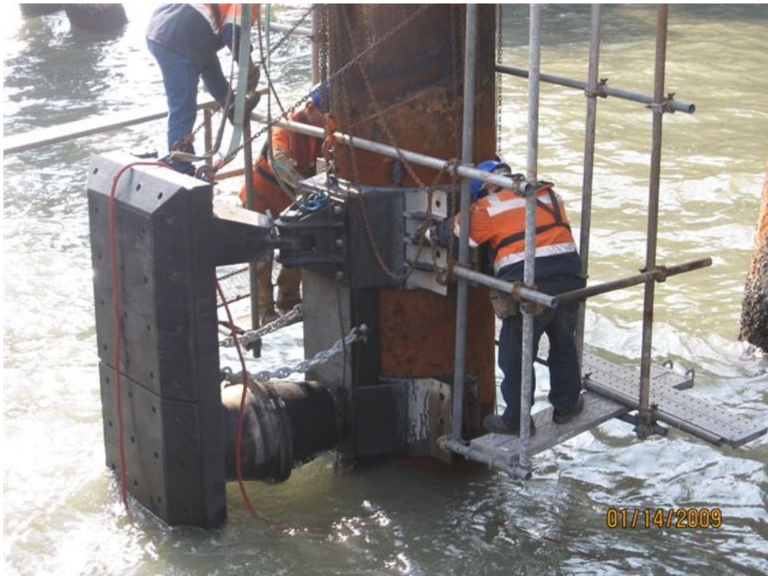
(14) LP 14-Jan-2009 Installation of PMF fender on pile
