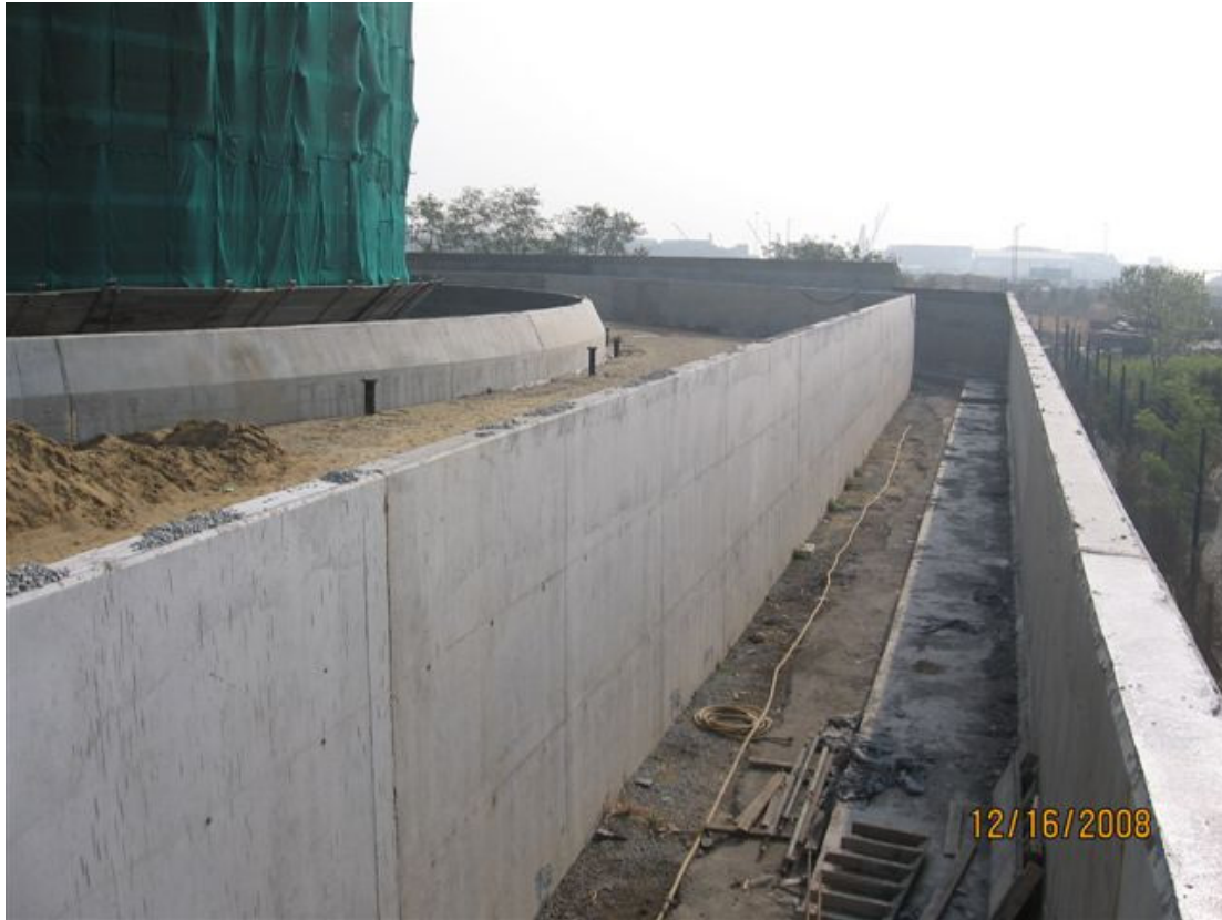
(15) Security wall 16-Dec-2008 General Condition for wall 1 & 2 behind T2 & T5
