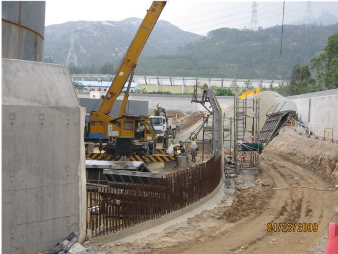
(7) Bund wall 23-Apr-2009 Stripping steel mould for wall near T11
