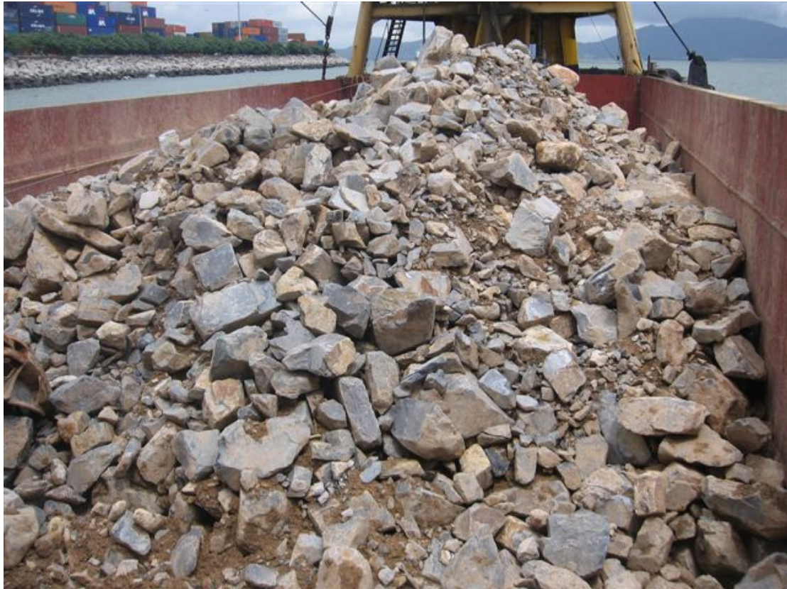
(17) Submarine pipe 23-Jun-2009 G700 rock material condition
