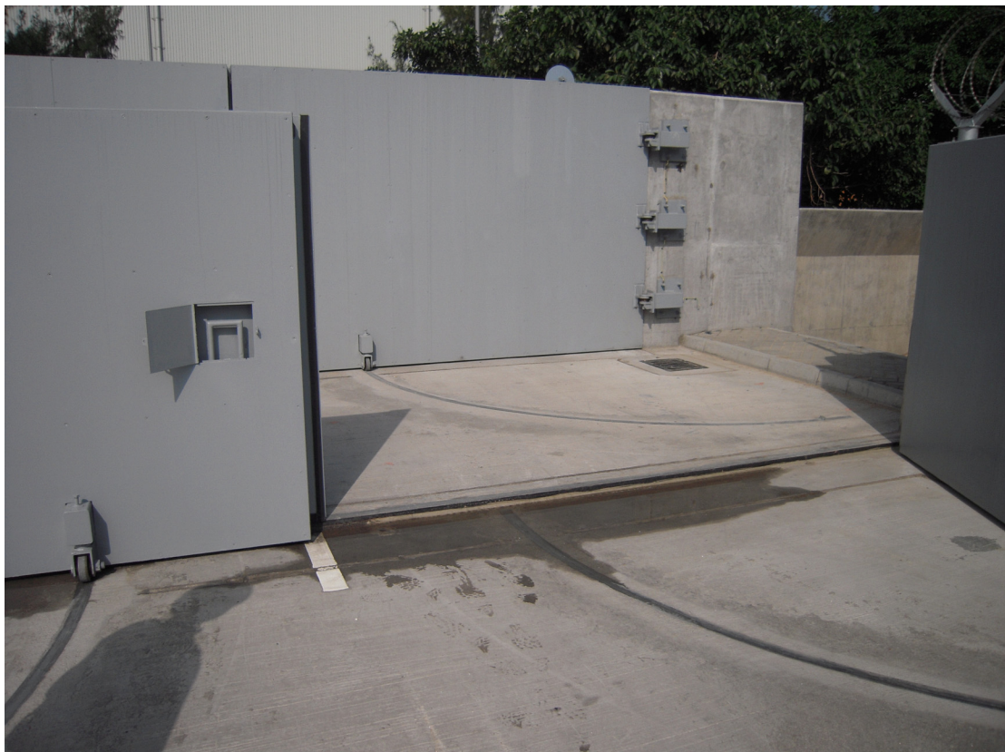
(26) Photo (4-Jan-2010) showing sealing of metal gates at security walls
