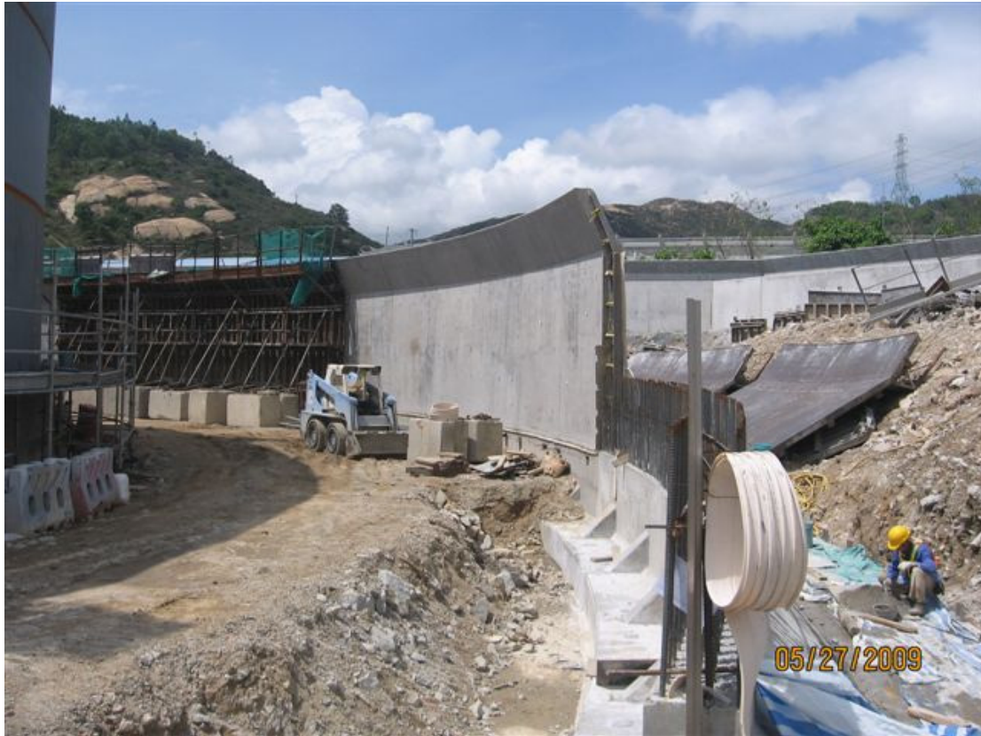
(5) Bund wall 27-May-2009 General view for wall slab behind T12
