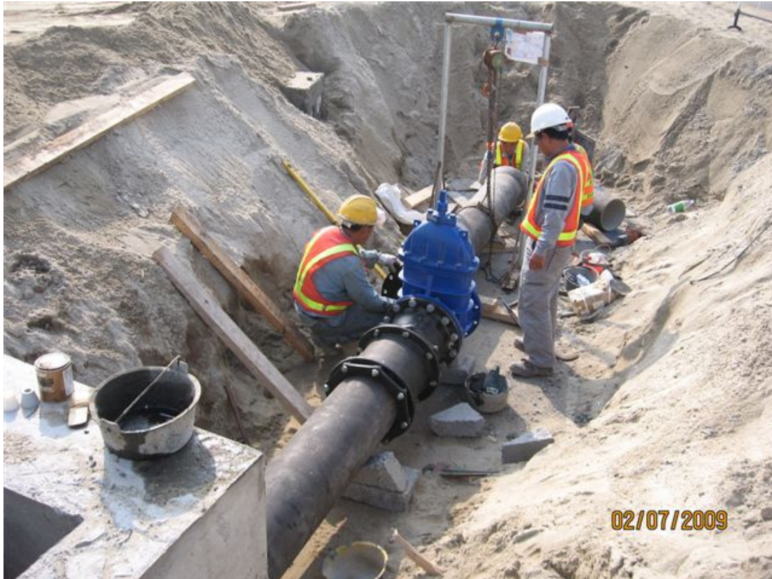
(11) Drainage 7-Feb-2009 Installation of 300 DI pipe between BM1 to G2
