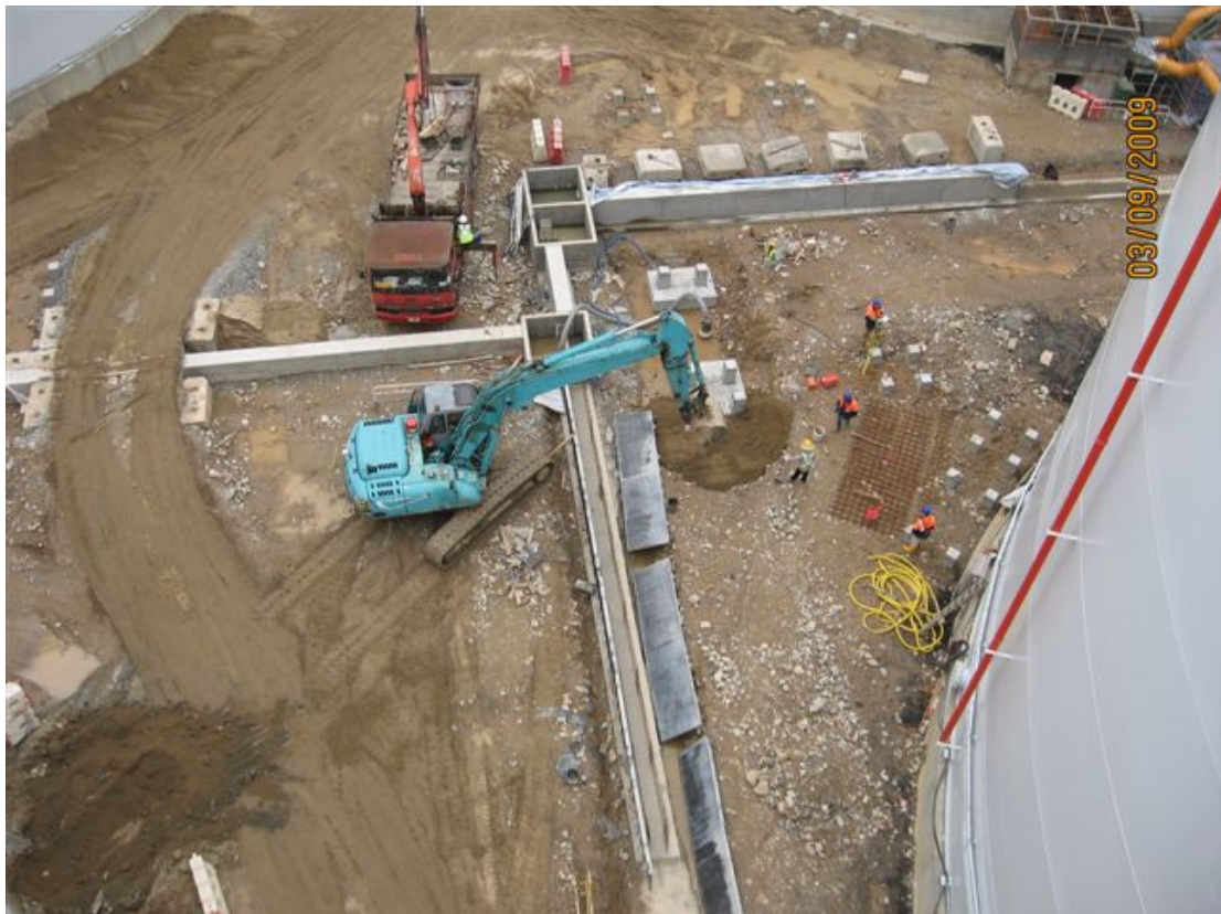
(2) Bund area 9-Mar-2009 General view for internal bund wall between T2 & T5
