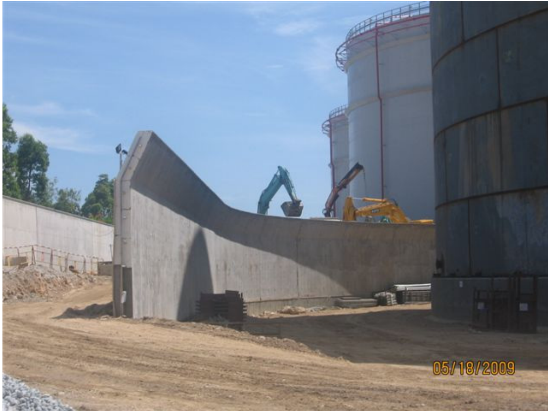
(3) Bund wall 18-May -2009 General view for wall slab near T11
