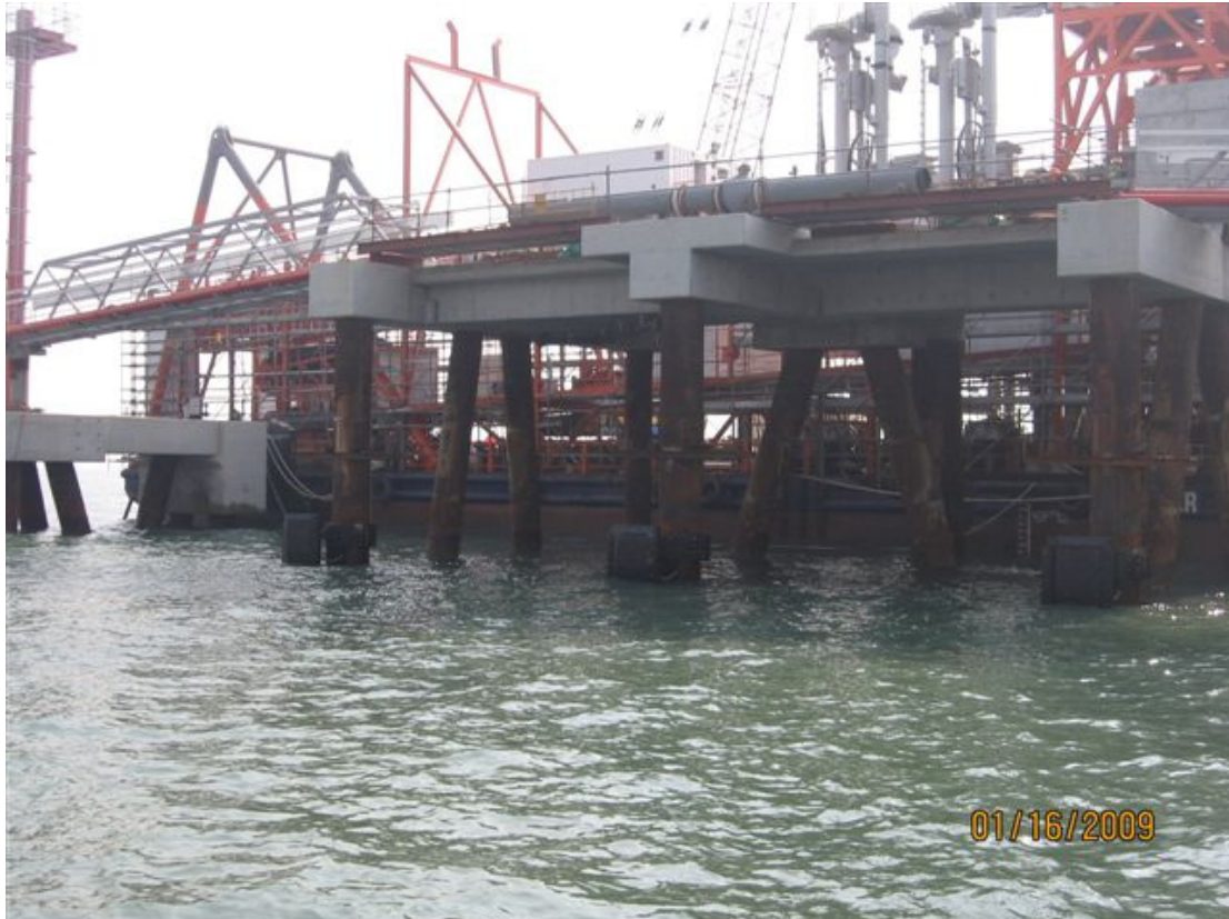
(13) LP2 16-Jan-2009 Condition of PMF fender after installation
