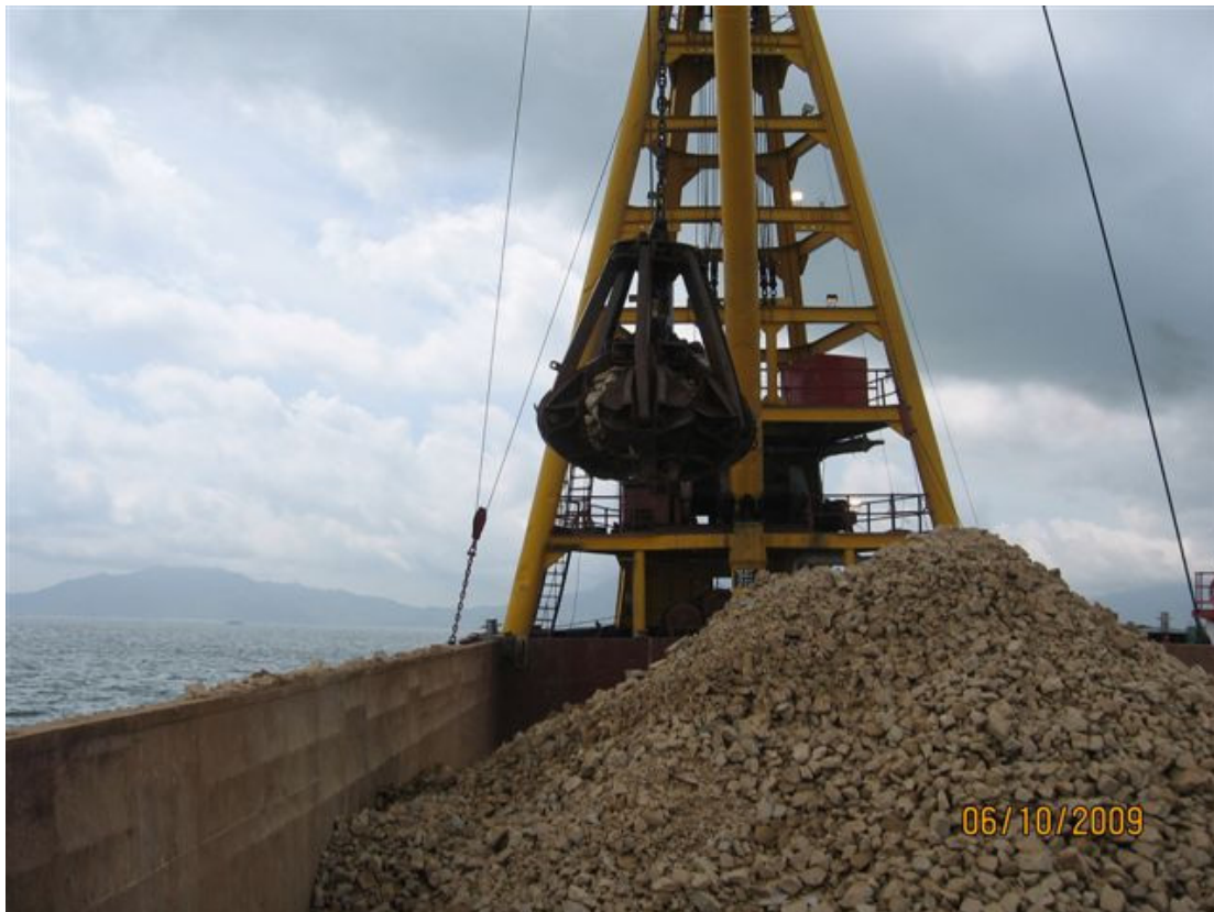
(16) Submarine pipe 10-Jun-2009 General view for rock fill in pipe trench
