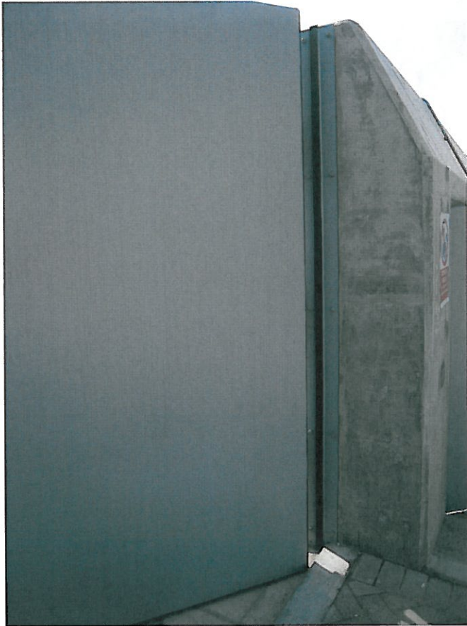
(25) Photo (4-Jan-2010) showing sealing of metal gates at security wall
