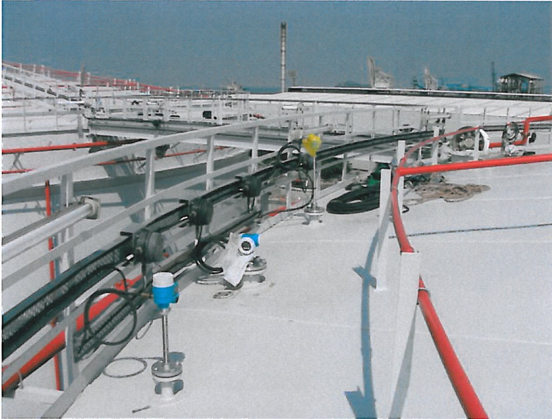
(19) Installation of HH level alarm independent of the ATG 10-Jul-2009
