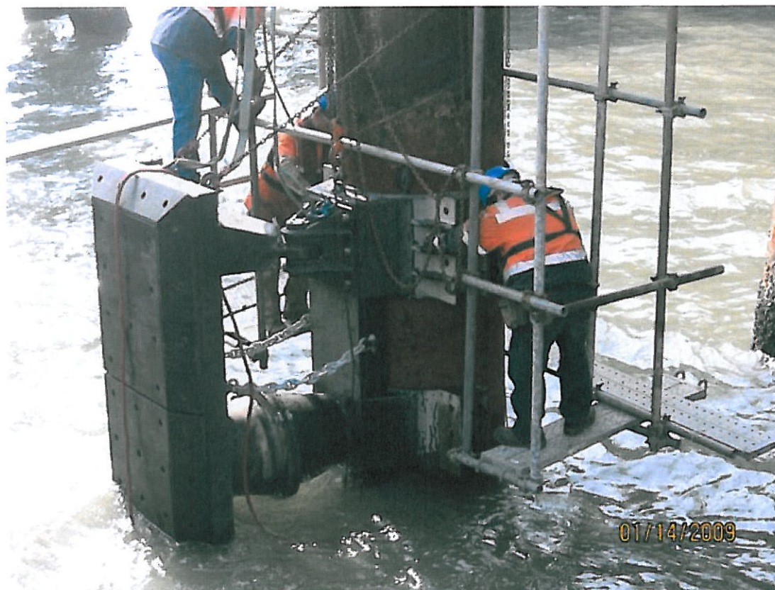
(14) LP 14-Jan-2009 Installation of PMF fender on pile
