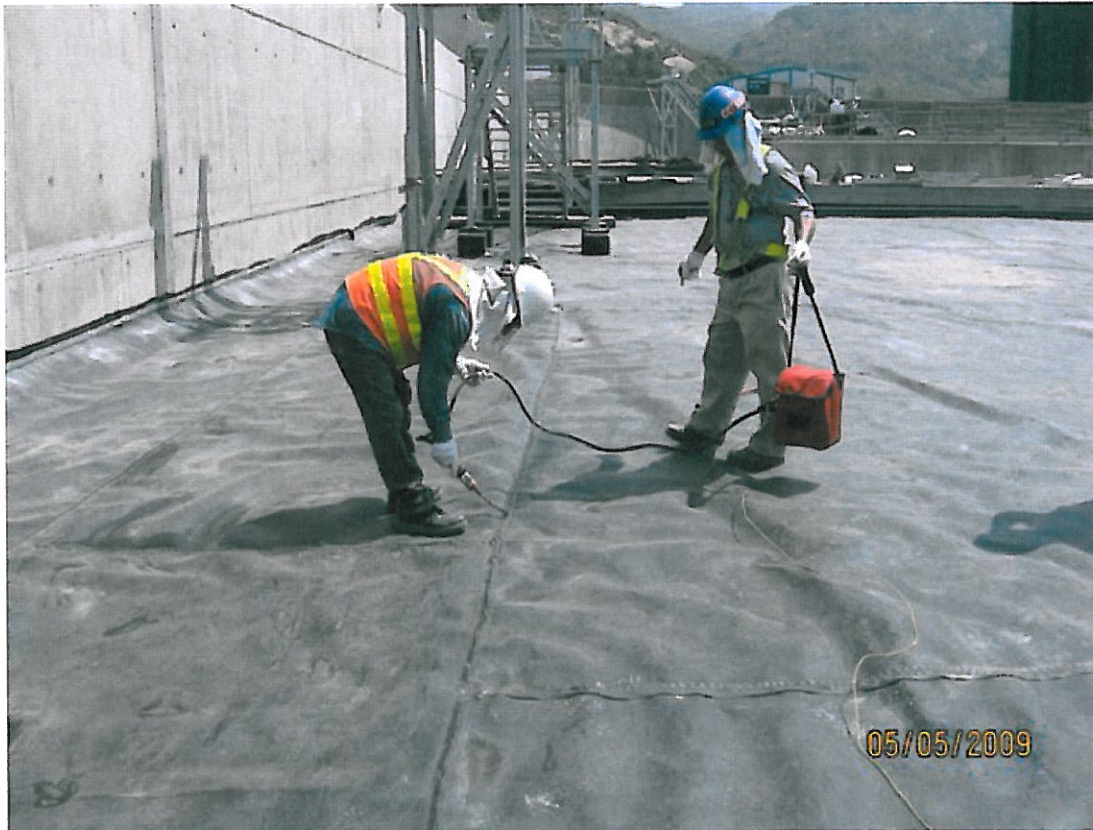
(1) Bund area 5-May-2009 Spark test for containment membrane around T1
