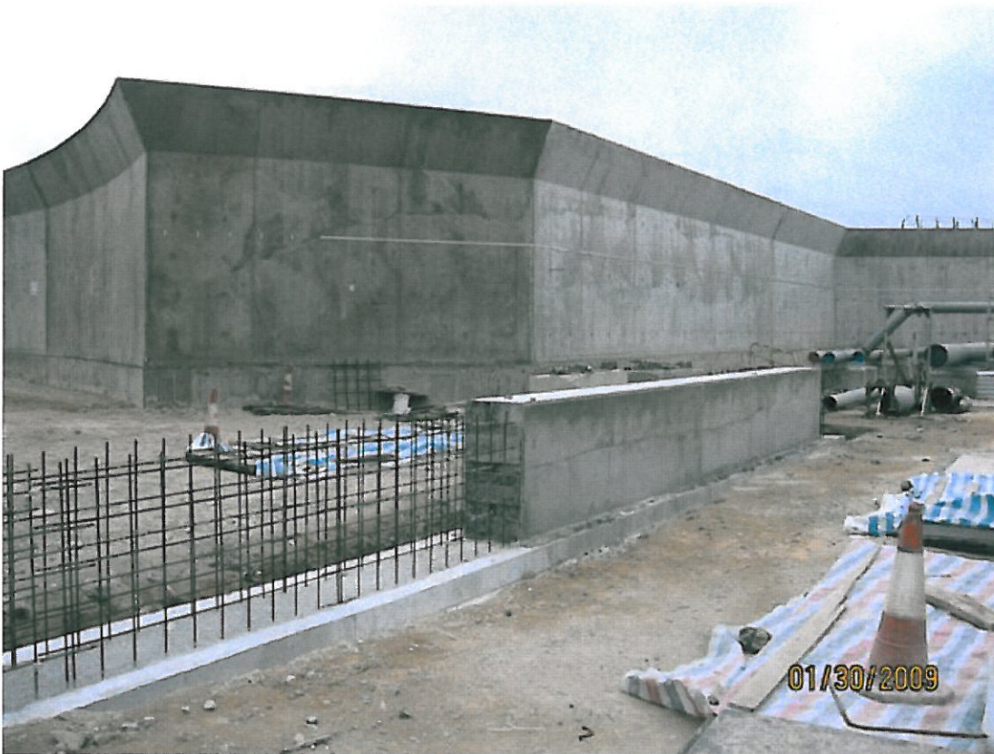
(12) Internal bund wall 30-Jan-2009 Condition of wall slab near T1
