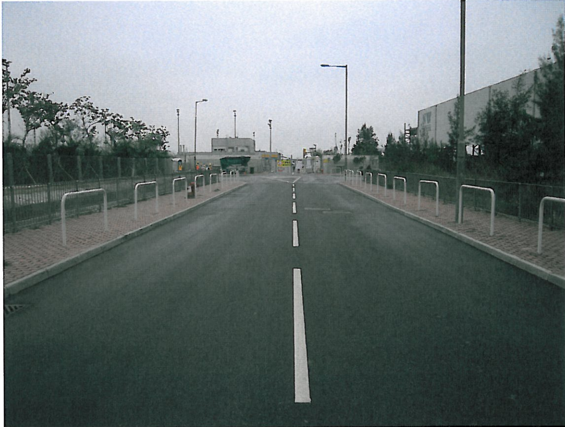
(33) Photo (4-Jan-2010) showing access road at PAFF Phase 1a under security control to designate a no waiting/parking area
