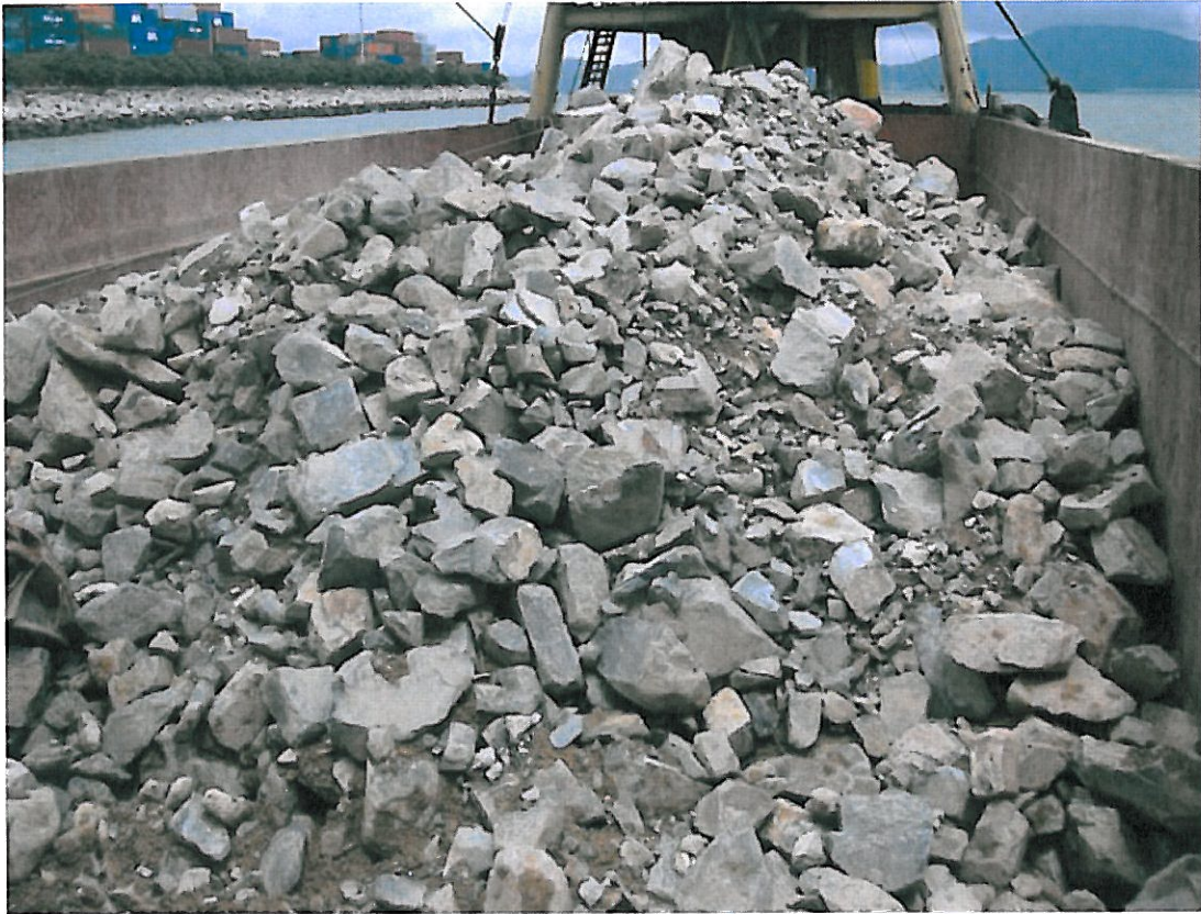
(17) Submarine pipe 23-Jun-2009 G700 rock material condition
