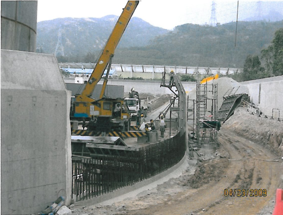
(7) Bund wall 23-Apr-2009 Stripping steel mould for wall near T11
