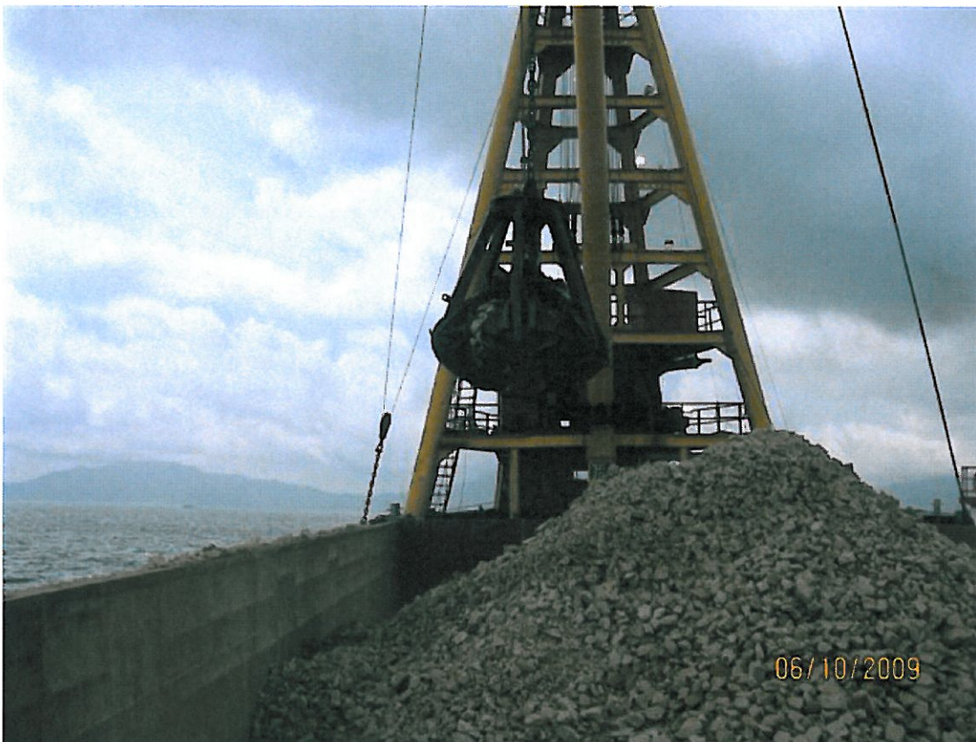
(16) Submarine pipe 10-Jun-2009 General view for rock fill in pipe trench
