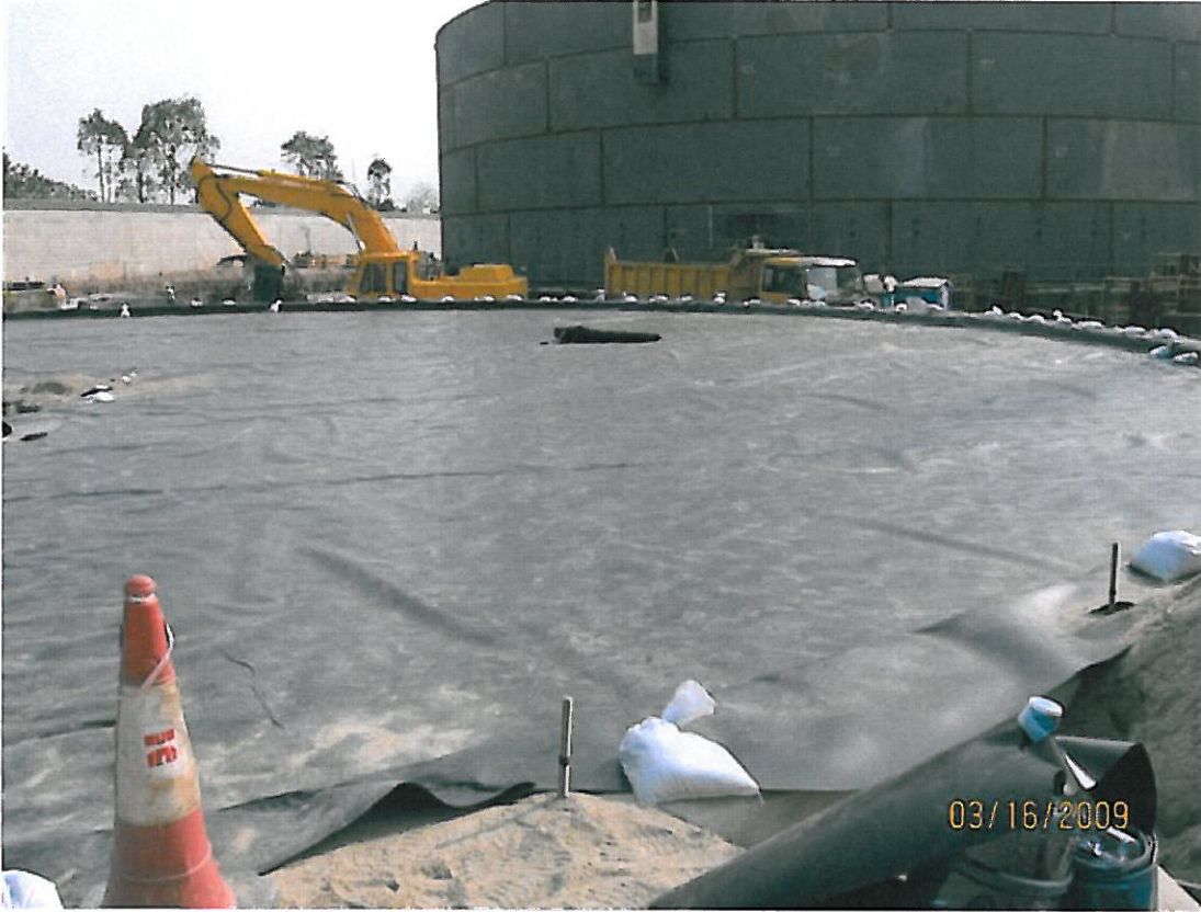
(23) Tank 16-Mar-2009 Condition of containment membrane on bottom of tank
