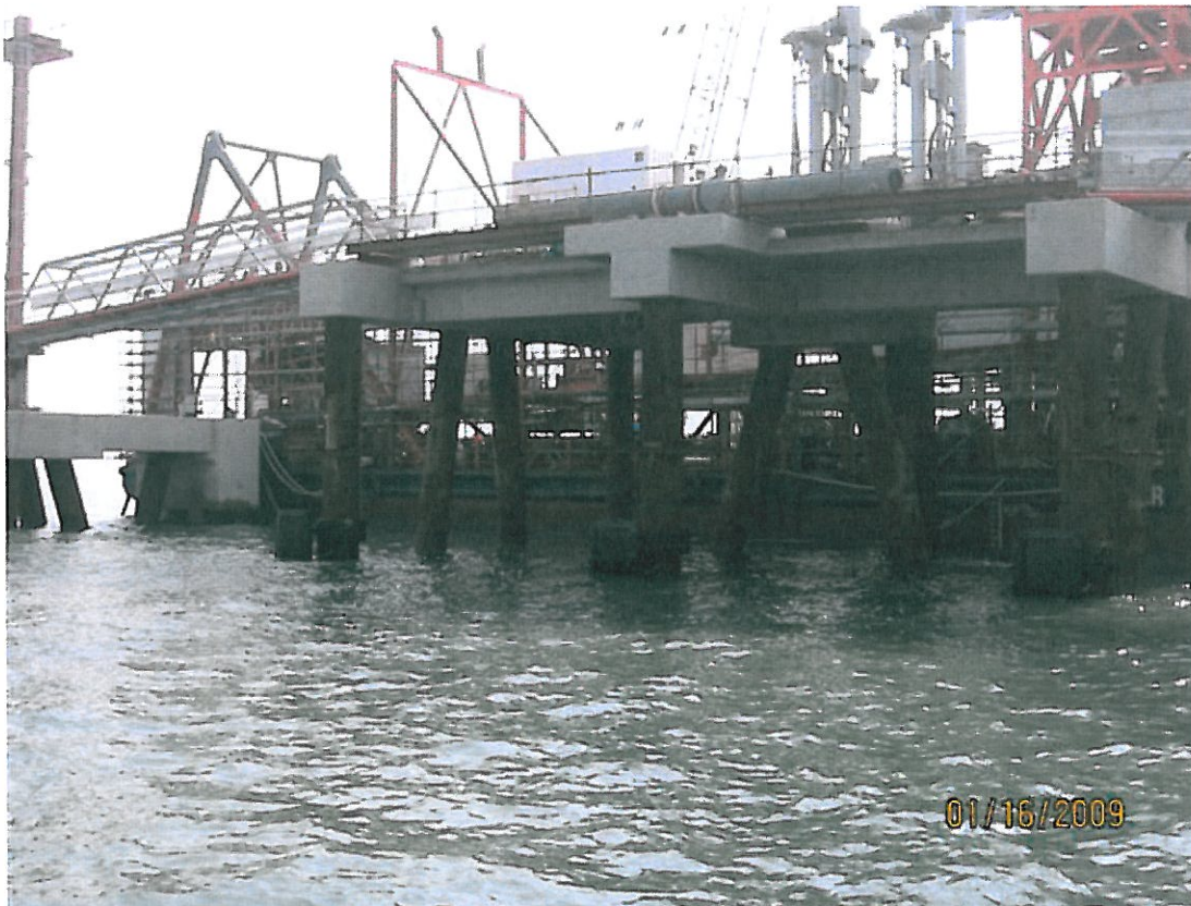
(13) LP2 16-Jan-2009 Condition of PMF fender after installation
