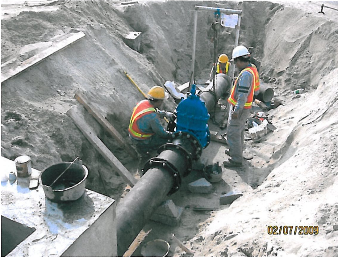
(11) Drainage 7-Feb-2009 Installation of 300 DI pipe between BM1 to G2
