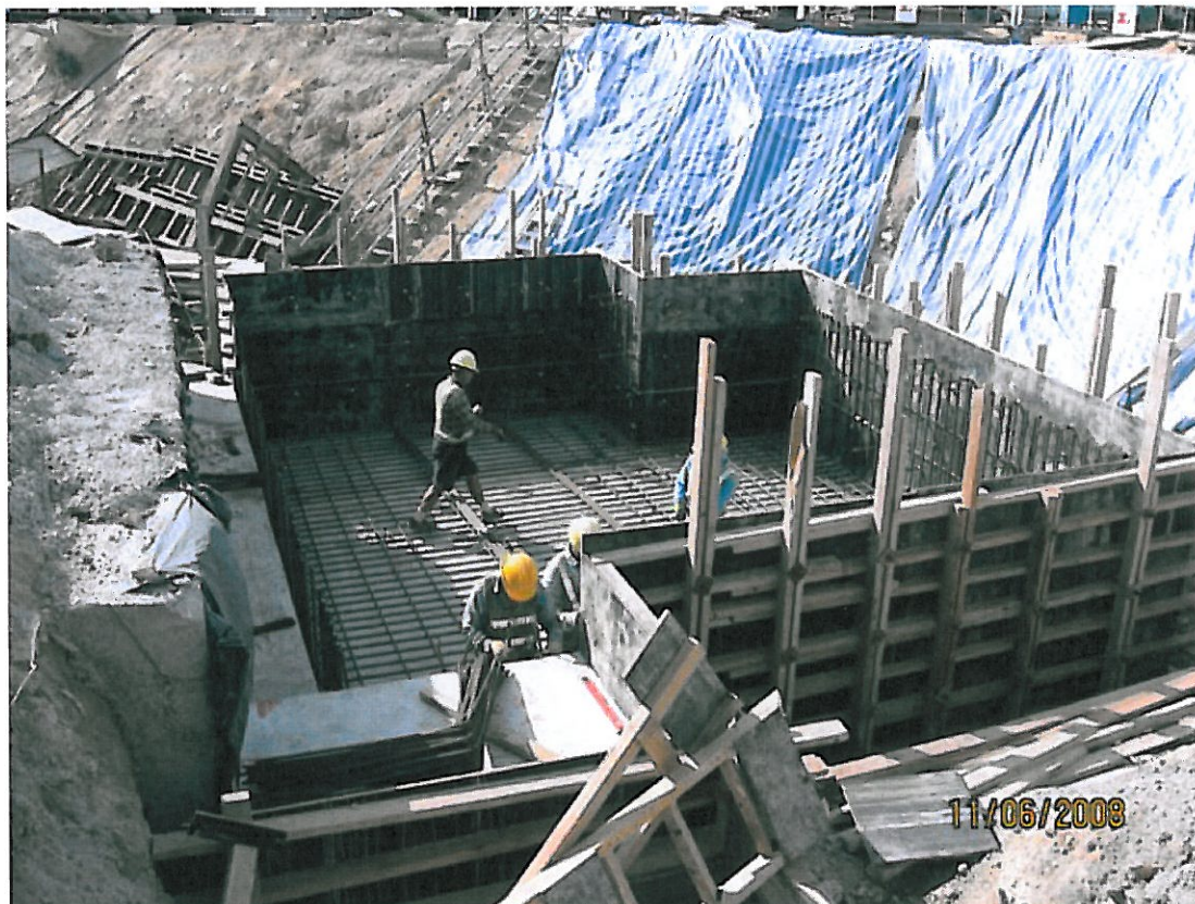
(10) Drainage 6-Nov-2008 Re-bar fixing for stage 2 oil interceptor chamber
