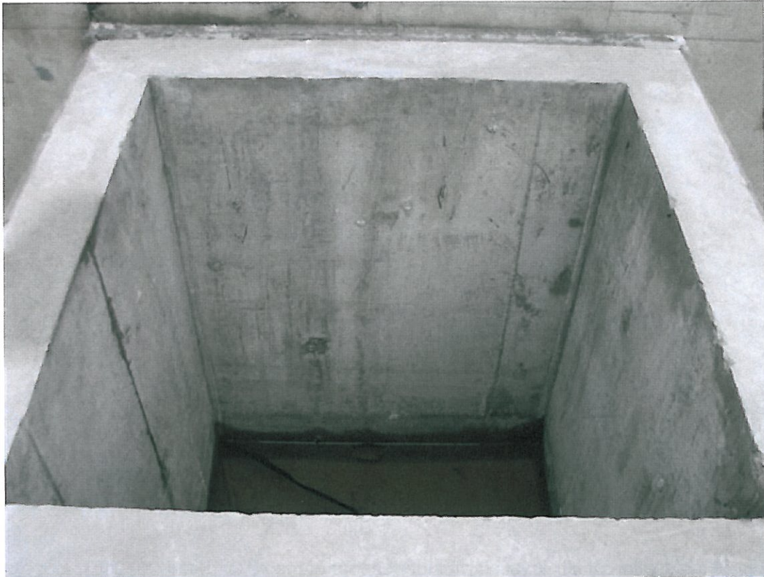
(21) Leak detection pipe underneath the storage tank opening out to a containment 15-Jul-2009
