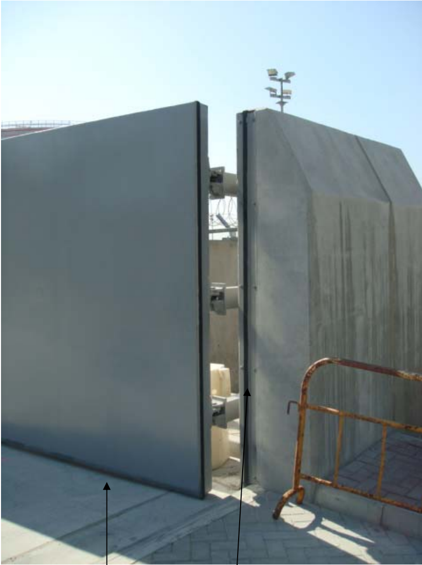
Sealant the full height and width of the gate
