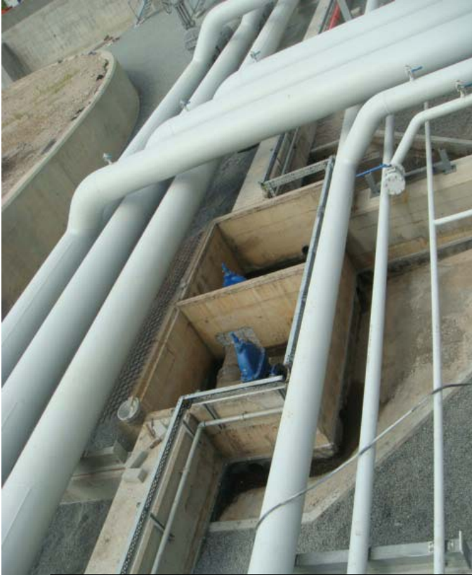
Valves inside the stormwater system inside the banded area of the tank farm
