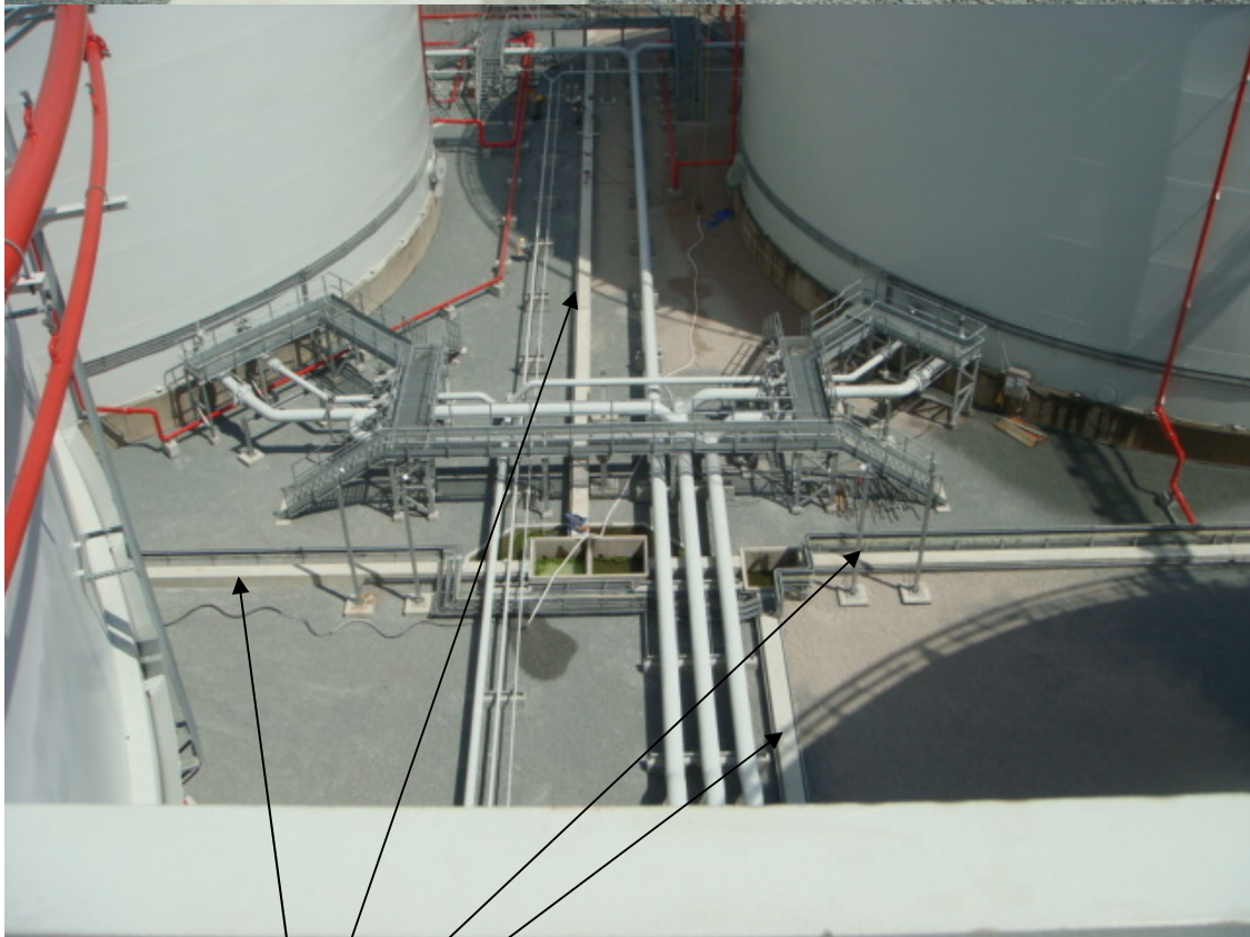
View of intermediate bunds between tanks 2, 4, 5 and 6
