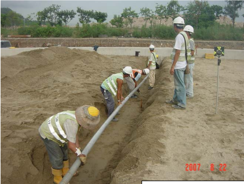
Installation of the leak detection system under the fuel tank
