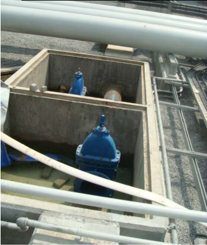
Valves inside the stormwater system inside the banded area of the tank farm
