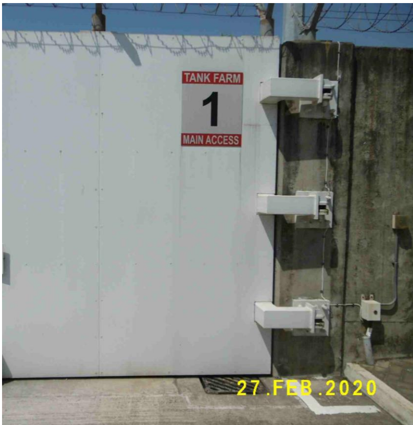
(14) Gates at security walls with sealant are maintained in good condition
