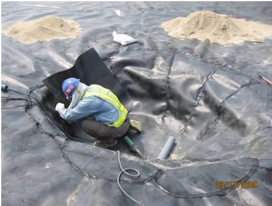
(23) Record photo shows imperious membrane laid at tank center sump with tell-tale pipe embedded for leak detection
