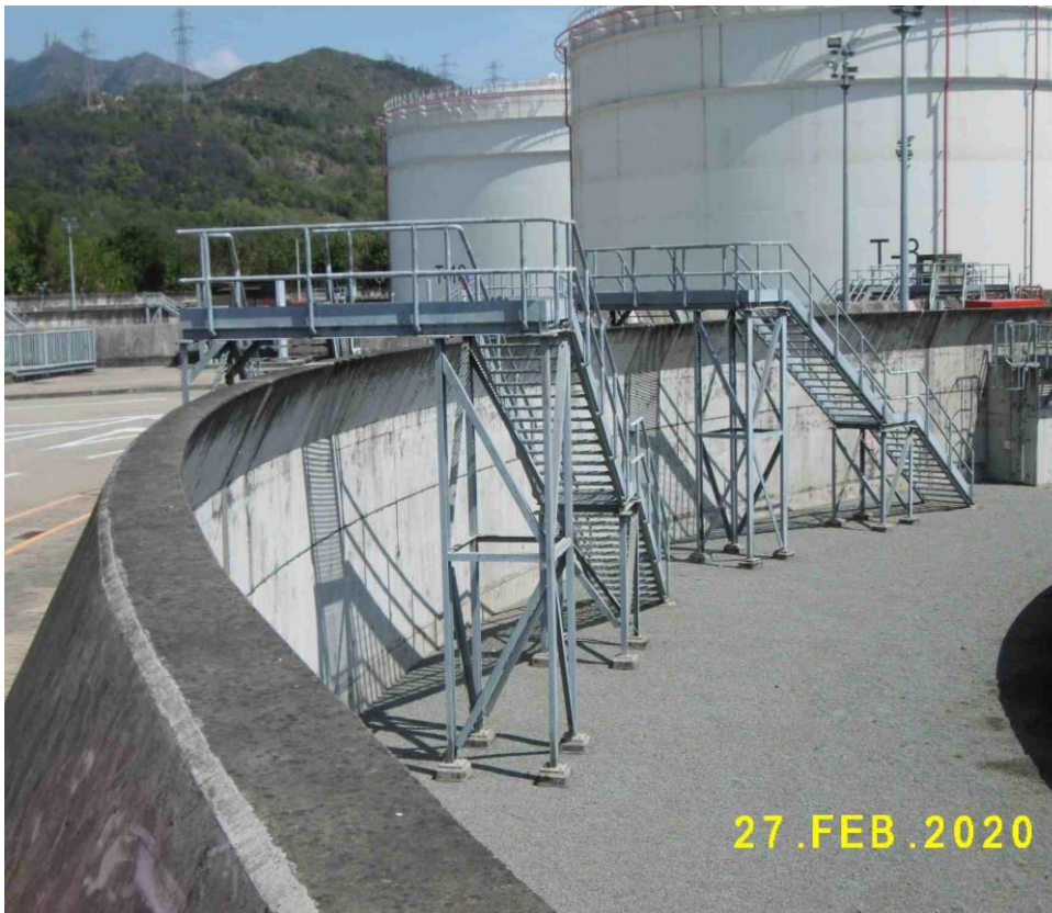
(5) Wave deflector is located at top of the bund
