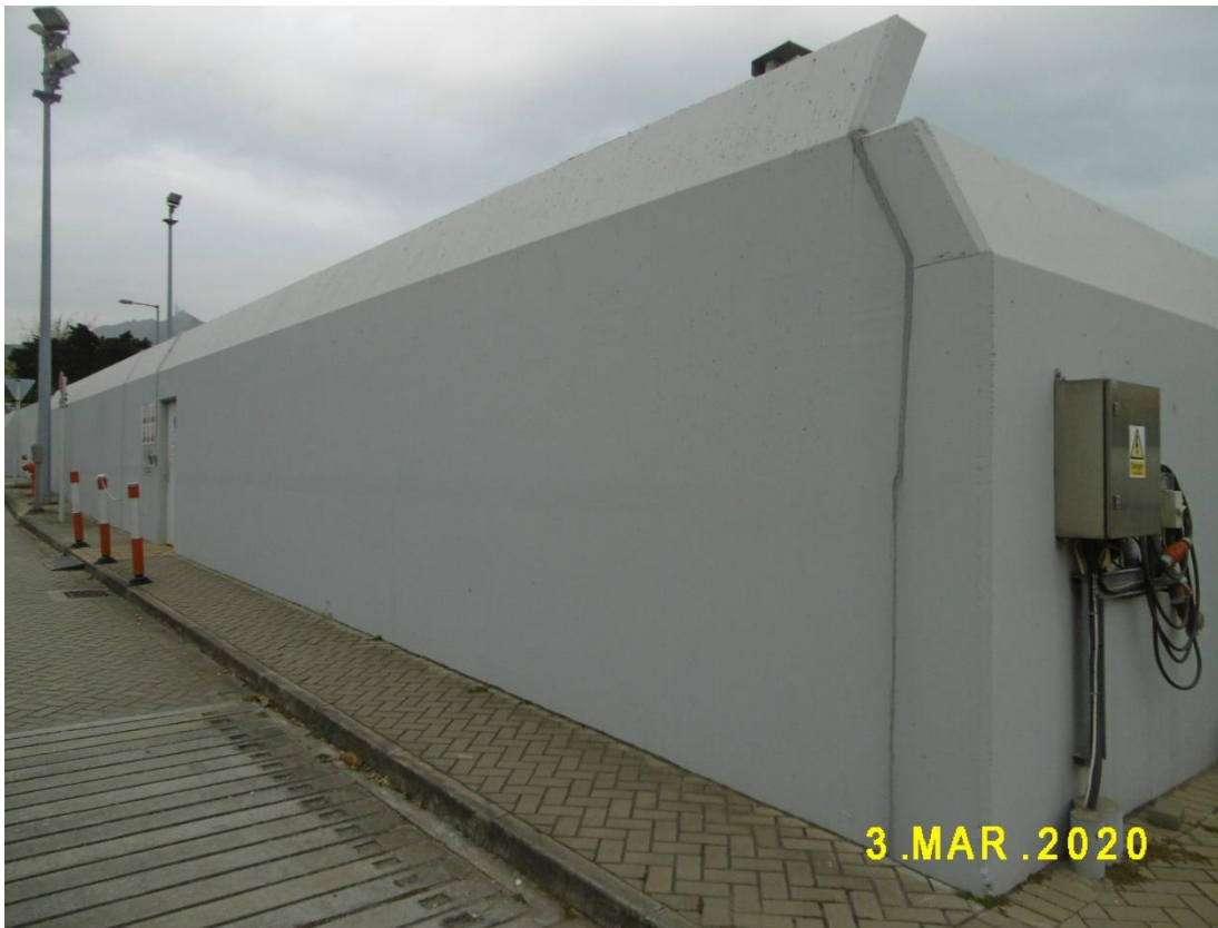
(17) This shows the thickness of the security wall provided
