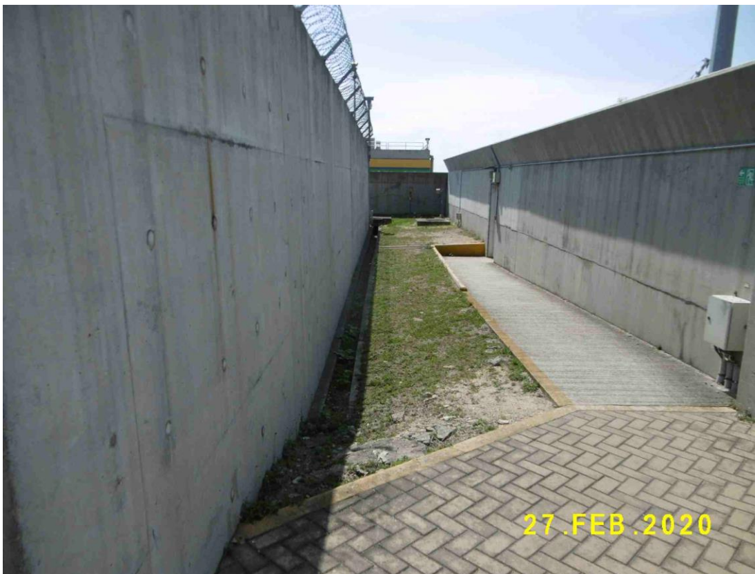
(10) Two impervious security walls are provided outside the bunded compounds
