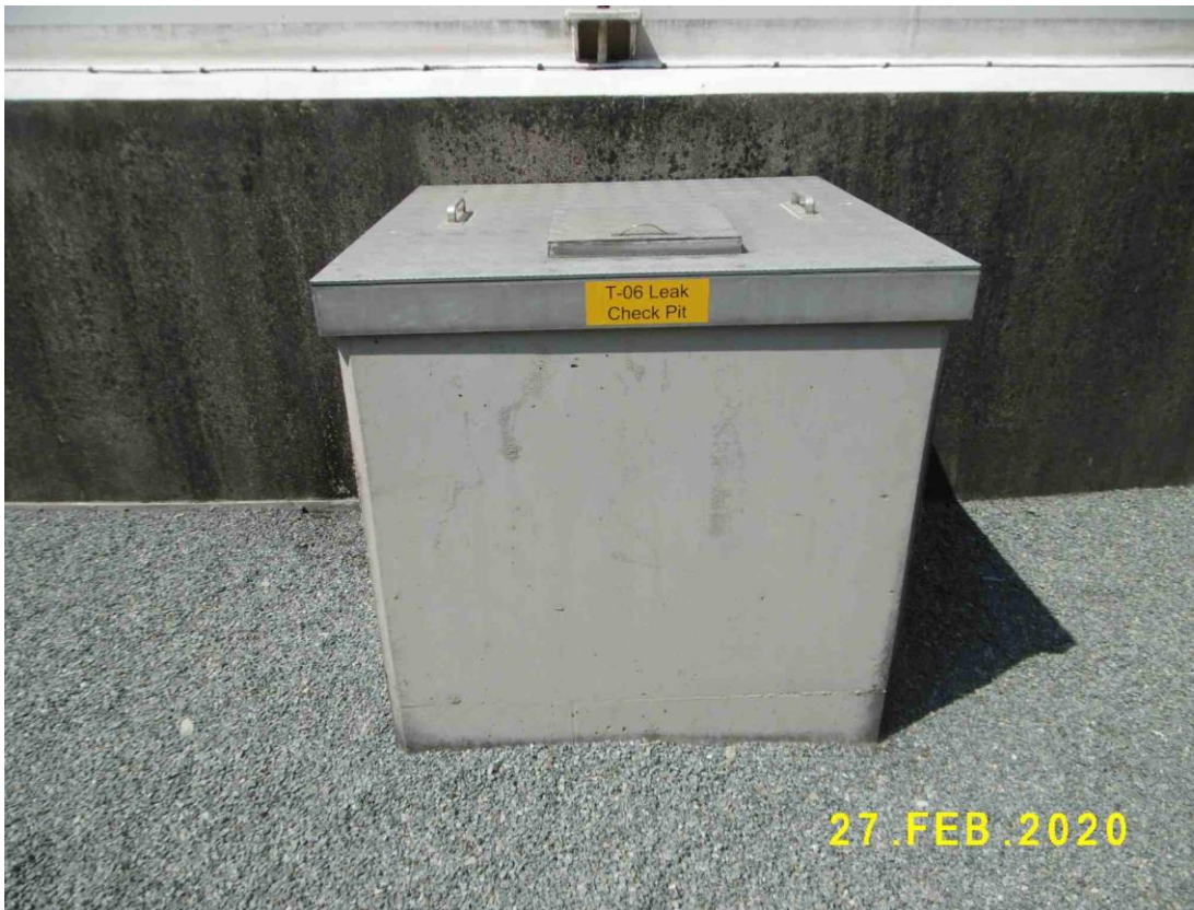
(29) Collection chamber located adjacent to tank foundation is maintained in good condition with periodic inspection
