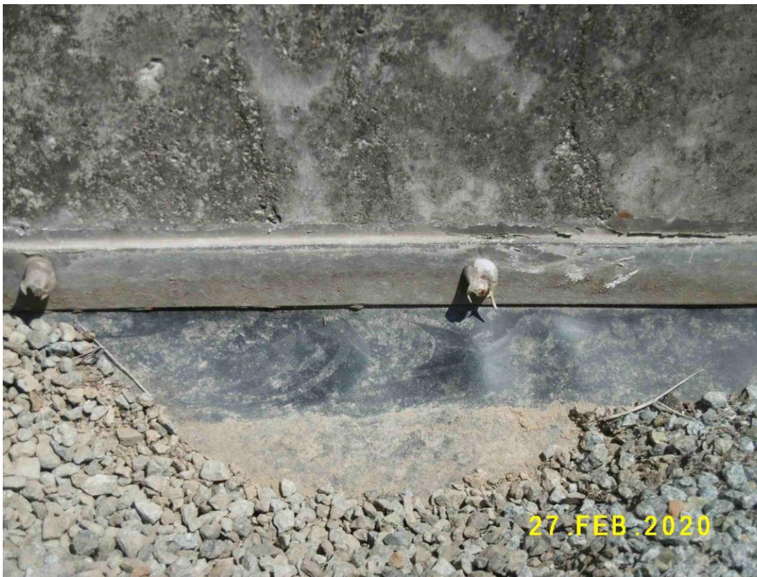
(18) Impervious lining are maintained in good condition
