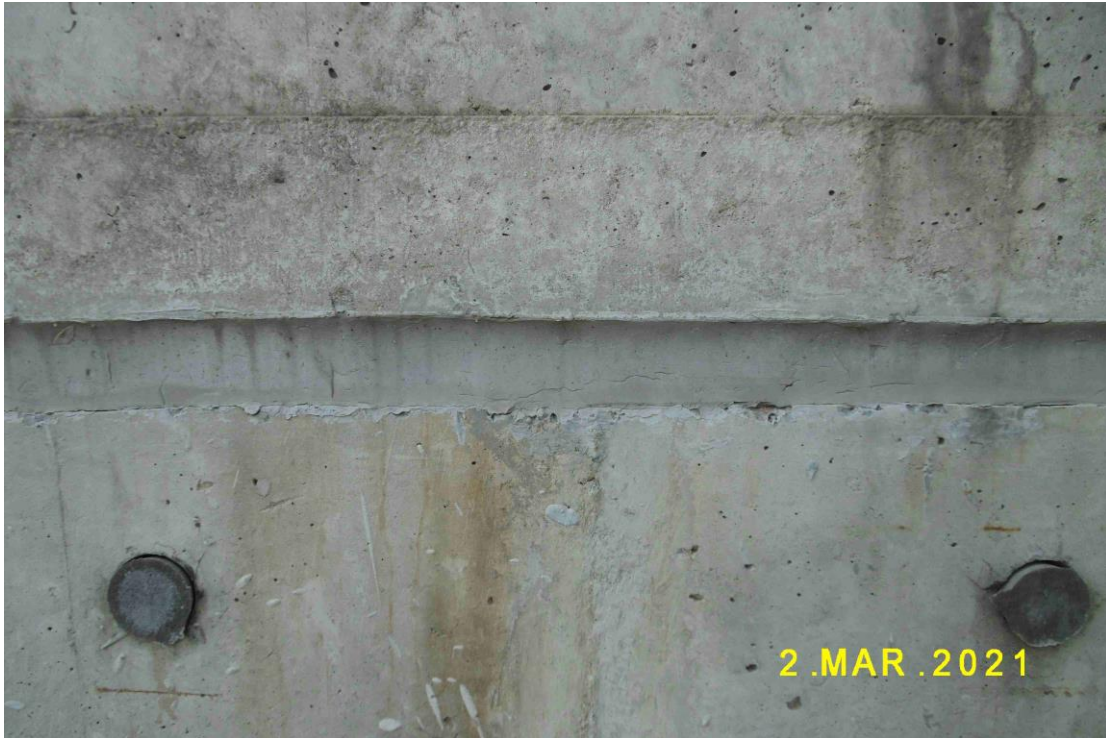
(7) Maintenance works have been performed on sealant at joints
