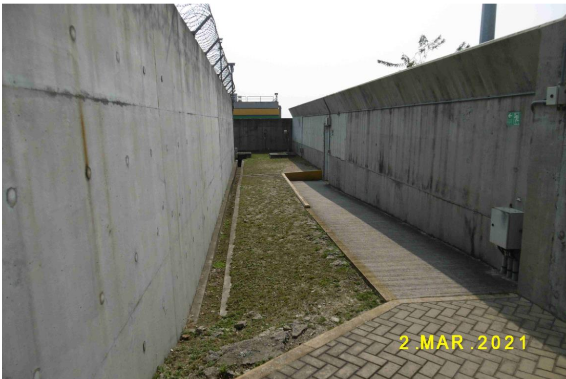
(10) Two impervious security walls are provided outside the bunded compounds
