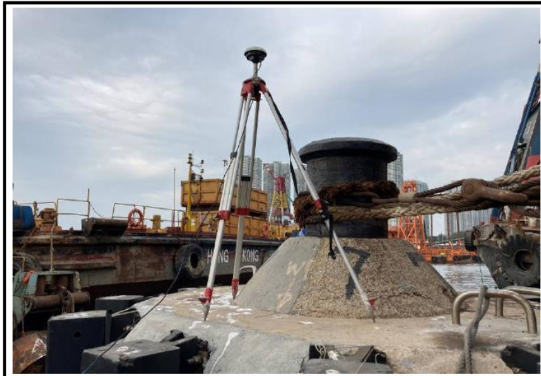
Plate 4: DGPS check at Tuen Mun Typhoon Shelter
