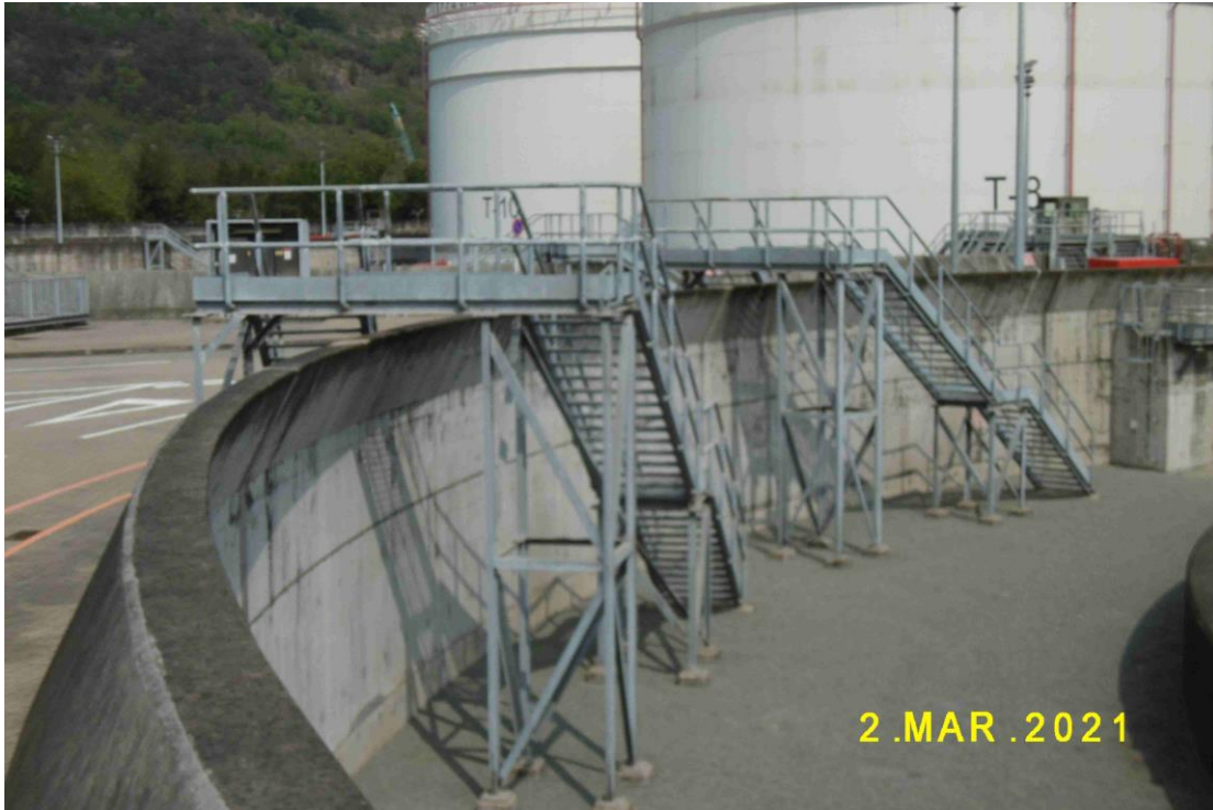
(5) Wave deflector is located at top of the bund
