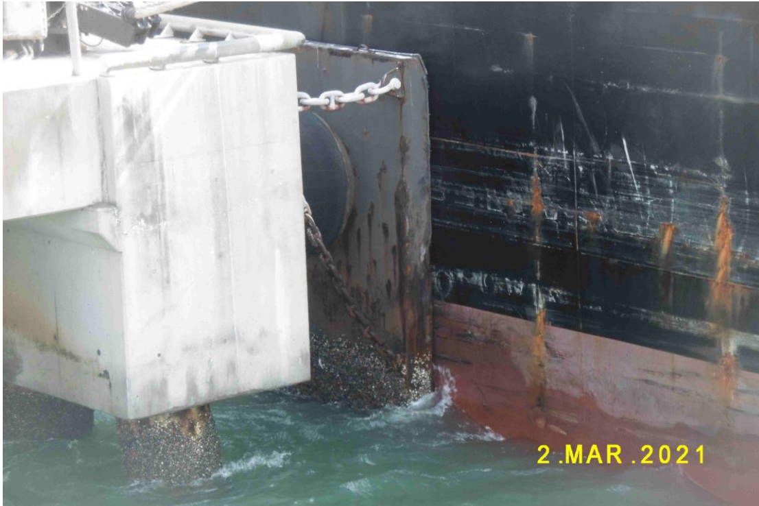
(37) Fenders are installed at sea side of the jetty
