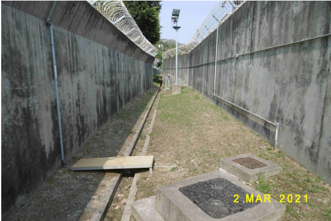
(11) Two impervious security walls are provided outside the bunded compounds
