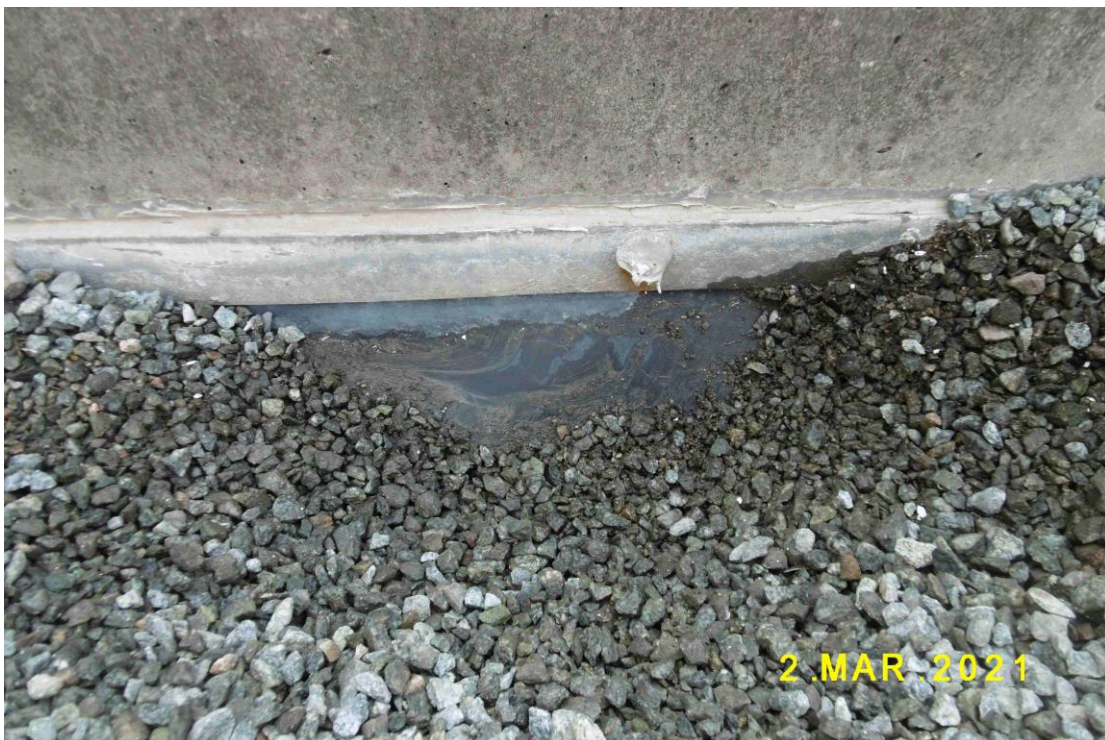
(18) Impervious lining are maintained in good condition
