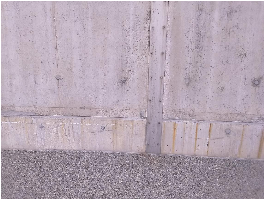
(6) Visible parts of the joints are covered by stainless steel plates on the inside at phase 1a bund
