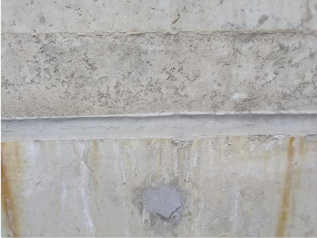
(7) Maintenance works have been performed on sealant at joints
