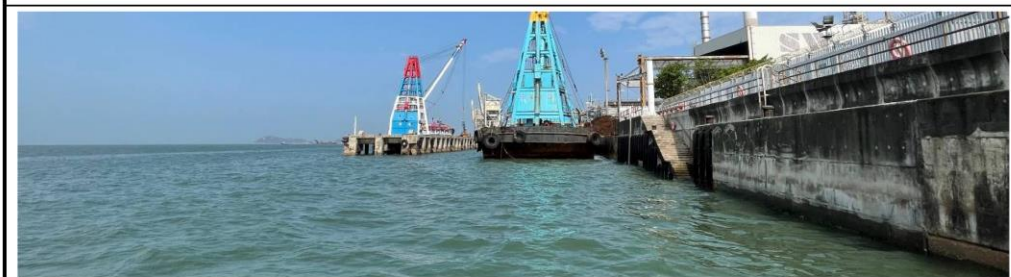
Plate 2: Sea front of the shore facility at Tuen Mun
