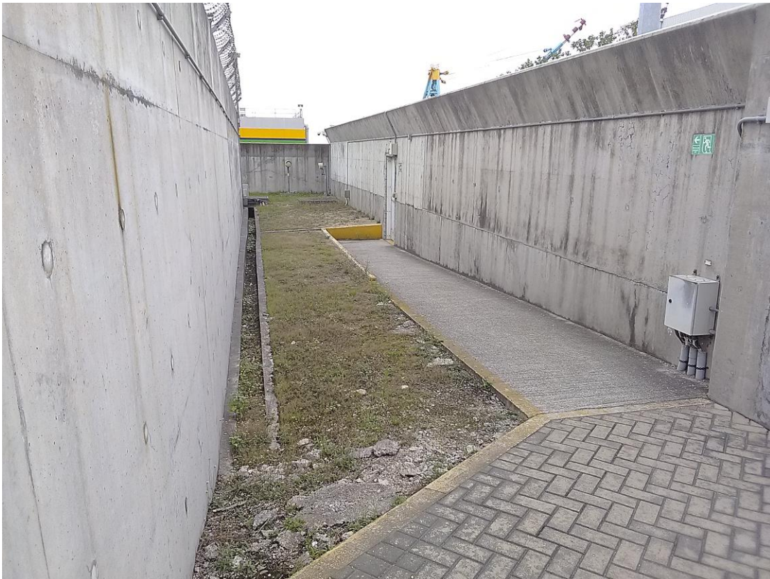
(10) Two impervious security walls are provided outside the bunded compounds
