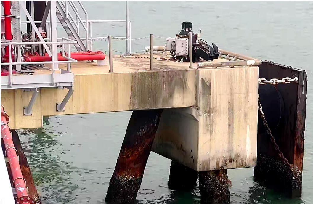
(37) Fenders are installed at sea side of the jetty
