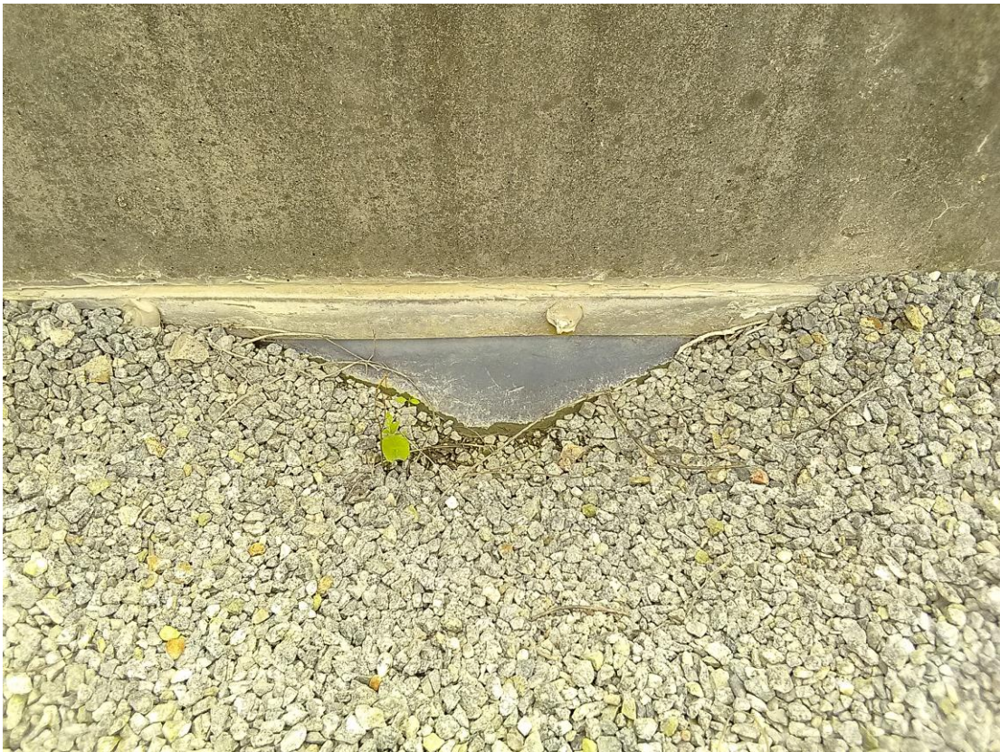
(18) Impervious lining are maintained in good condition
