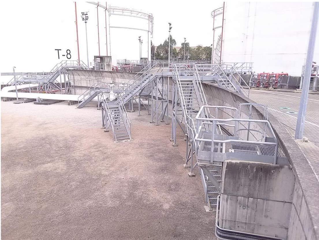
(4) Phase 1b bunded compound is lower than the ground level outside the bunds
