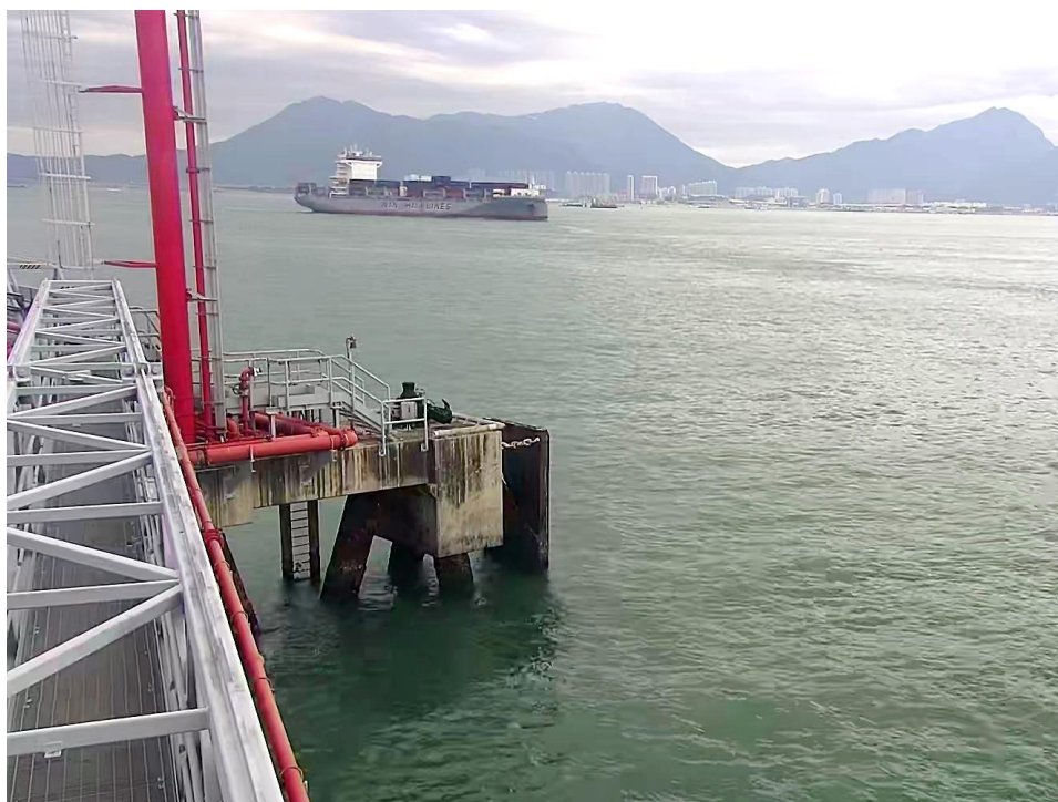
(36) Fenders are installed at sea side of the jetty
