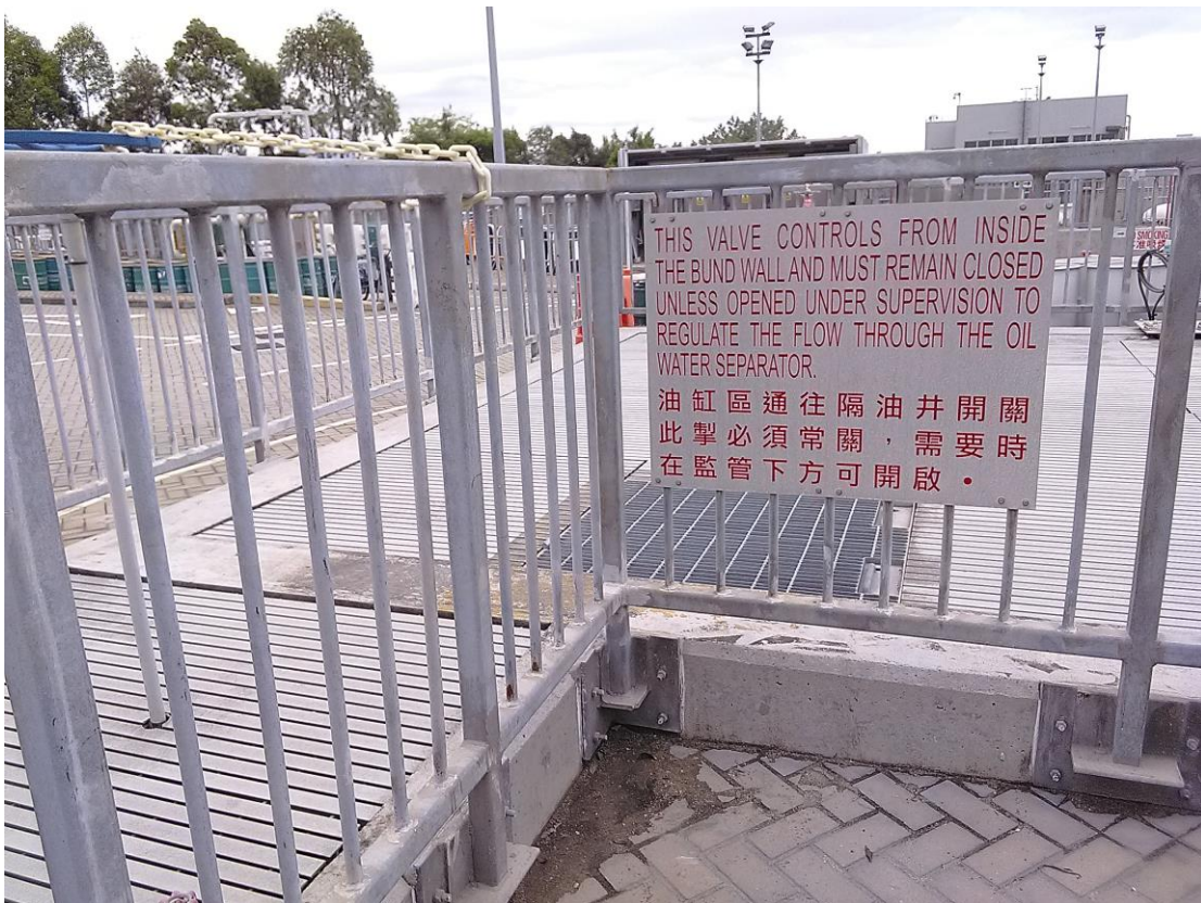
(20) Outlet valve provided for Phase 1a Interceptor with instruction sign to keep “normally closed”
