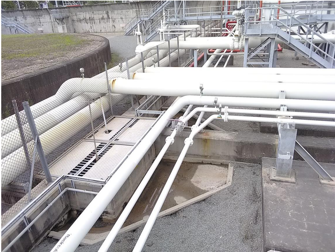
(19) Tank farm is with appropriate gradient and the drainage falls to interceptor for collection
