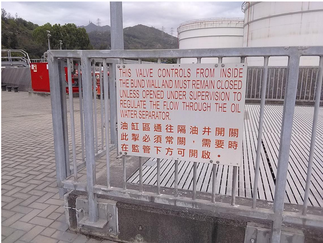
(21) Outlet valve provided for Phase 1b Interceptor with instruction sign to keep “normally closed”
