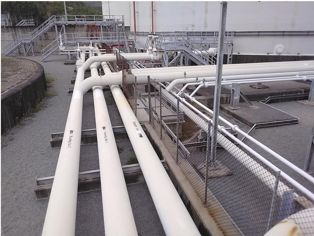
(8) Intermediate bund walls are provided in place near T-01-004
