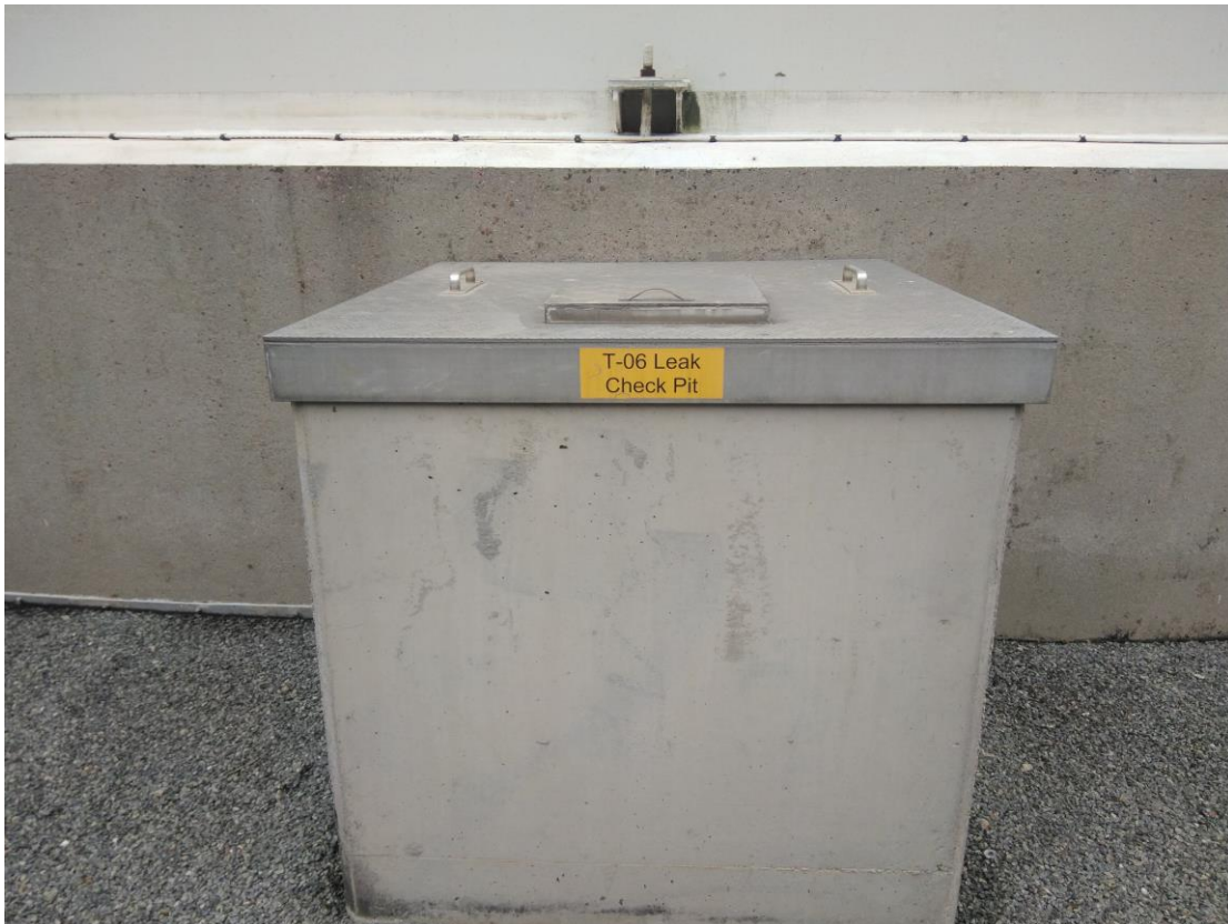
(29) Collection chamber located adjacent to tank foundation is maintained in good condition with periodic inspection
