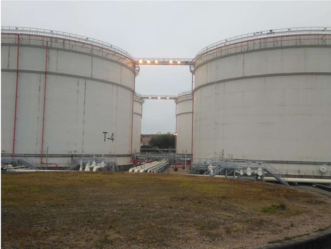
(1) Four tanks are located within bunded compound – Phase 1a
