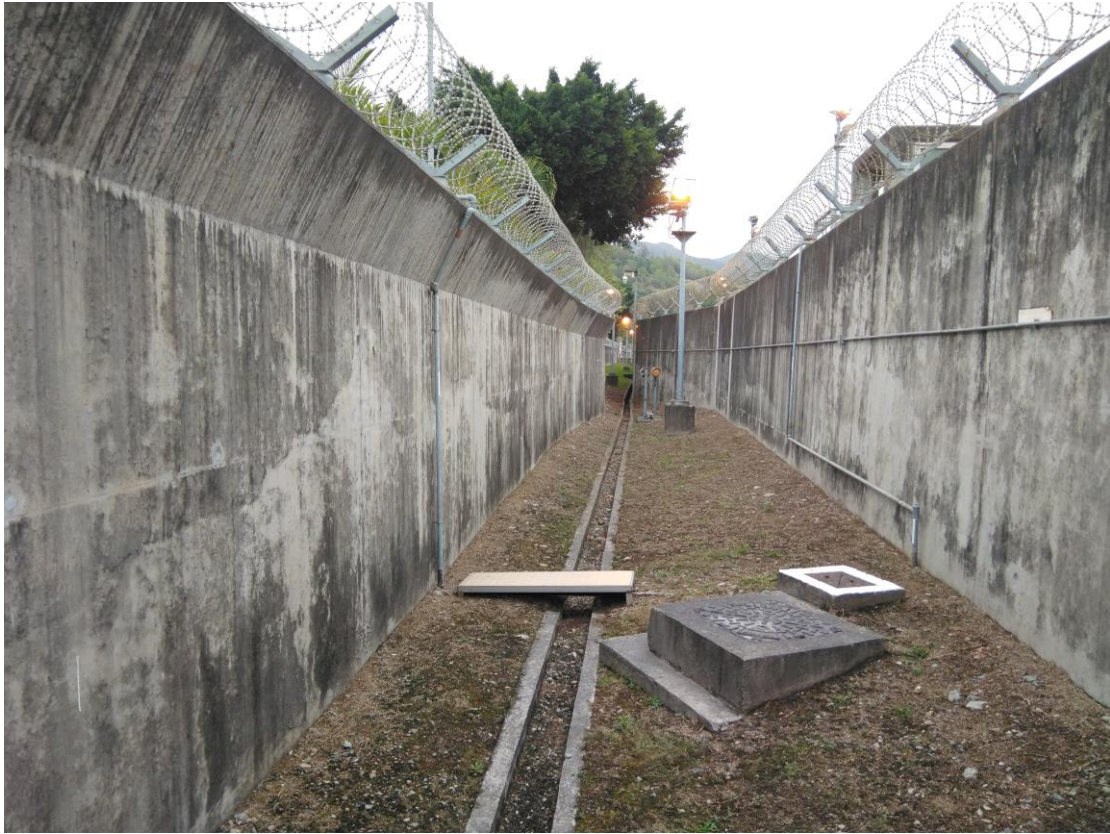
(11) Two impervious security walls are provided outside the bunded compounds
