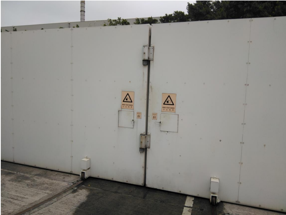
(15) Gates at security walls with sealant are maintained in good condition
