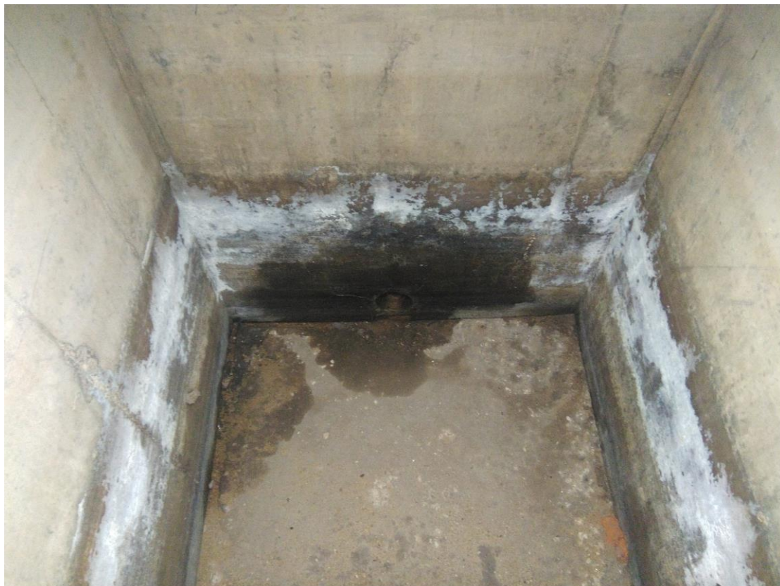
(28) Leak detection tell-tale pipe underneath the storage tank opens out to a collection chamber
