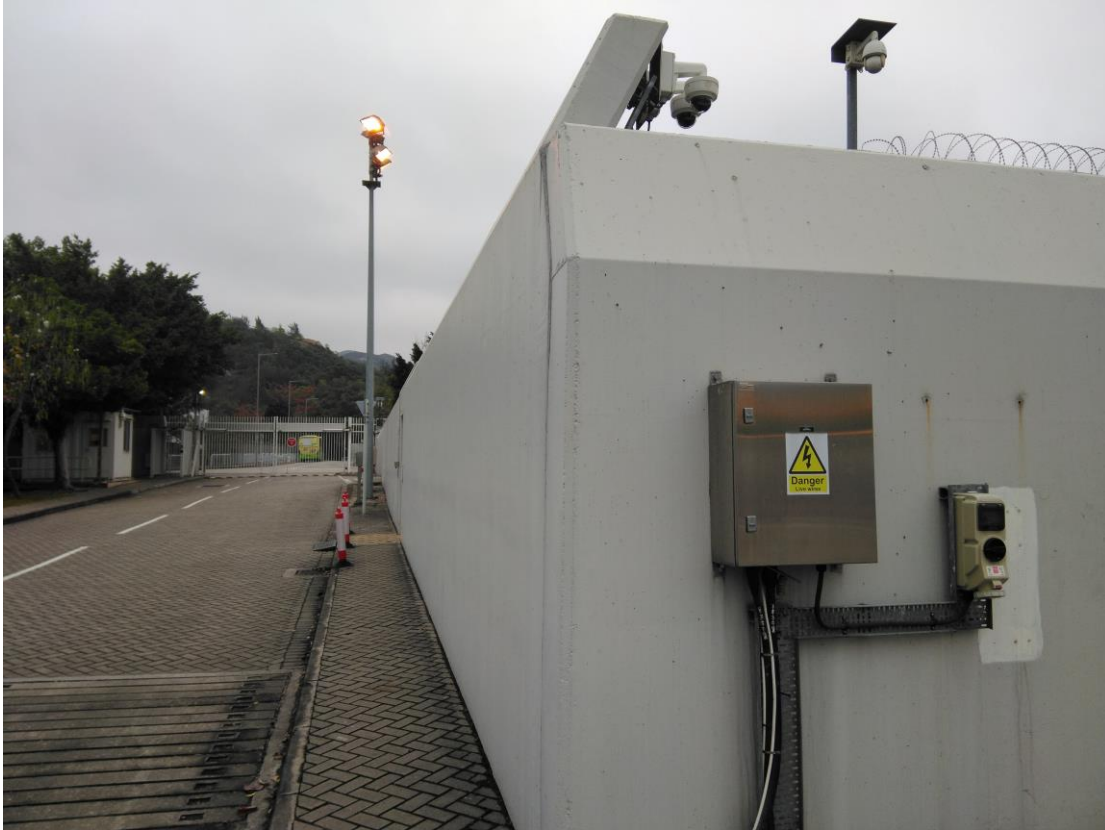
(17) This shows the thickness of the security wall provided
