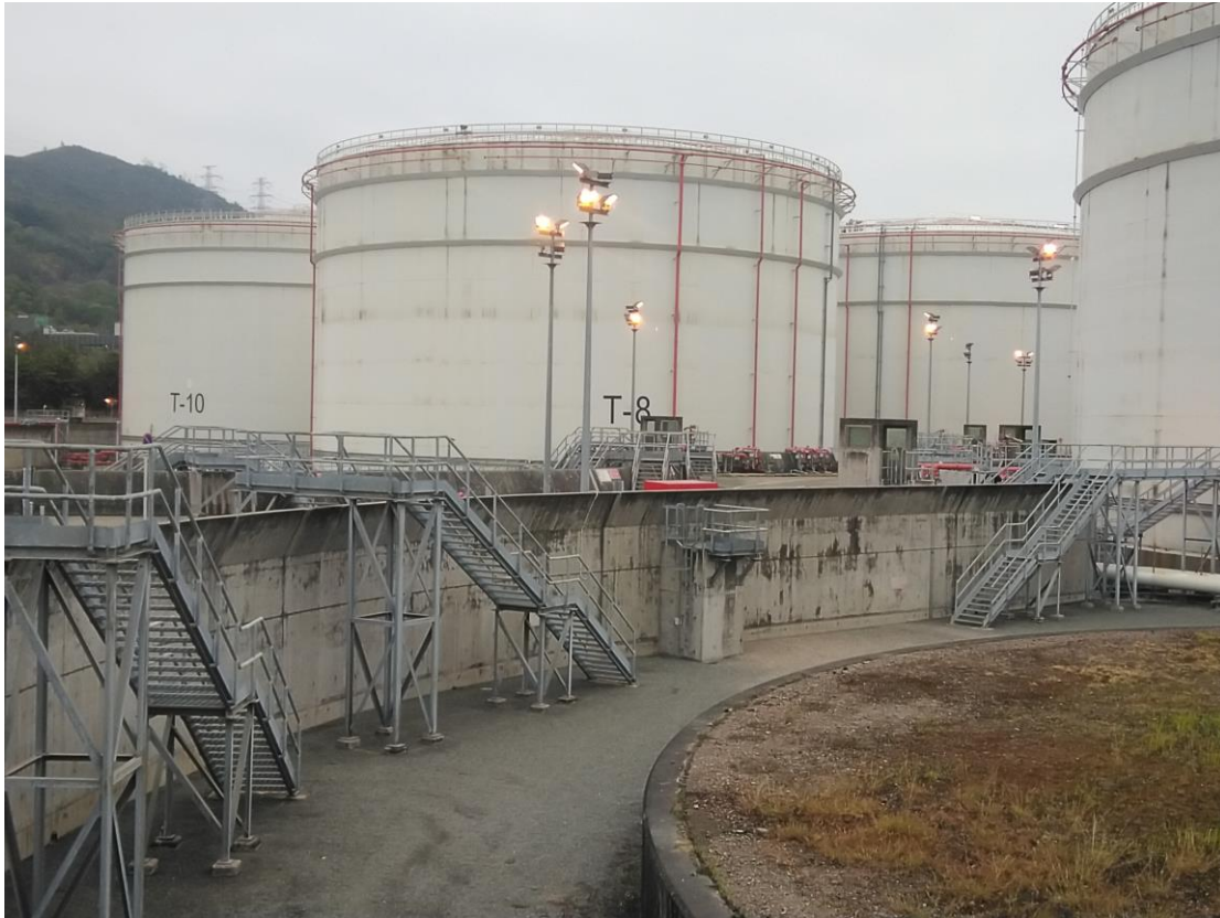
(5) Wave deflector is located at top of the bund
