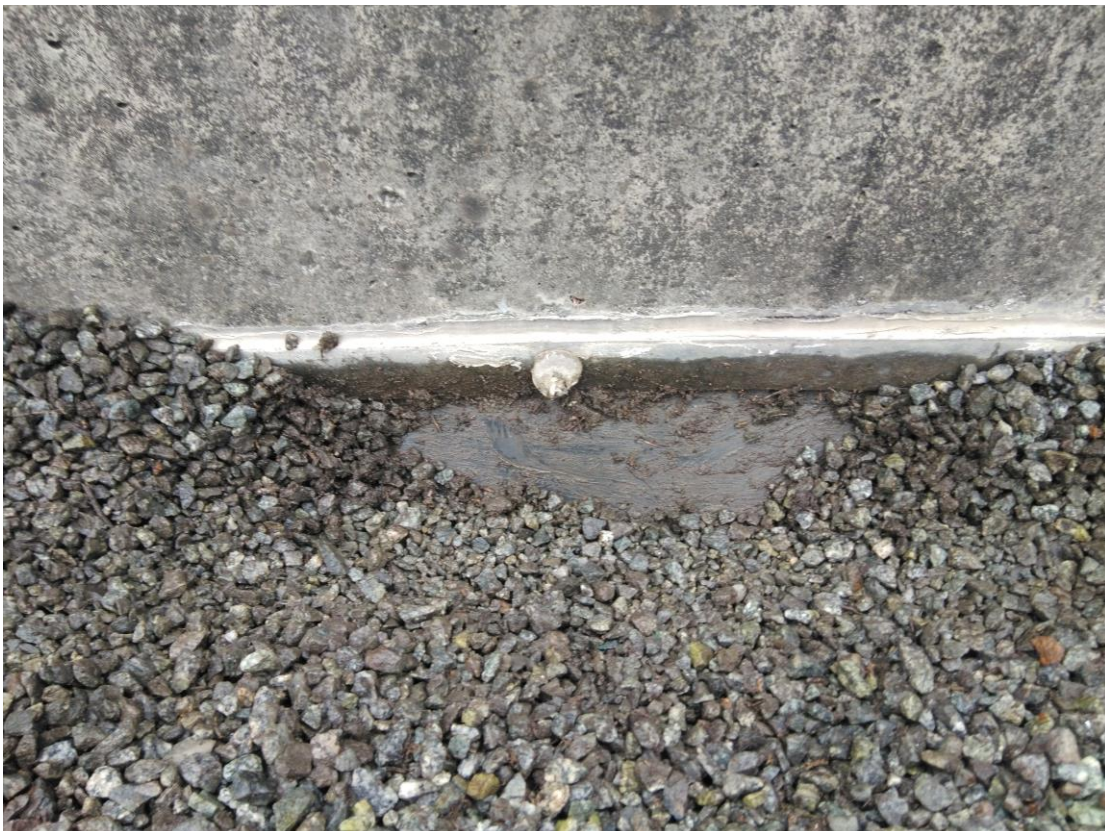
(18) Impervious lining are maintained in good condition
