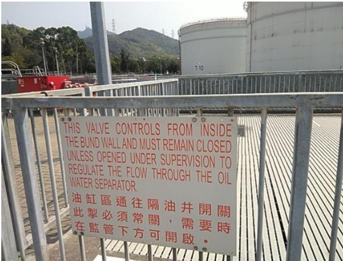
(21) Outlet valve provided for Phase 1b Interceptor with instruction sign to keep “normally closed”
