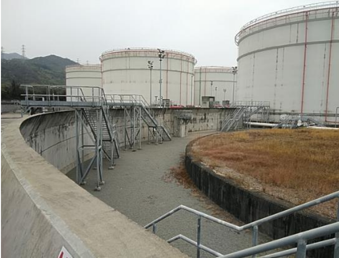
(5) Wave deflector is located at top of the bund
