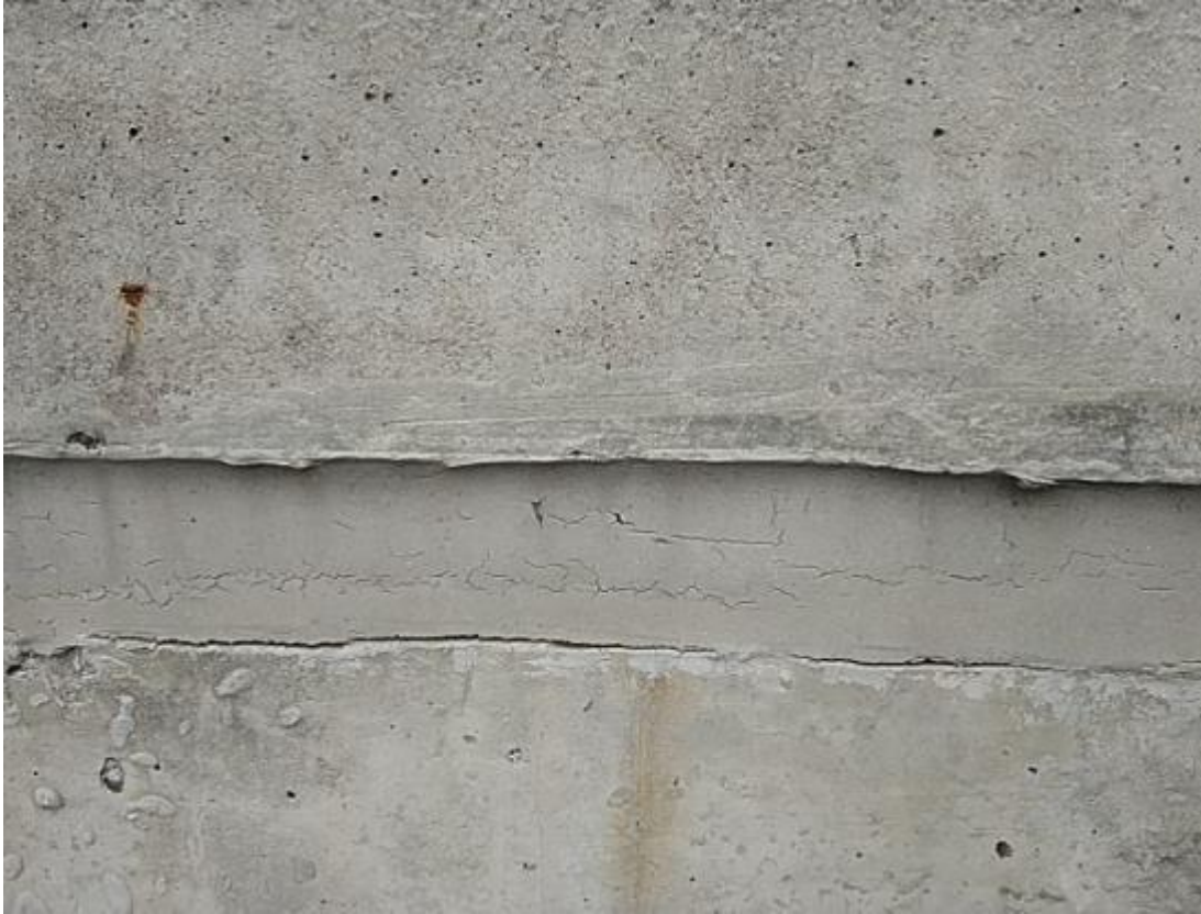
(7) Maintenance works have been performed on sealant at joints
