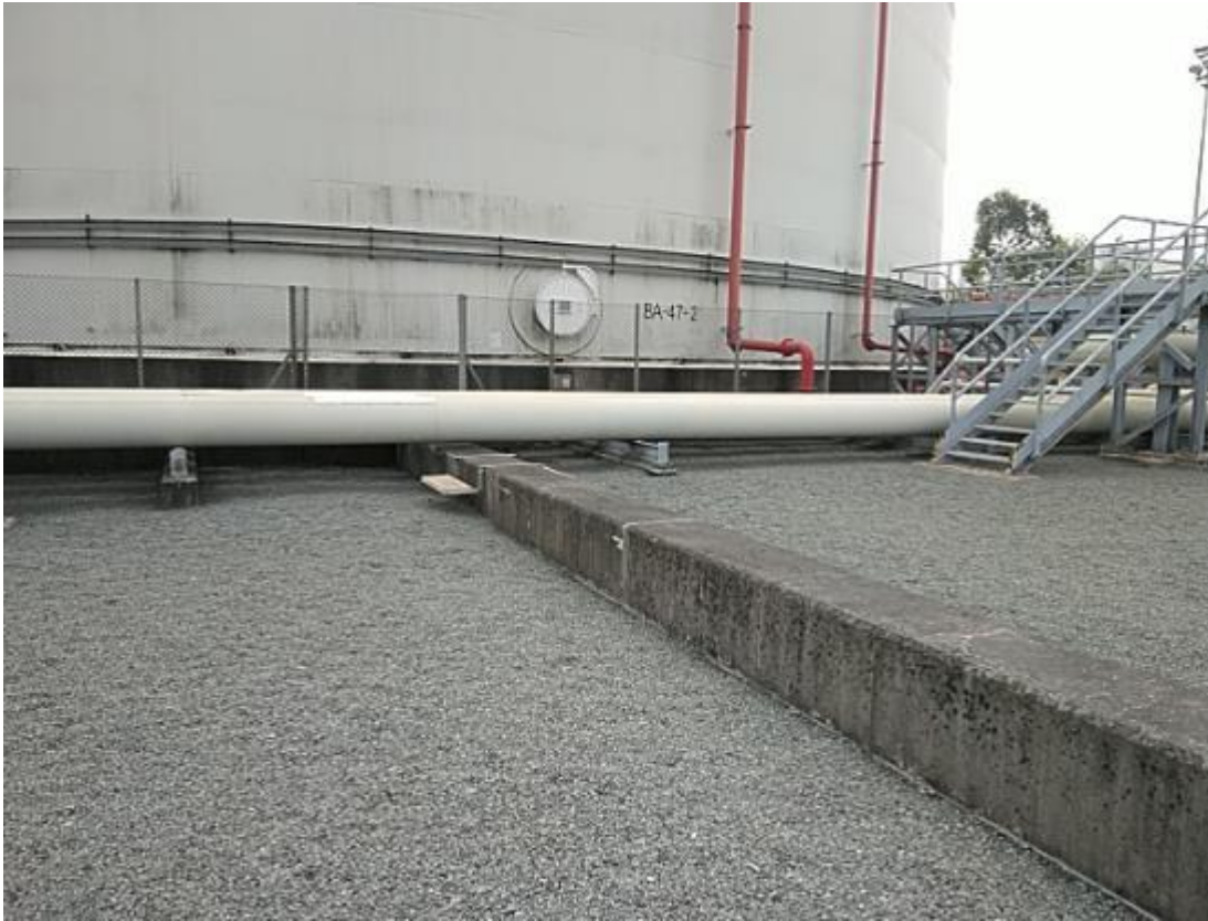
(9) Intermediate bund walls are provided in place near T-01-002
