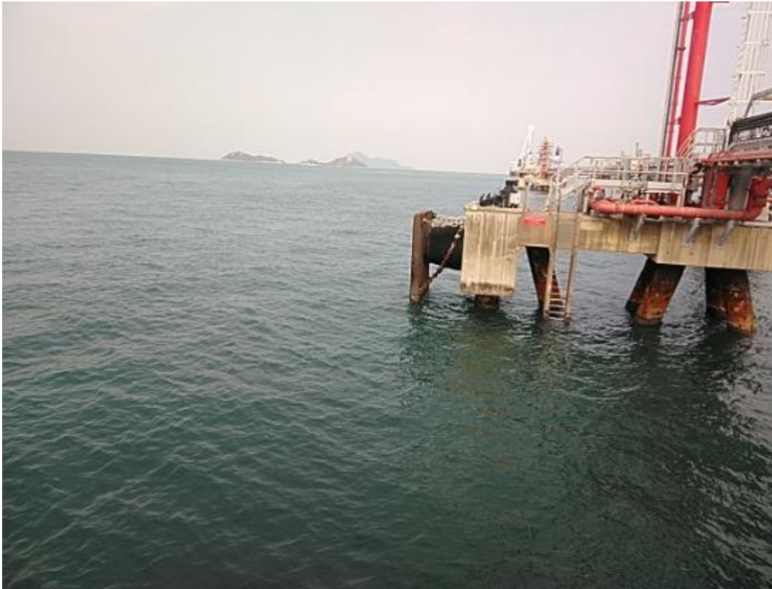
(37) Fenders are installed at sea side of the jetty
