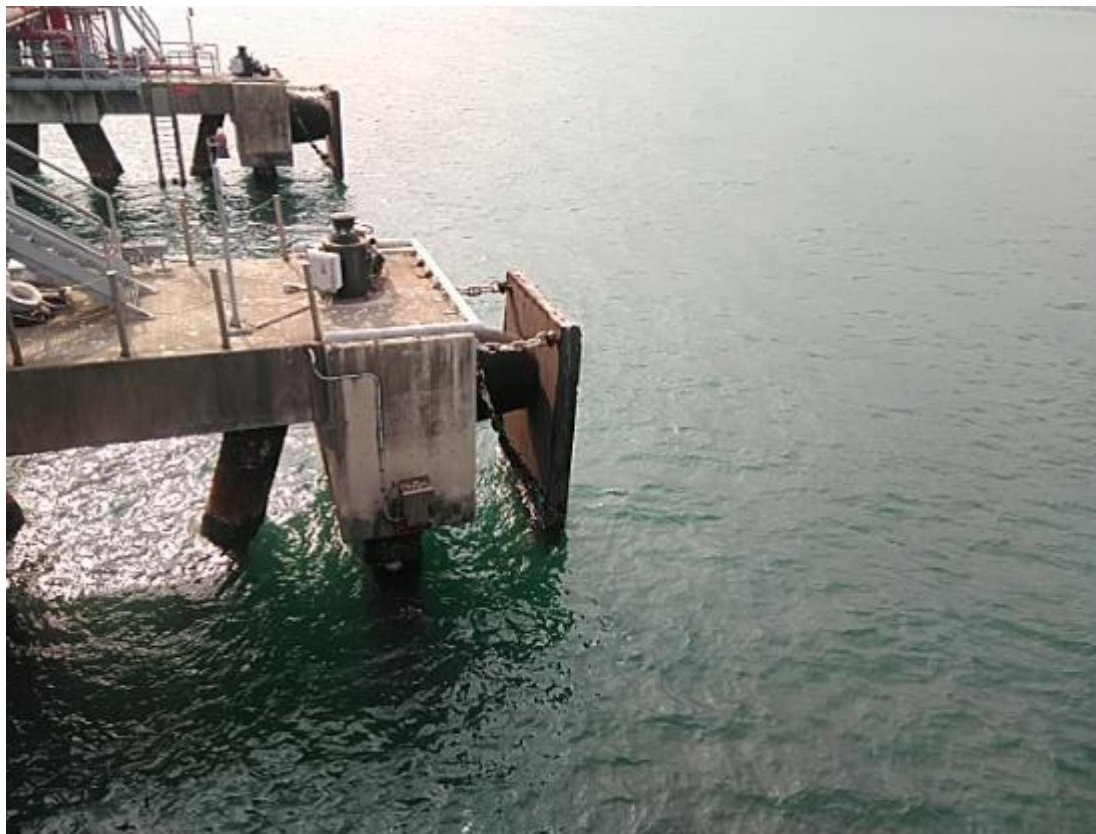
(36) Fenders are installed at sea side of the jetty
