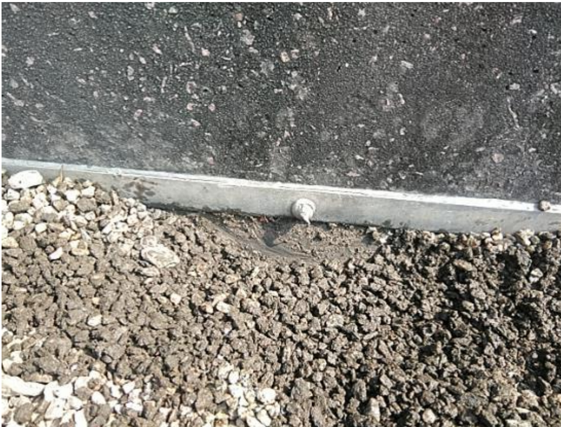
(18) Impervious lining are maintained in good condition
