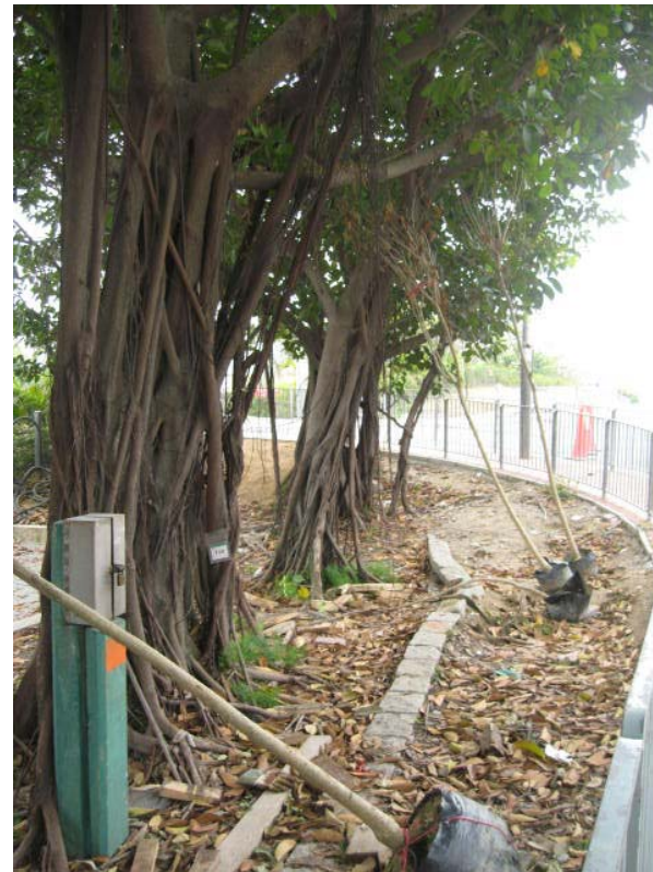
Photo 2 - Construction materials and debris stored near retained trees T68 and T69 are all cleared and retained trees are protected.
