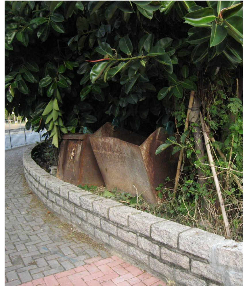
Photos 2 – Stockpile of construction material observed near Retained Tree T1
