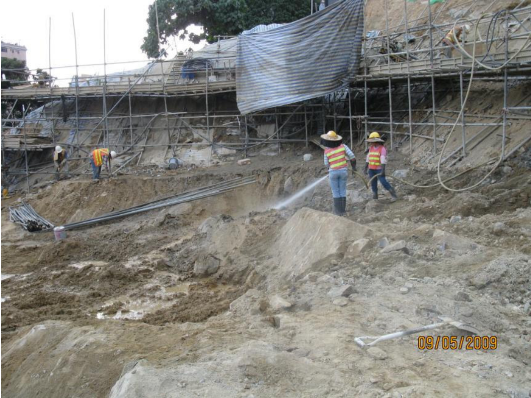
1. Water spraying for the exposed area.
