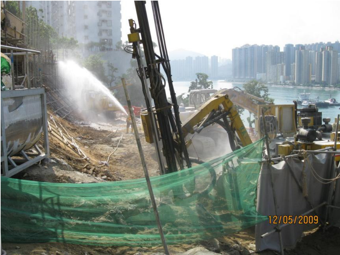
3. Water spraying during rock breaking.
