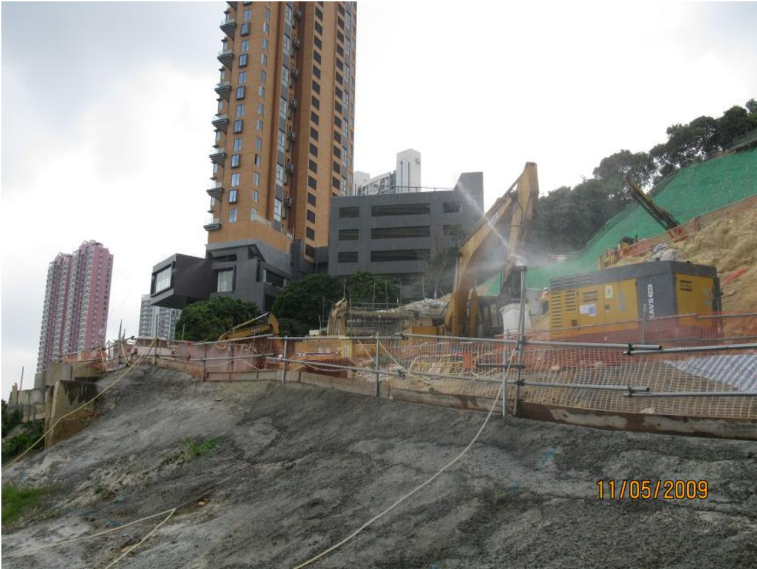
1. Water spraying for the exposed area.
