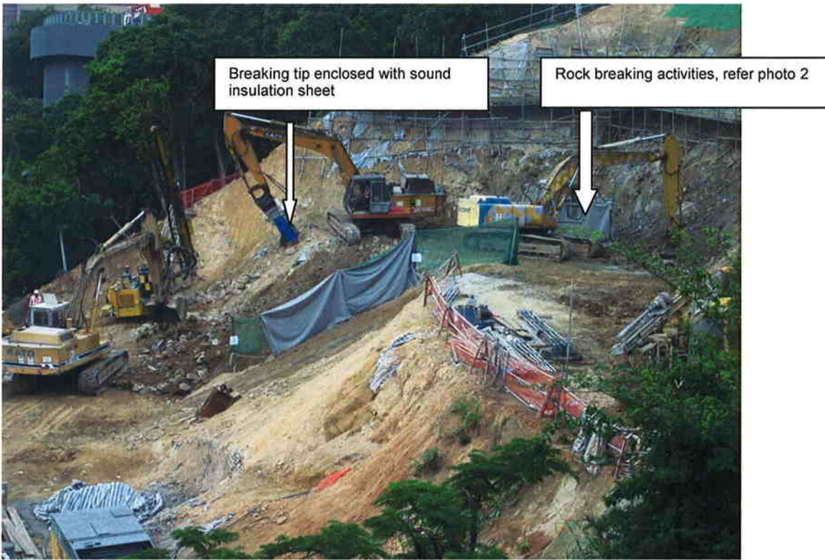
1. Sound insulation sheet erected with the green net.
