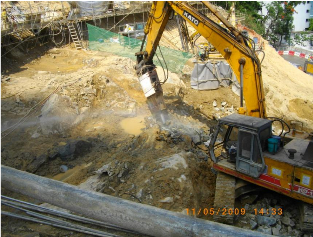
3. Water spraying during rock breaking.
