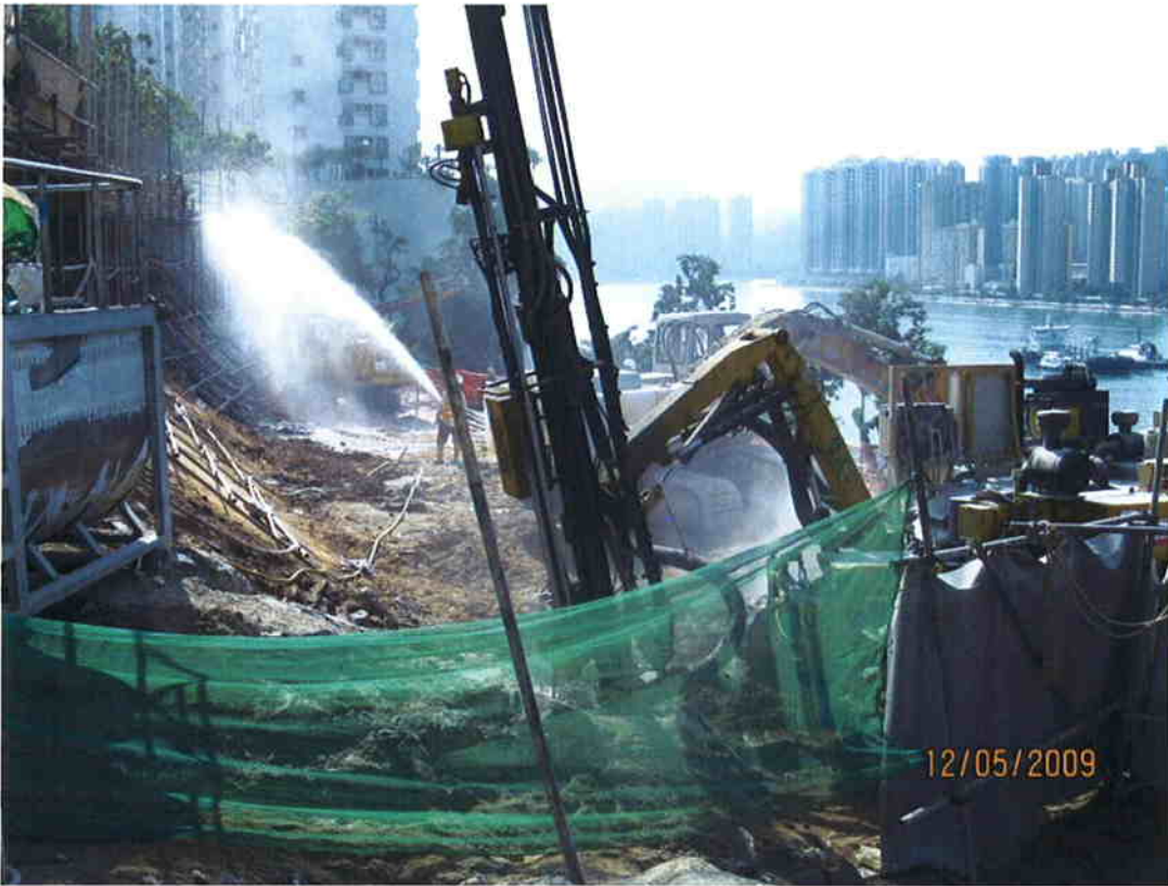
4. Water Spraying for soil nail work.
