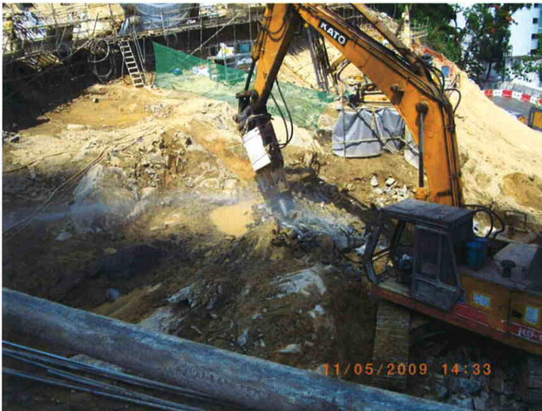
3. Water spraying during rock breaking.
