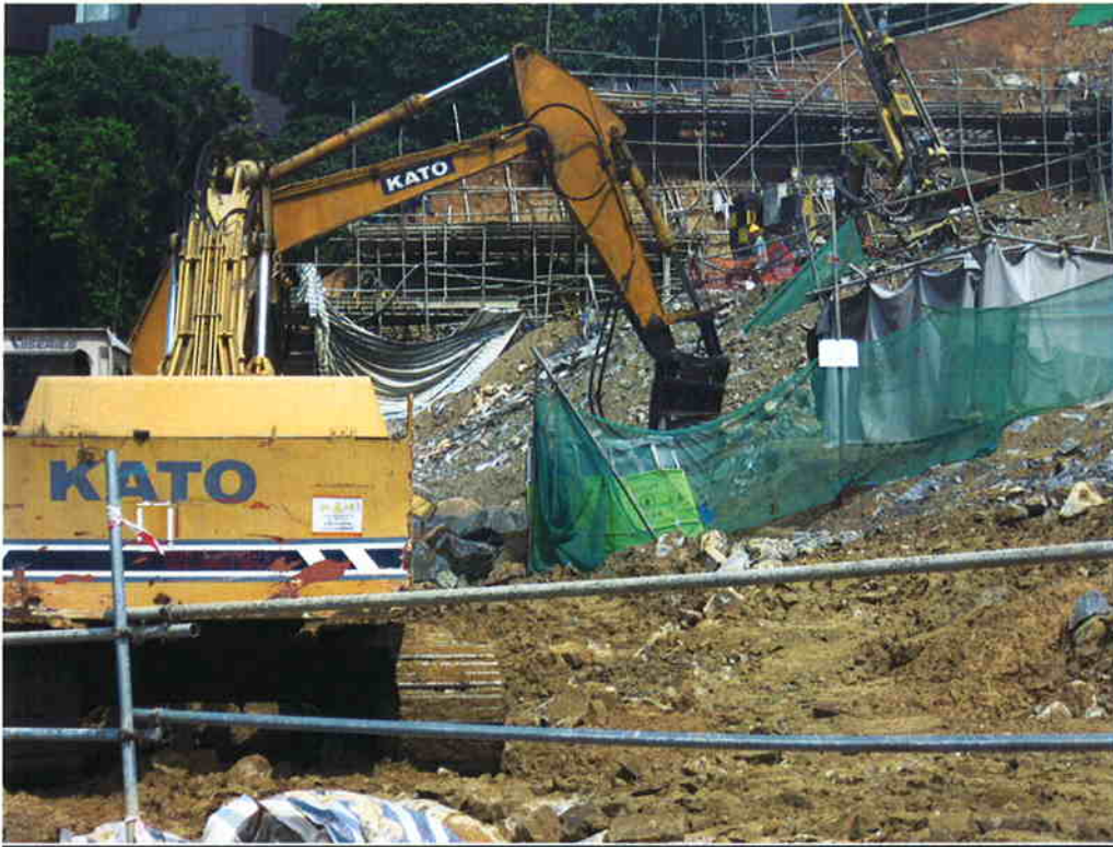
3. Noise insulation material for rock breaking.
