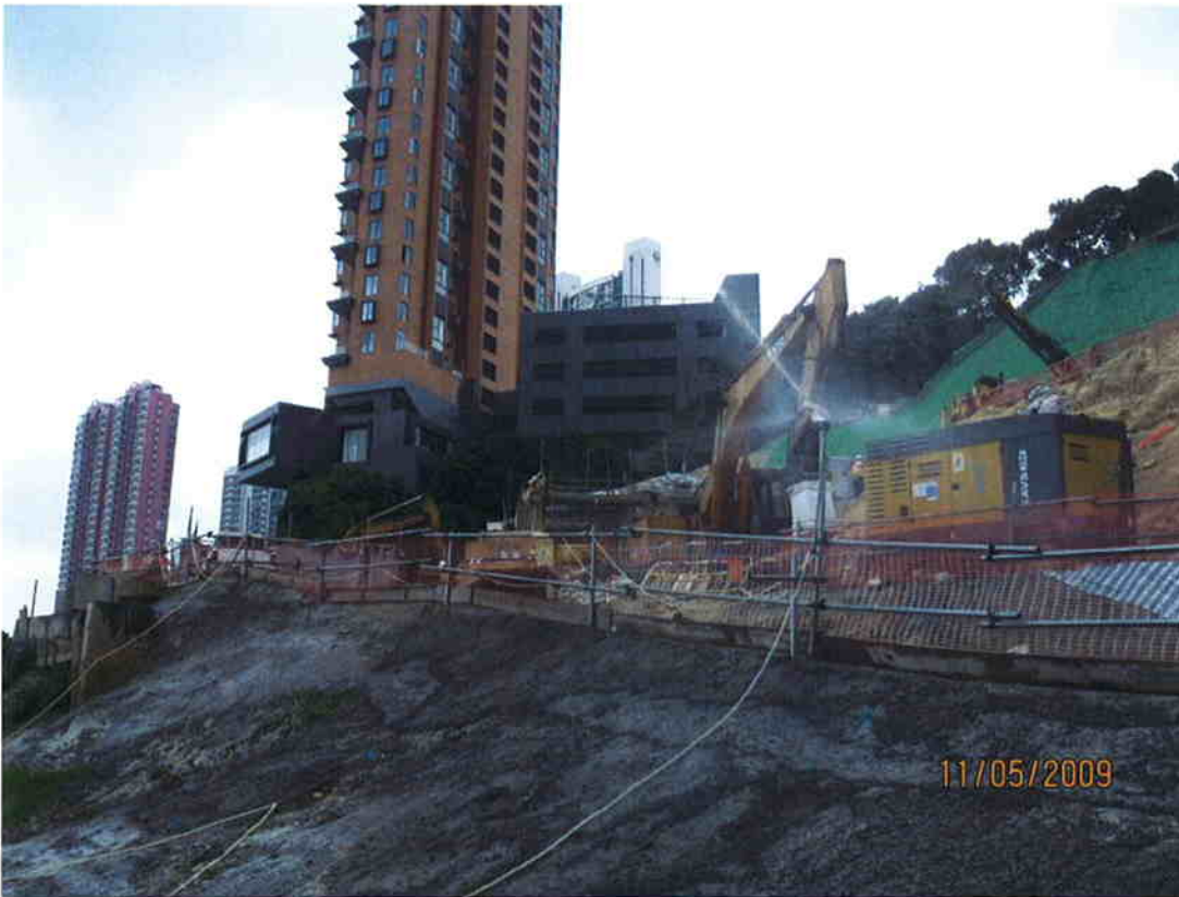
2. Automatic sprinkler spraying the haul road.
