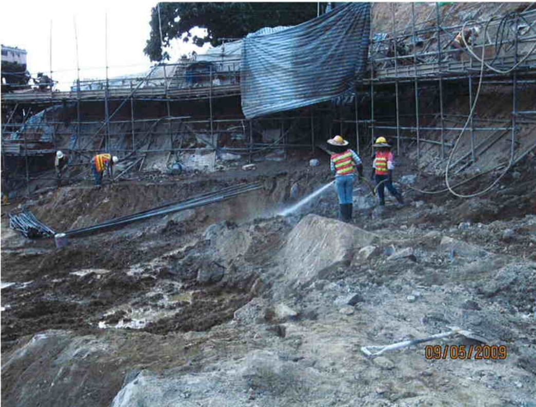
1. Water spraying for the exposed area.
