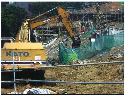
3. Noise insulation material for rock breaking.
