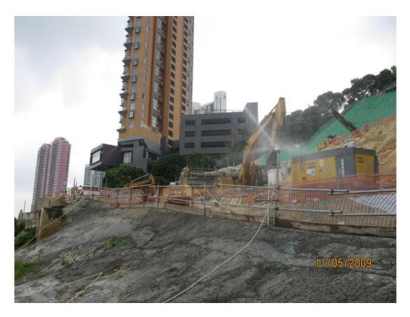
2. Automatic sprinkler spraying the haul road.
