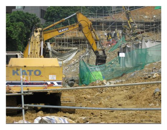
3. Noise insulation material for rock breaking.
