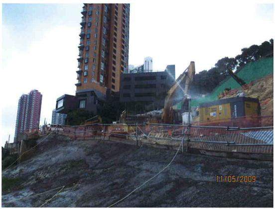
2. Automatic sprinkler spraying the haul road.
