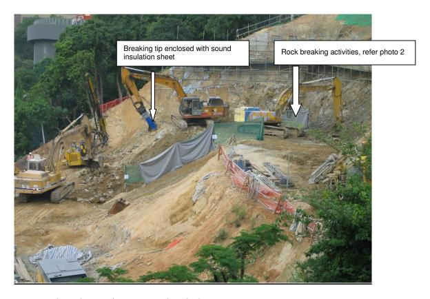
1. Sound insulation sheet erected with the green net.
