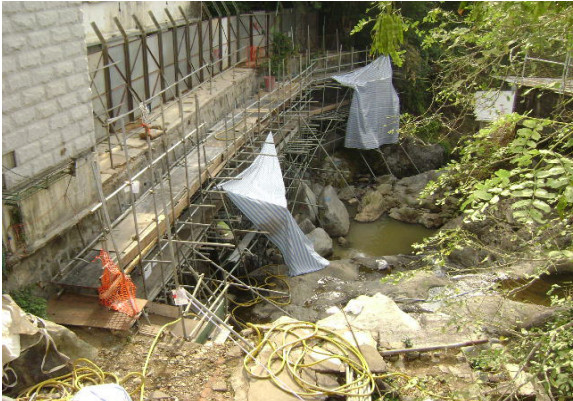
Construction activities at I-2-C.
