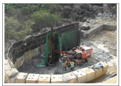
Sound insulation sheets were installed covering the working area during rock drilling in order to block the line of sight to the NSR.
