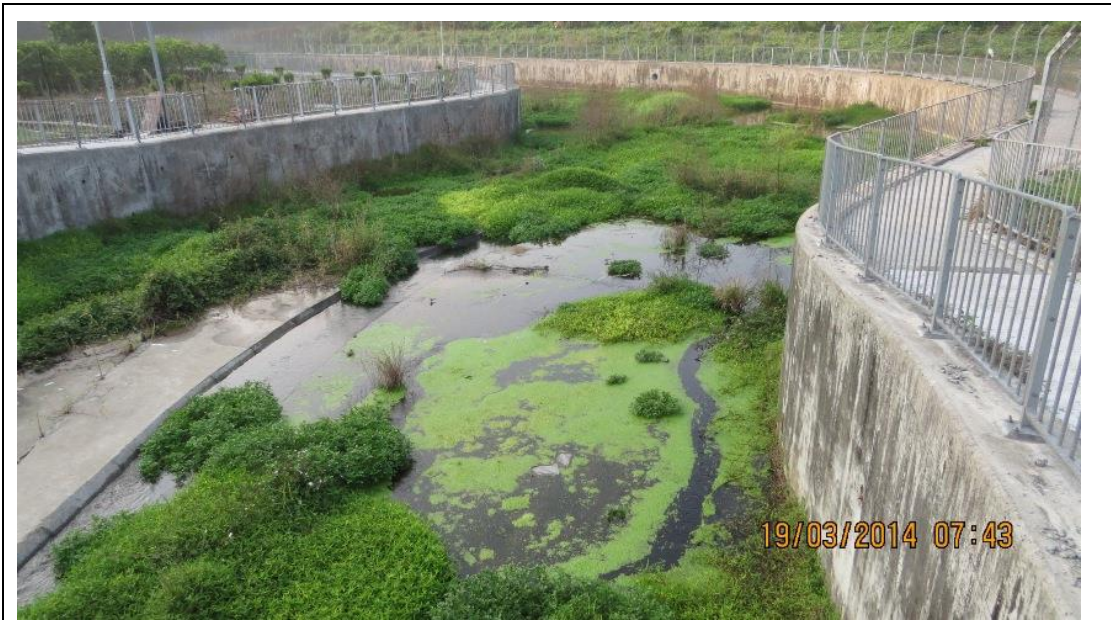
Photograph showing general view of She Shan River in March
