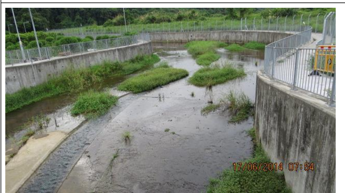
Photograph showing general view of She Shan River in June. In the wet season, most of the plants in riverbed had been washed away by flood.
