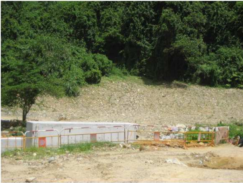
Fig.5 – Condition of Area DD21, lot232 in the complaint stated
