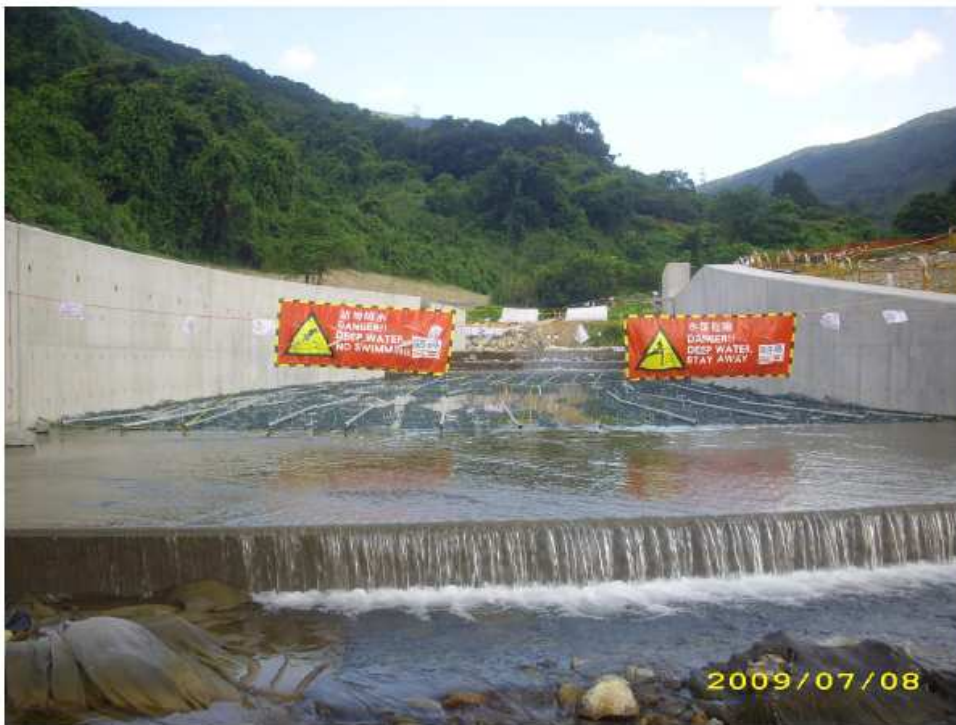
Fig.2 – River water passing through the boulder trap of UTPR was observed to be clear
