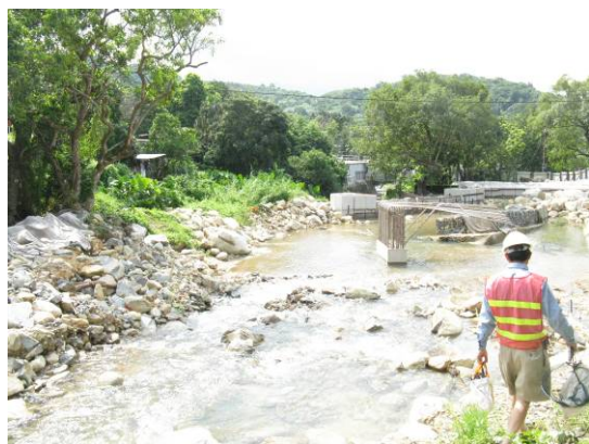
Photo 1: General view of the works area
