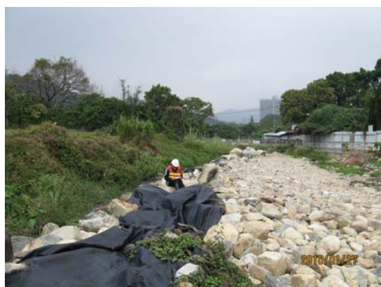
Photo 1: General view of the works area
