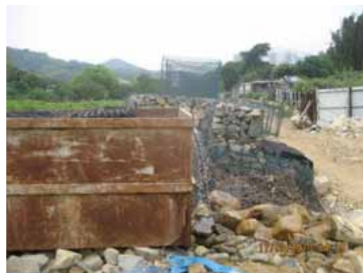
Fig.6.2 – De-silting tank was provided for site water treatment
