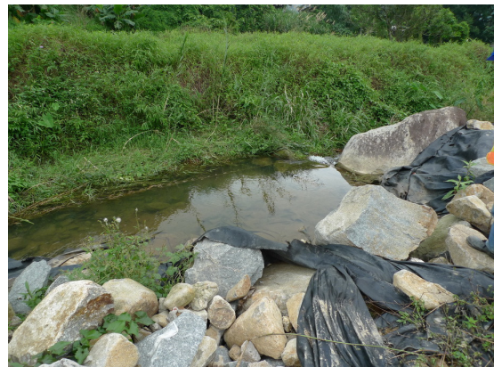
Fig.6.2 – River water at approximate ch.150
