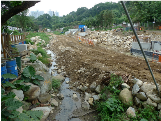
Fig.7.2 – reformed haul access at approximate ch.450
