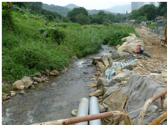
Fig.6.1 – River water at approximate ch.50
