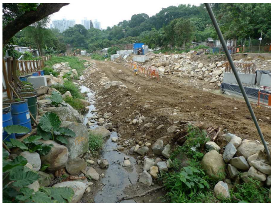
Fig.4.2 – Reformed haul access at approximate ch.450
