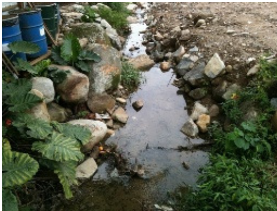
Fig.3.3 – River channel near site ch.400
