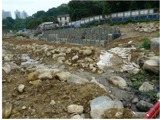
Fig.7.1 – reformed haul access at approximate ch.300
