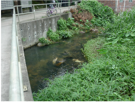
Fig.6.3 – River water at downstream area
