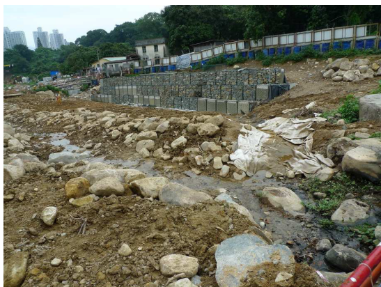
Fig.4.1 – Reformed haul access at approximate ch.300
