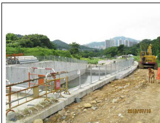
Photo 1: General view of the works area
