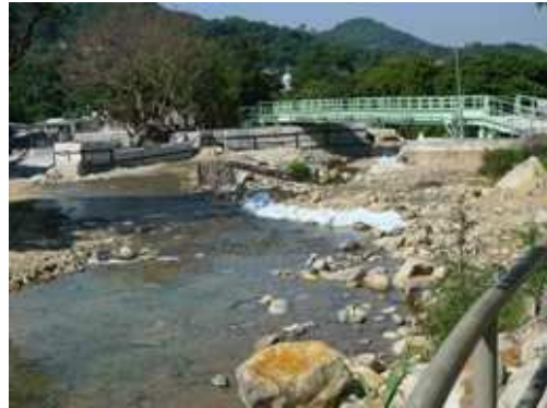
Fig.4.4 – Provision of geo-textile coverings to riverbanks at ch.250
