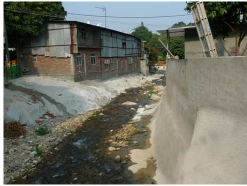
Fig.3.4 – Water quality at down stream area (taken on 19/11)
