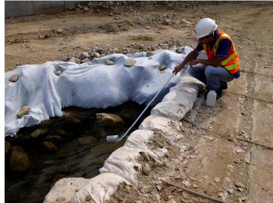
Fig.4.2 – Sampling and monitoring at approx. ch650 on 16/11 (Photo provided by Contractor)
