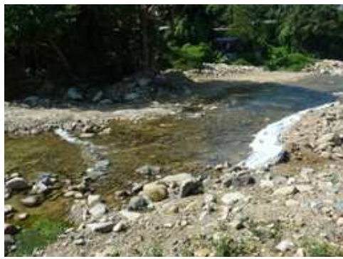
Fig.4.1 – Provision of sandbags barriers at approximate ch.250(1) Fig.4.2 –Provision of sandbags barriers at approximate ch.250(2)
