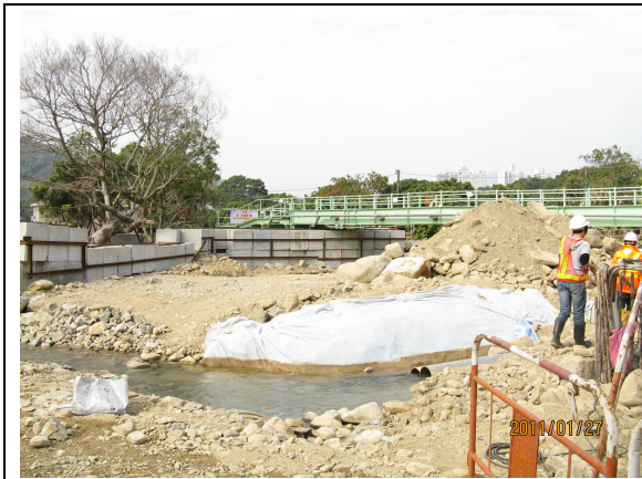
Photo 1: General view of the works area
