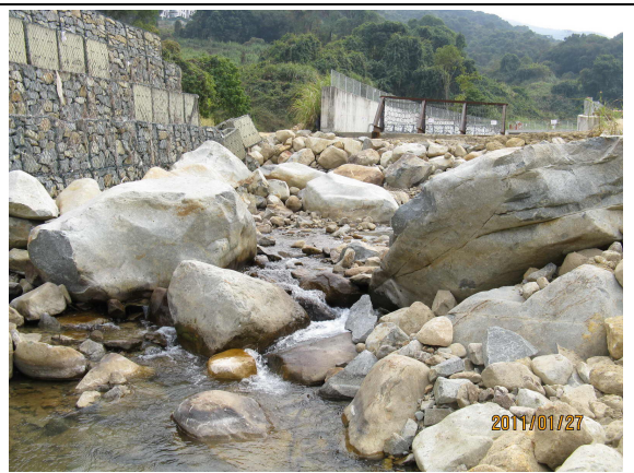
Photo 2: General view of the works area
