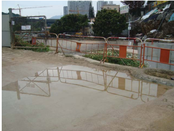
Fig.6.1 – Wheel Washing Bay is cleaned before and after works everyday
