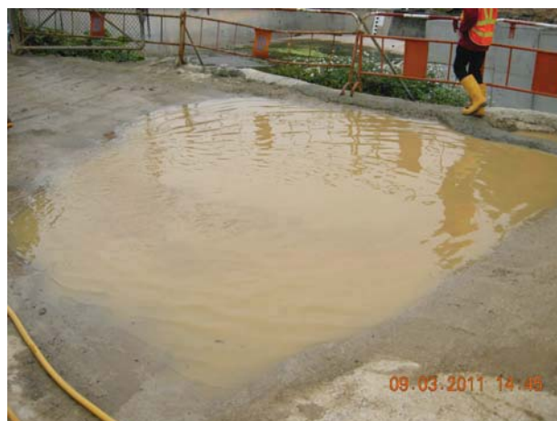
Fig.4 – Condition of Wheel Washing Bay at site entrance located at ch.600
