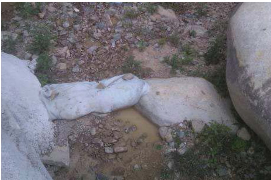
Fig.3.1 – Sandbags barriers was formed to form enclosed environment for construction activities carrying out at ch.400
