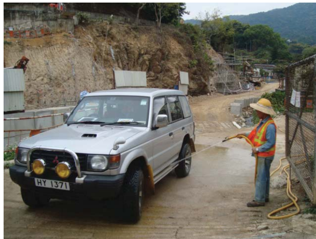
Fig.6.2 – Briefing has been given to staff to remind importance of vehicle washing before leaving site
