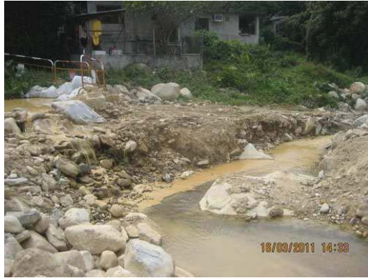
Fig.2.1 – Effluent discharge from ch.200 on 16/03/11
