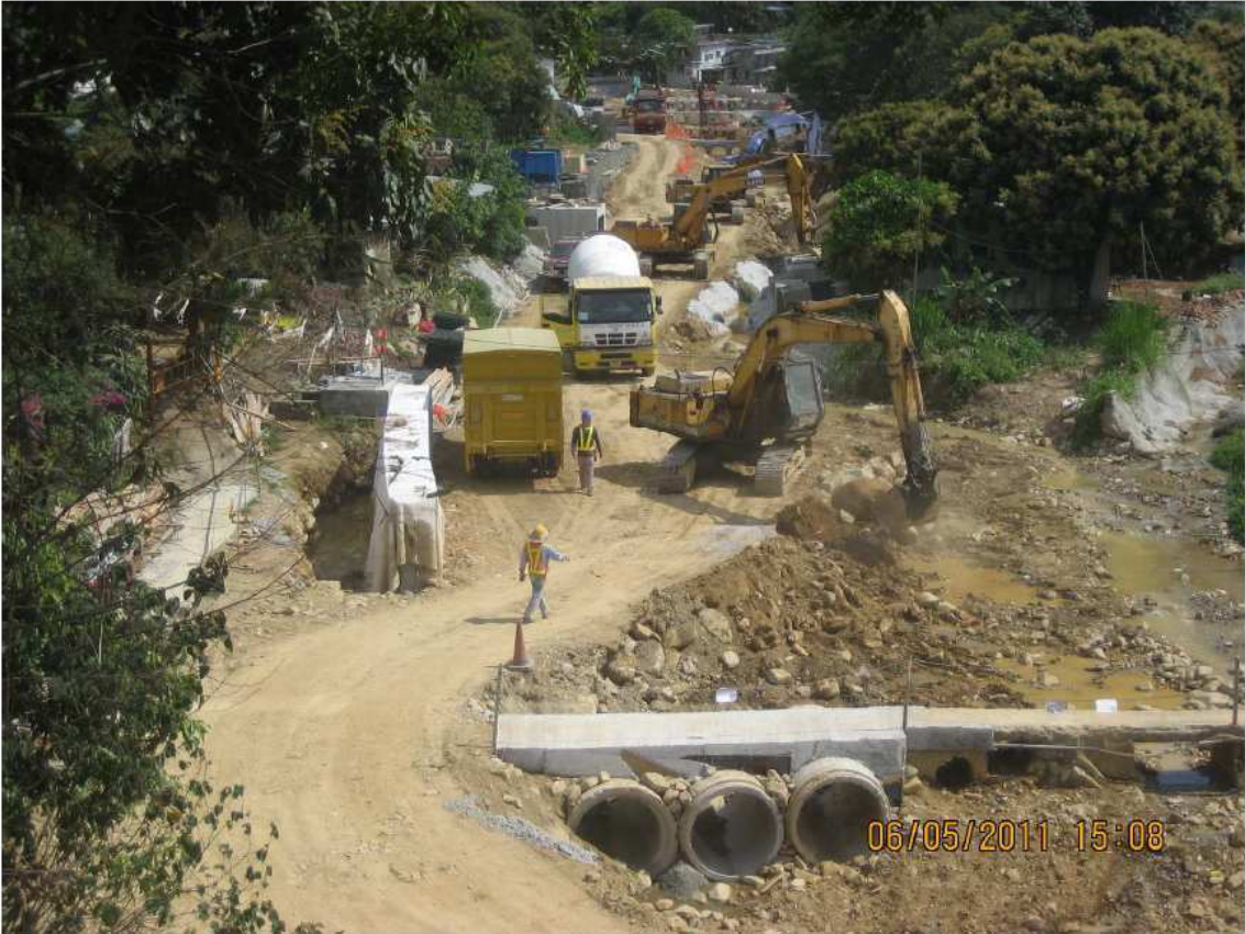
Fig.1 – Excavators were operating at the same time
