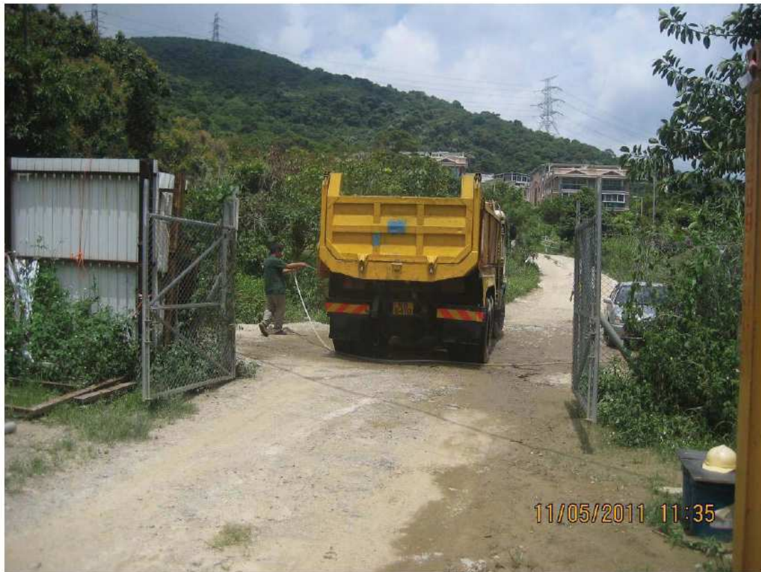
Fig.5.1 – Water condition in the wheel washing bay at site entrance at ch.600 was muddy.
