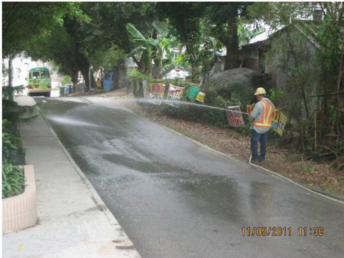
Fig.4.1 – Regular water spraying was provided for the public area at Tat Wan Road.
