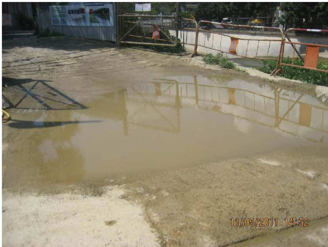
Fig.5.1 – Water condition in the wheel washing bay at site entrance at ch.600 was muddy.
