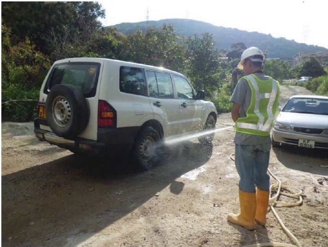
Fig.4.4 – High jet water sprayer was used for wheel washing at site entrance at Access Road D.
