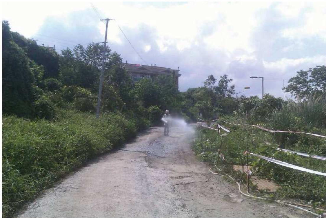
Fig.4.2 – Regular water spraying was provided for Access Road D.
