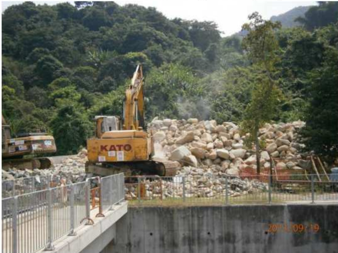
Fig.5.2 – Dust emission was still observed during the rock breaking activity.
