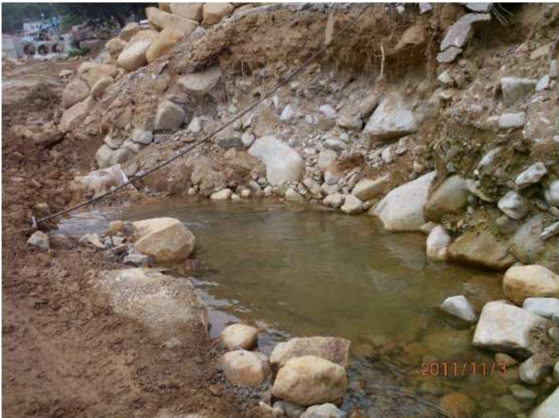
Fig.6.1 – Earth bunds was provided to avoid leakage of muddy runoff entering into the river (photo provided by Contractor).
