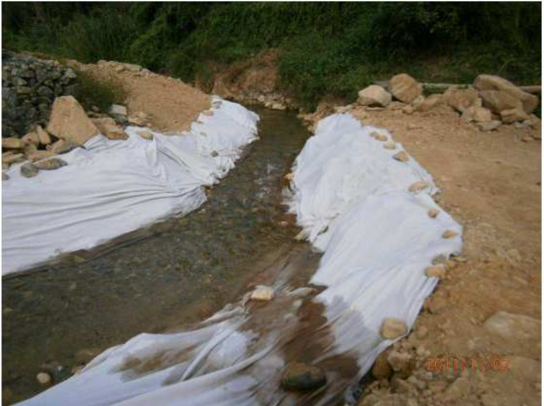
Fig.5.1 – Geo-textile covering was provided to prevent soil erosion.
