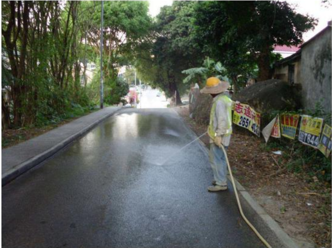
Fig.4.2 – Regular water spraying was provided for Access Road D.
