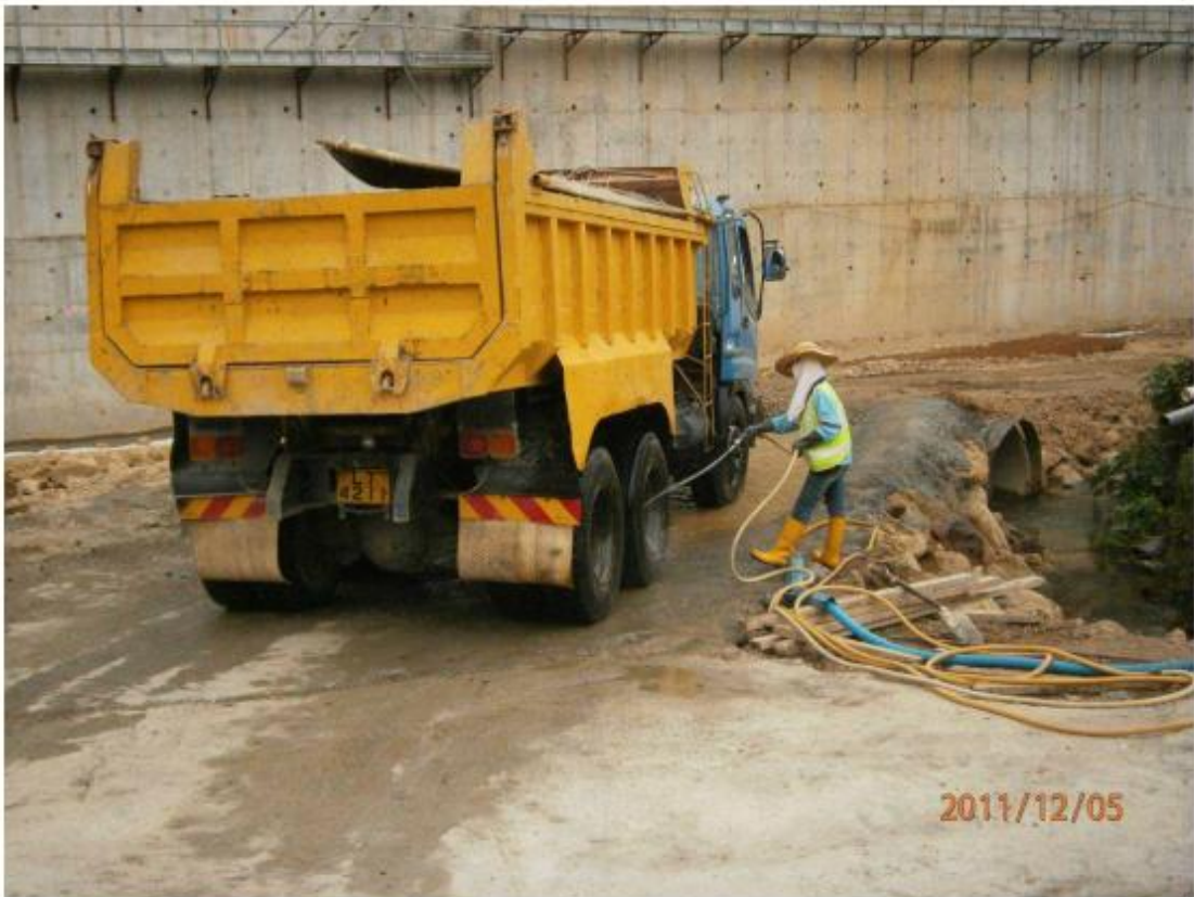
Fig.5.1 –High jet water sprayer and wheel washing bay was used for wheel washing at site entrance at ch.600.
