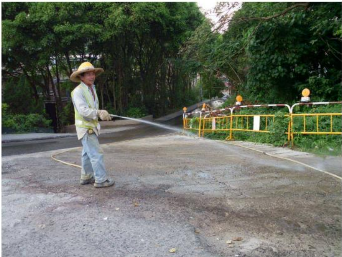
Fig.4.2 – Regular water spraying was provided for Access Road D.
