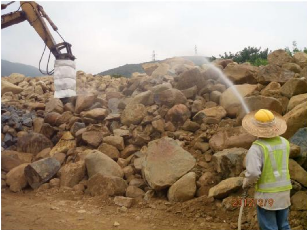
Fig. 2 – Water spraying was provided by frontline staff for dust suppression.
