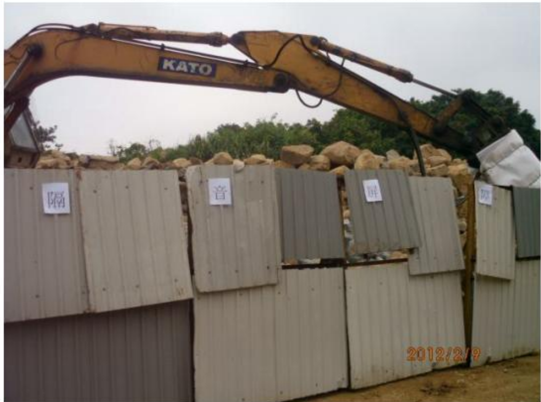
Fig.4 –Temporary noise barrier was erected for noise screening.
