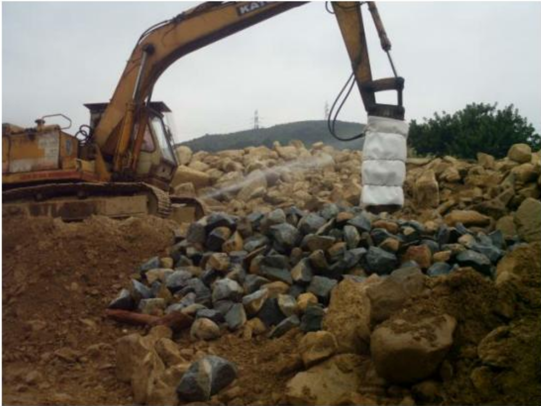
Fig.4 –Temporary noise barrier was erected for noise screening.
