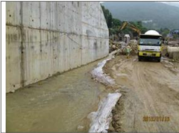
Photo 1: General view of the works area
