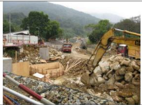
Photo 2: General view of the works area
