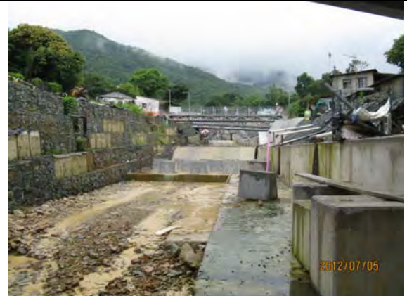
Photo 2: General view of the works area
