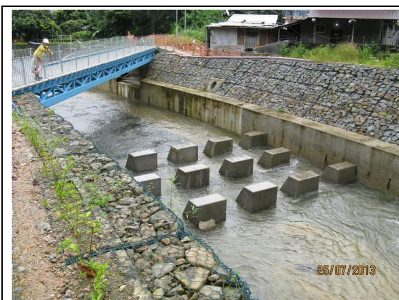
Photo 1: General view of the works area
