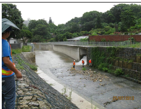
Photo 2: General view of the works area
